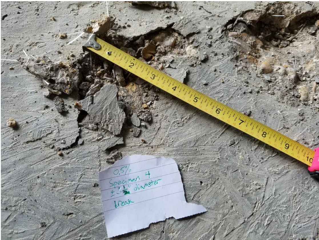
Figure 40: 0.5% Fiber - Specimen 4 Failure
