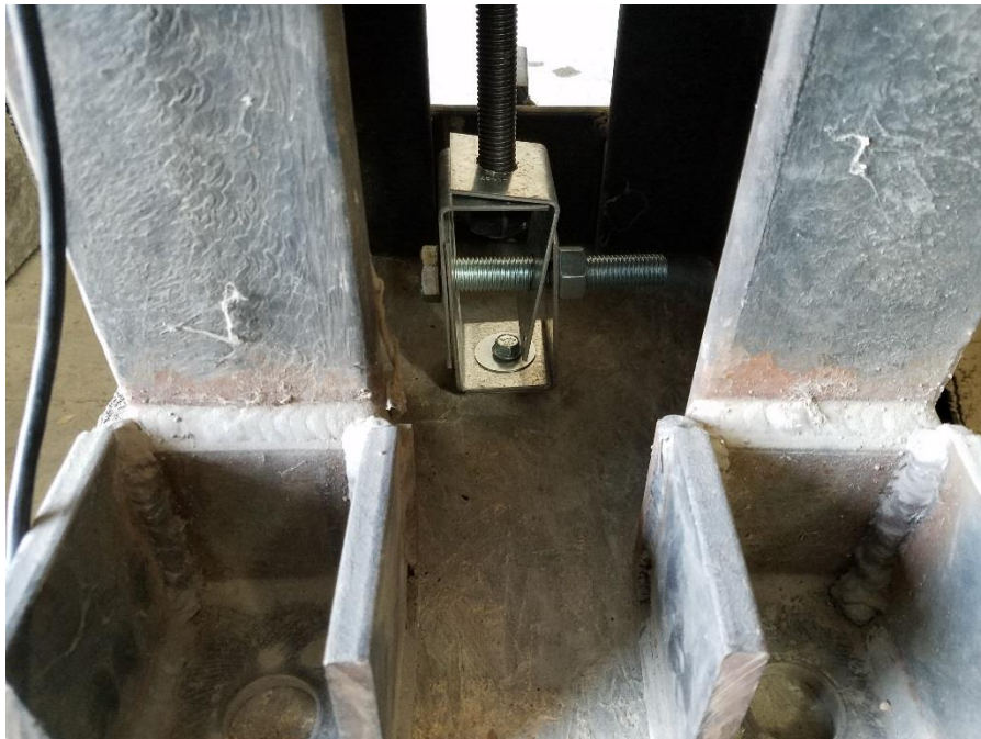
Figure 18: Anchor pullout test closeup
