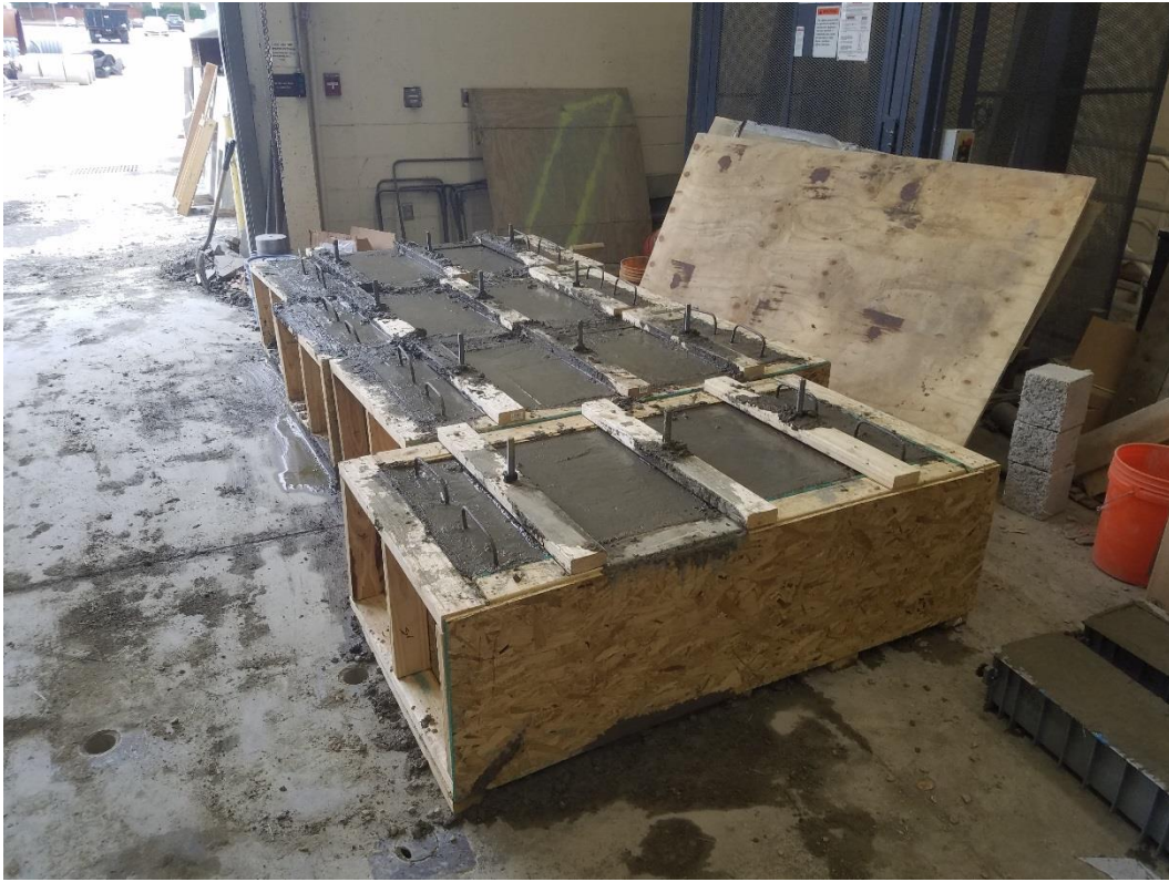
Figure 8: Large concrete beams after pour
