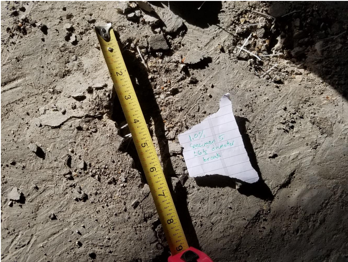
Figure 46: 1.0% Fiber - Specimen 5 Failure
