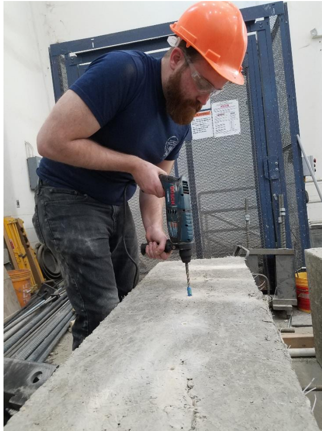
Figure 14: Holes are being drilled for the installation of the screw anchors
