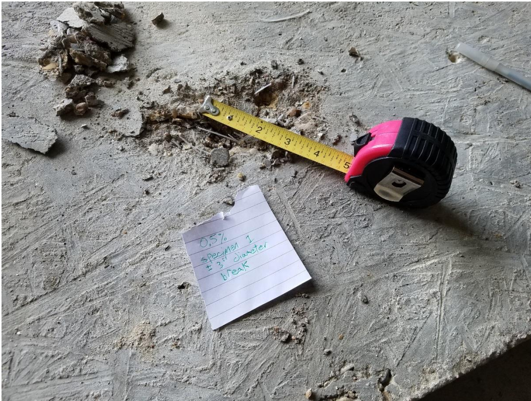
Figure 37: 0.5% Fiber - Specimen 1 Failure
