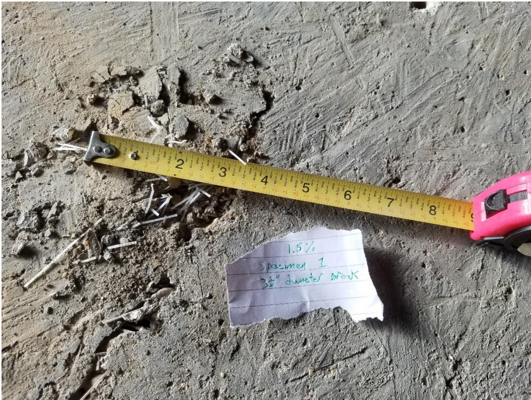
Figure 47: 1.5% Fiber - Specimen 1 Failure
