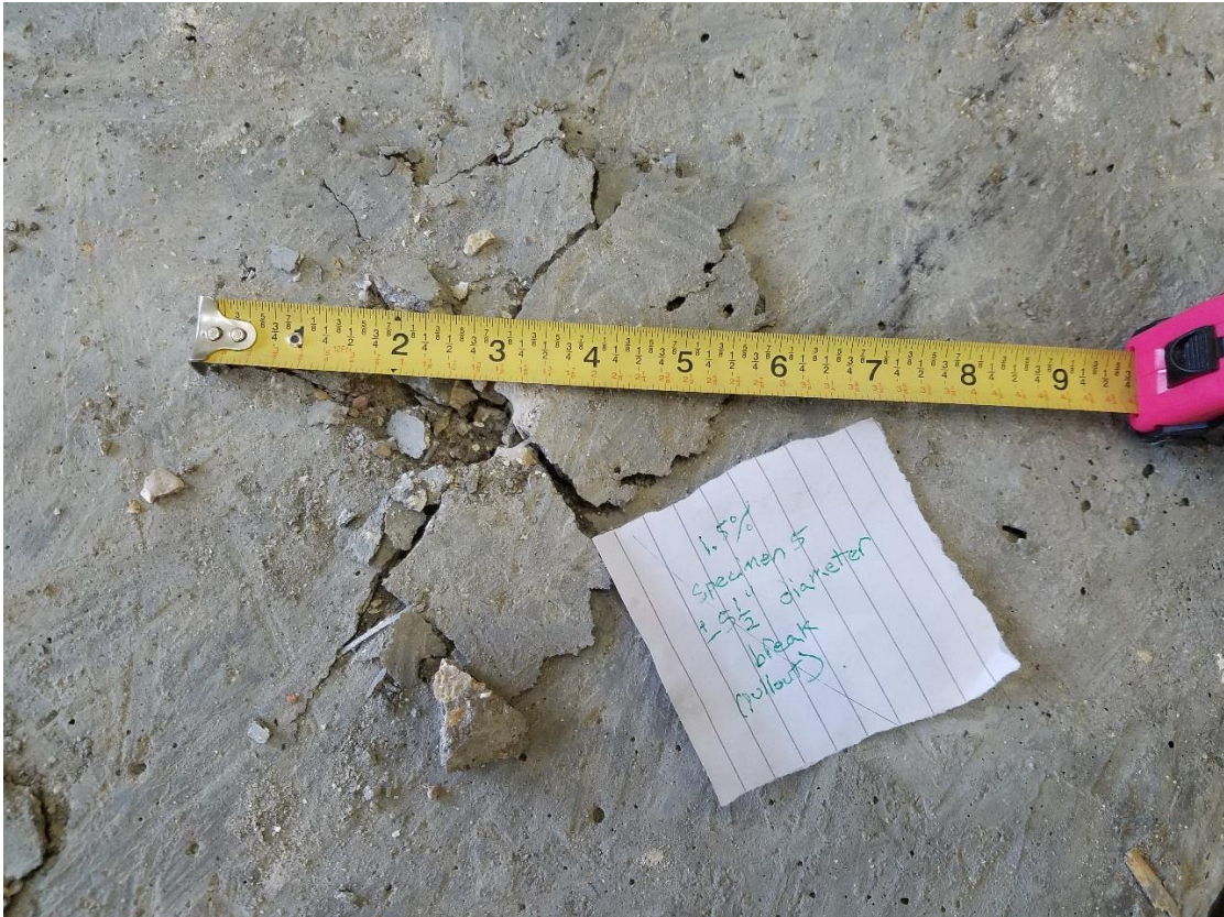
Figure 51: 1.5% Fiber - Specimen 5 Failure
