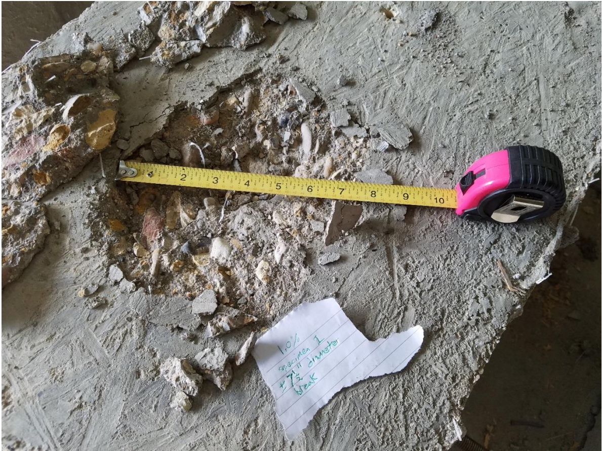
Figure 42: 1.0% Fiber - Specimen 1 Failure
