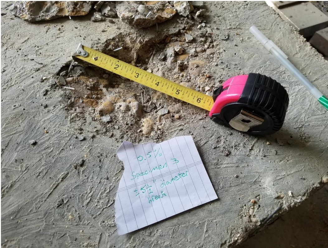
Figure 39: 0.5% Fiber - Specimen 3 Failure
