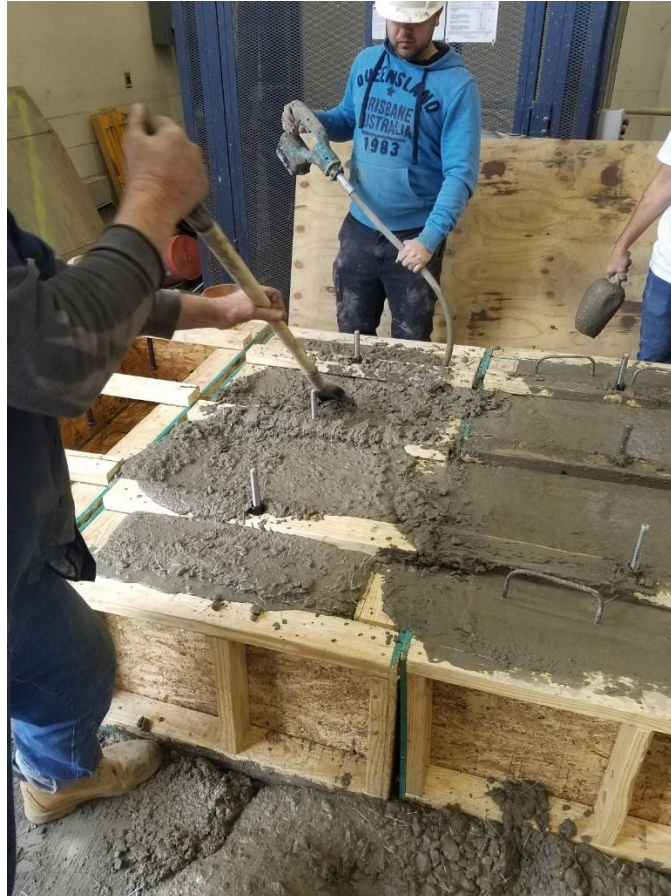
Figure 5: Concrete beam being vibrated and consolidated
