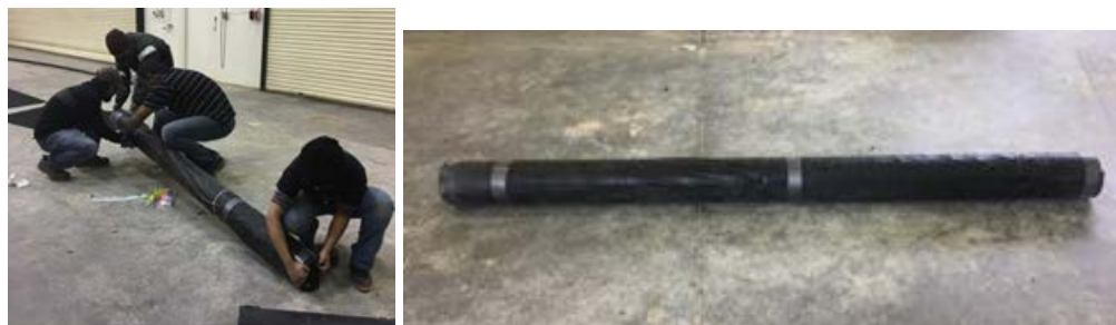
Figure 5-29 Geotextile wrapping around gas well
