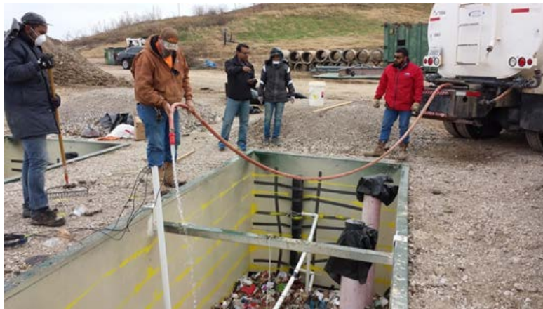
Figure 5-19 Water addition during waste filling
