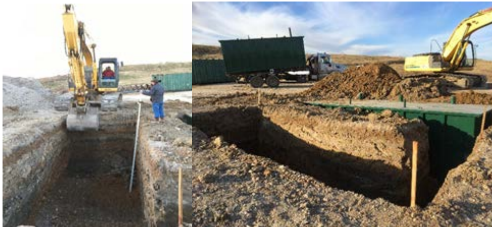
Figure 5-5 Completed excavation area for cell placement
