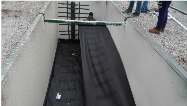
Figure 5-14 Placement of geotextile drainage layer
