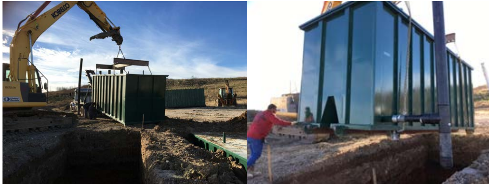
Figure 5-6 Cell placement in the excavated area
