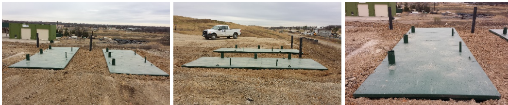
Figure 5-10 Installed box after extensive earth work and backfilling
