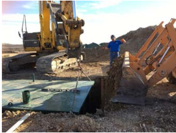
Figure 5-9 Backfilling around cell
