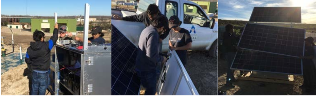
Figure 5-36 Solar panel installation
