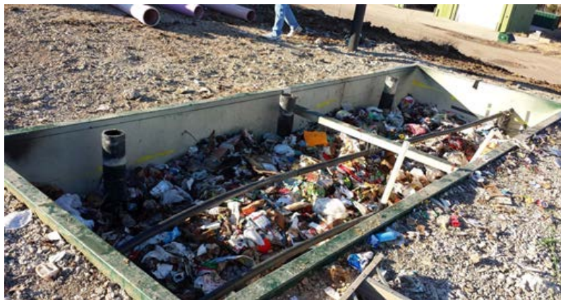
Figure 5-20 Recirculation pipe placement after waste filling
