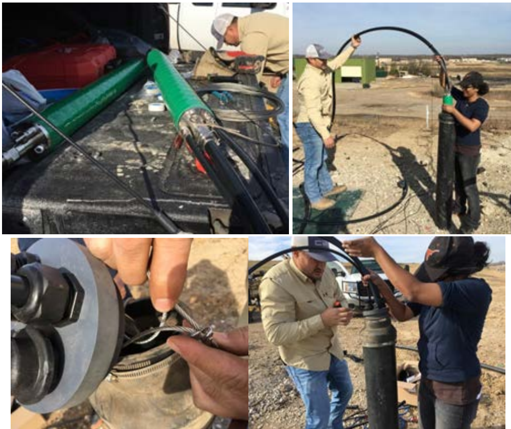
Figure 5-32 Pneumatic pump installation in sump pipe
