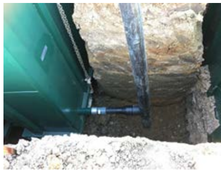
Figure 5-7 Additional area excavated for placement of leachate collection sump
