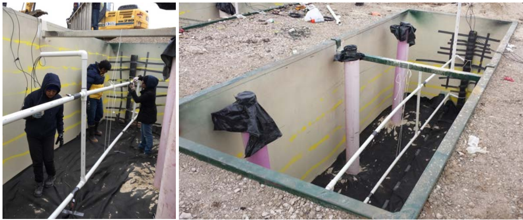
Figure 5-17 Placement of PVC pipe frame holding the sensors in the cells
