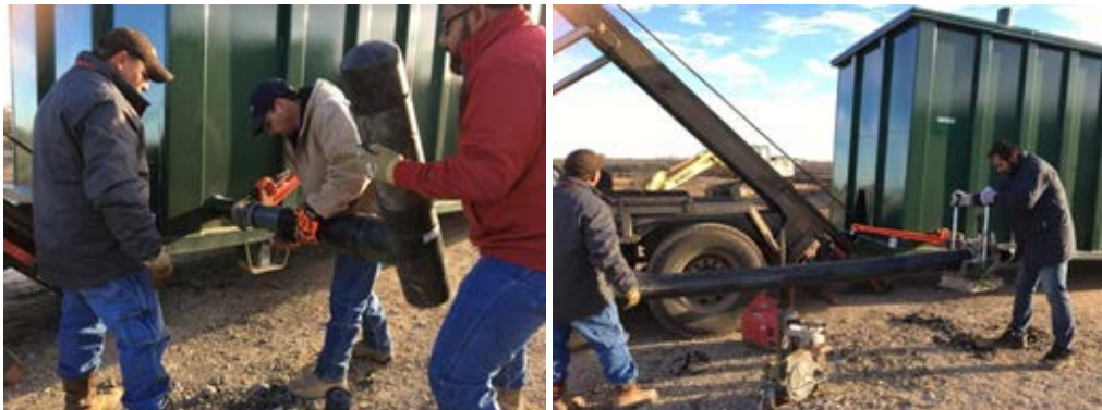
Figure 5-23 Leachate collection sump connection with drainage port of the cell
