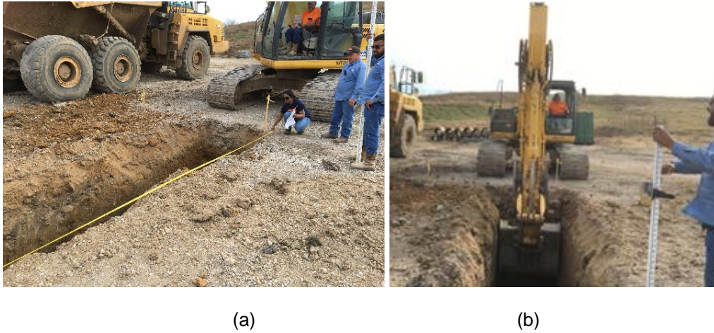
Figure 5-4 (a) Measurement of excavated area; (b) Excavation of cell
