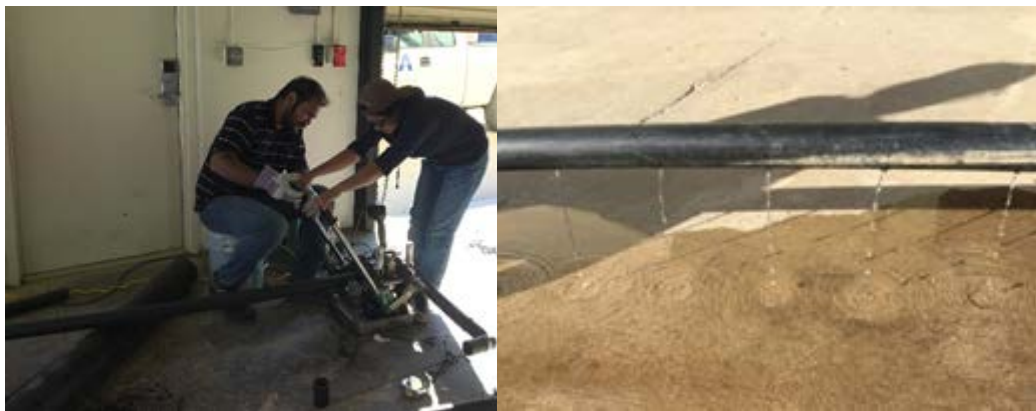
Figure 5-25 Leachate recirculation pipe perforation at 120 degrees
