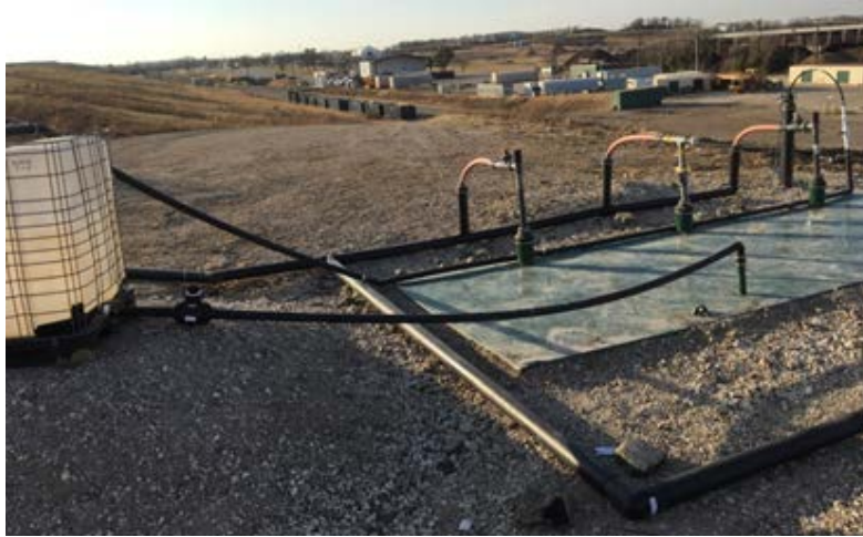
Figure 5-27 Leachate collection and recirculation system
