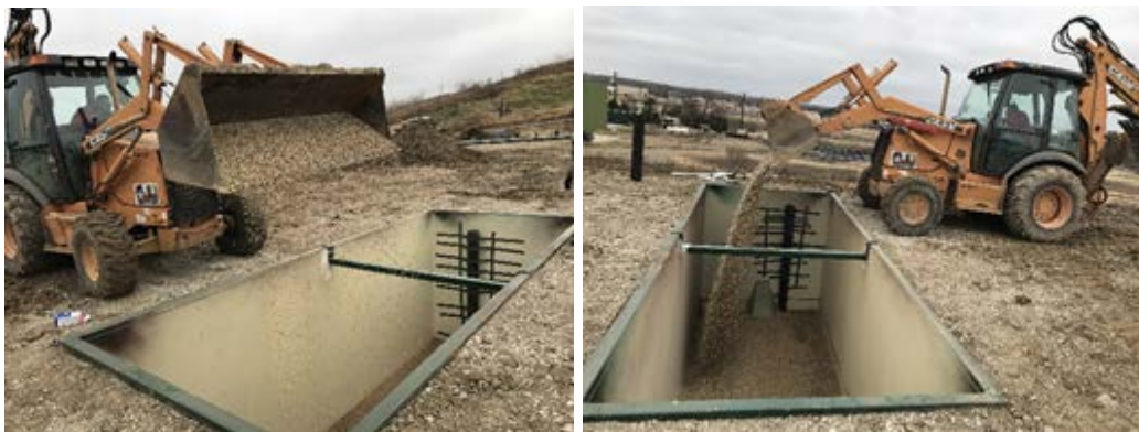
Figure 5-12 Pouring pea-gravel in the cells
