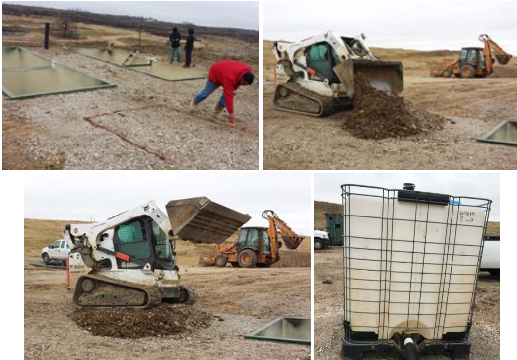
Figure 5-24 Construction of platform for leachate storage tank and placement
