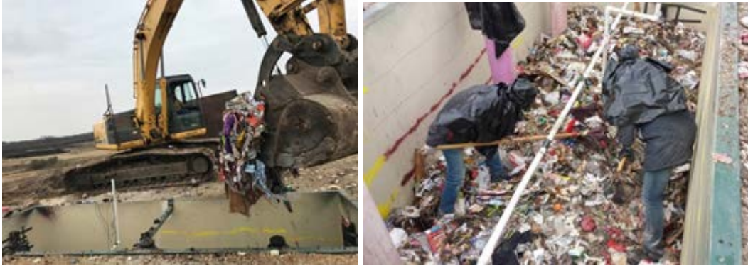
Figure 5-18 Waste filling in the cell
