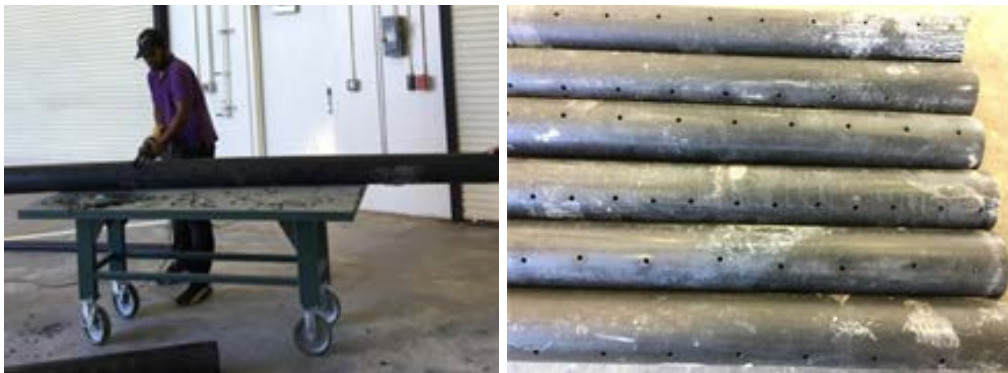
Figure 5-28 Gas well cutting and perforation
