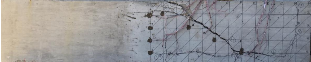
Figure 461 RC control beam #1
