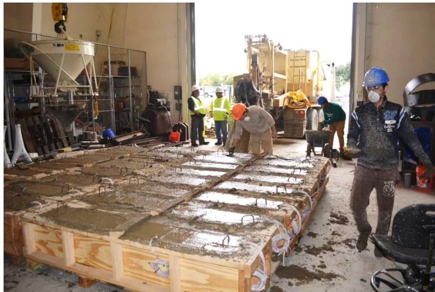
Figure 33 Typical photo of casted large-scale beams
