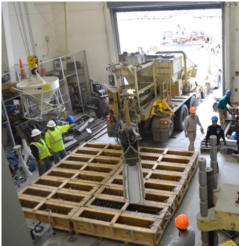
Figure 28 Typical photo of concrete casting at the CELB, UTA
