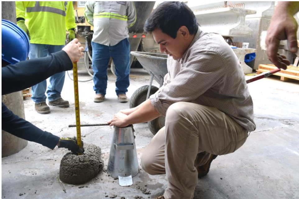
Figure 29 Typical photo of measuring slump of concrete during casting
