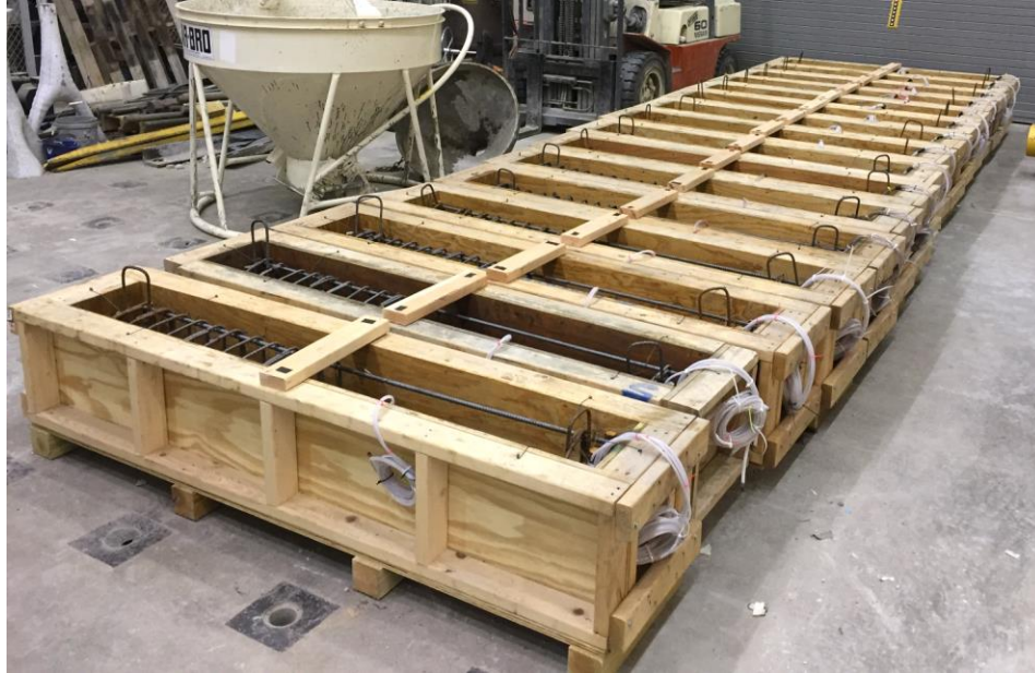
Figure 27 Typical photo of formworks ready for casting
