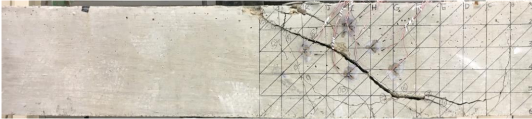
Figure 470 RC control BM# 10
