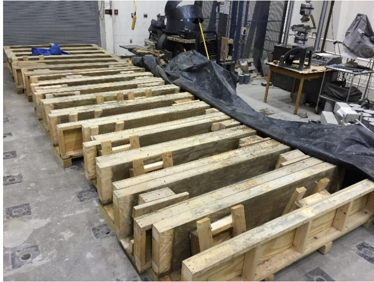
Figure 30 Typical photo of demolded formworks ready for second stage of casting
