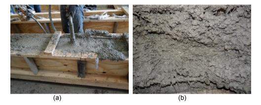
Figure 3-14 (a) Pouring of concrete in formwork and compacting with needle vibrator
