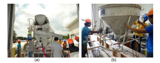
Figure 3-13 (a) Ready mix truck (b) Concrete bucket used for casting beams
