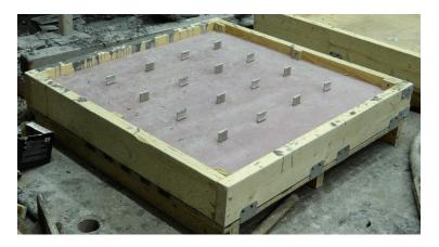
Figure 7-6: Connector ties (tying both front and back wythes)
