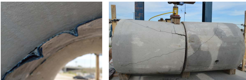
Figure 5-33 - Local buckling of CFRP coupler and crack pattern on springline
