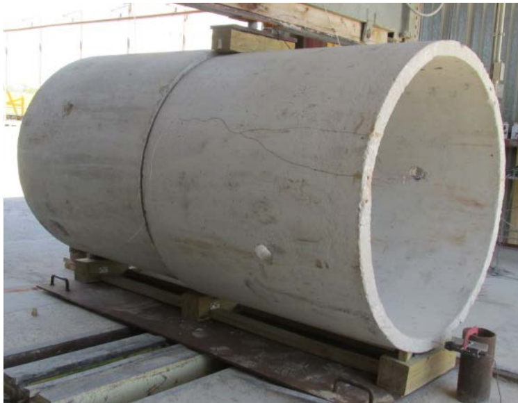
Figure 5-39 - Compressive failure on concrete pipe for TW-36-0.25
