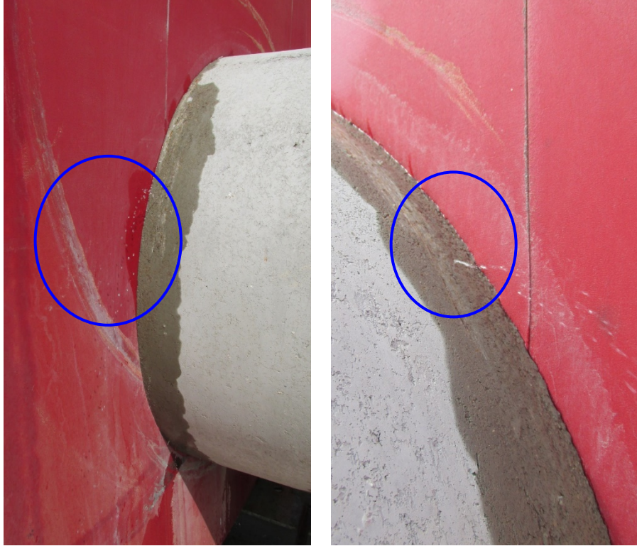
Figure 5-63 - The 1 st leakage on the concrete pipe wall
