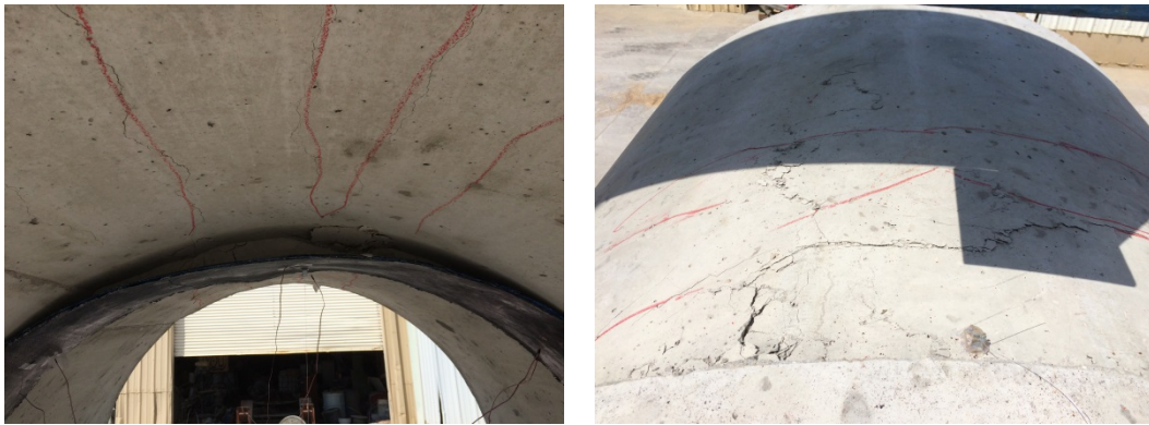
Figure 5-50 - Collapse of the CFRP internal coupler for TW-72-0.375 specimen
