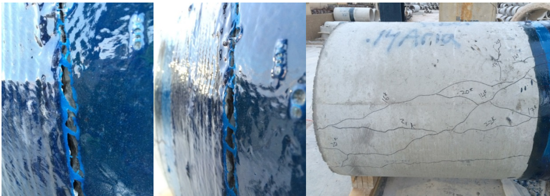
Figure 5-9: Flaking of concrete (Mode I)
