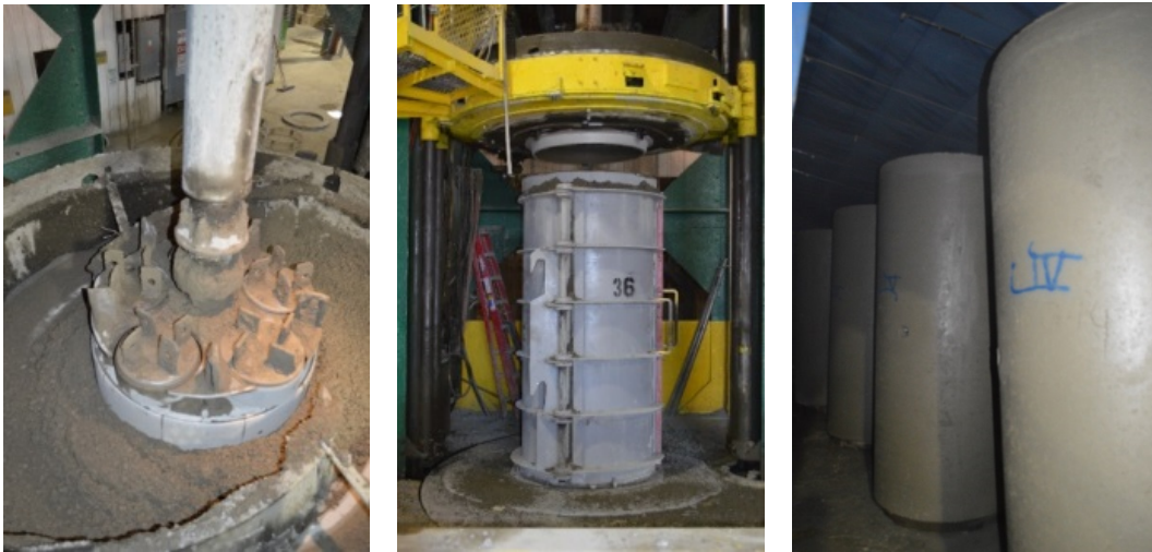
Figure 5-1 - Production of thin-wall concrete pipe: (a) Packerhead, (b) Steel mold, and (c) Steam curing
