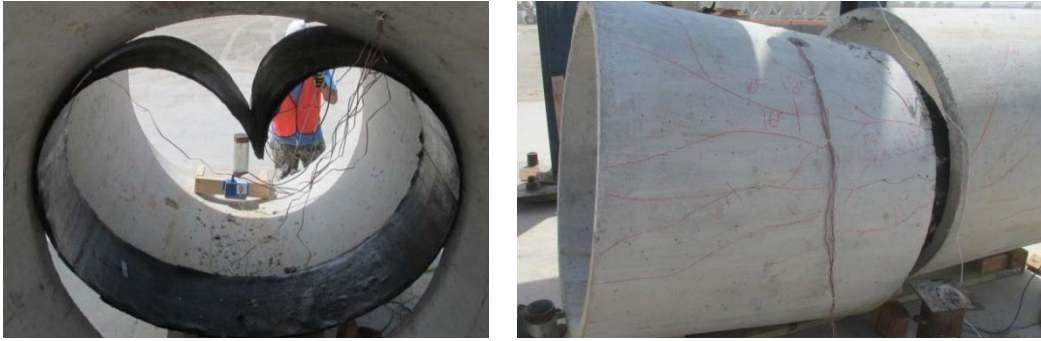
Figure 5-43 - Collapse of the CFRP internal coupler for TW-48-0.1875 specimen
