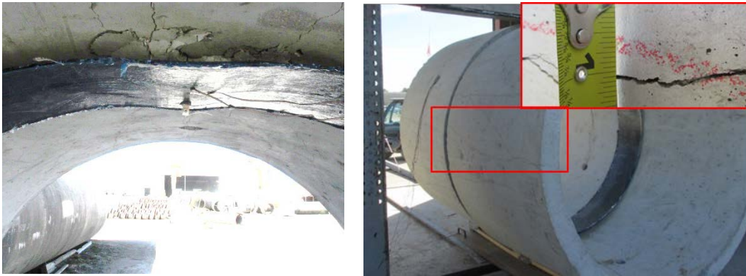
Figure 5-49 - Collapse of the CFRP internal coupler for TW-72-0.25 specimen
