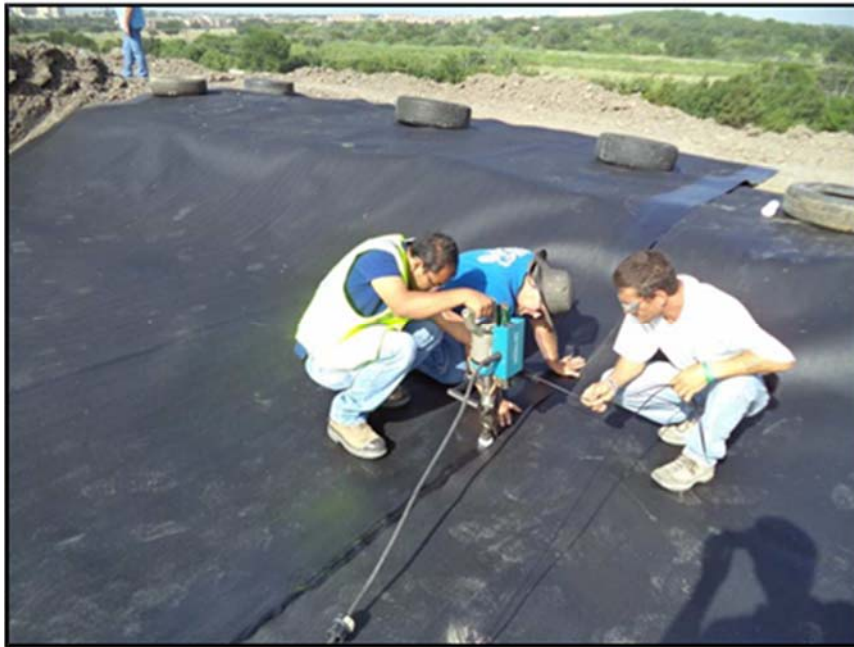
Figure A.83: Welding of the geomembrane by UTA-three (3).
