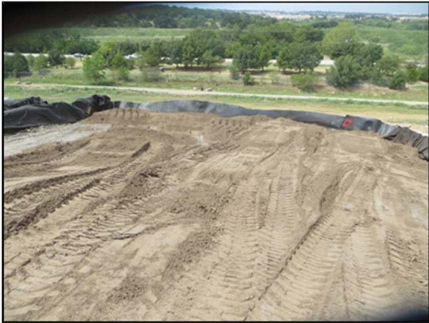
Figure A.368: Topsoil placed in the north inclined section.
