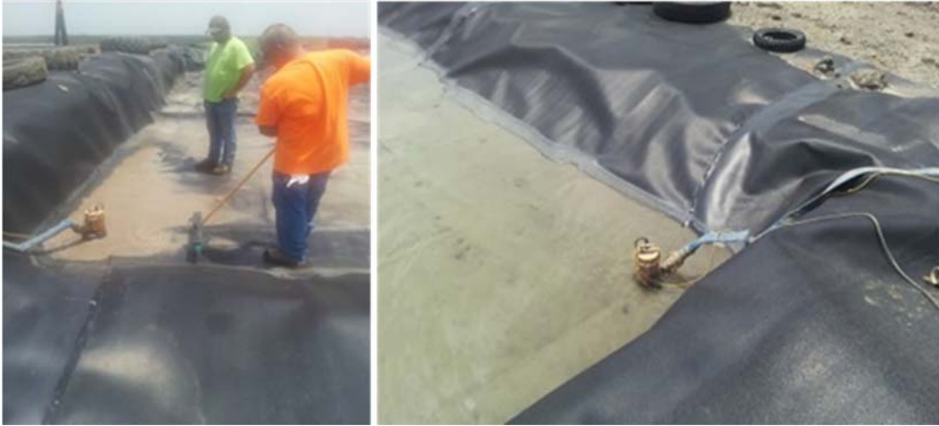
Figure A.130: North Top Section lysimeter (pumping out water)
