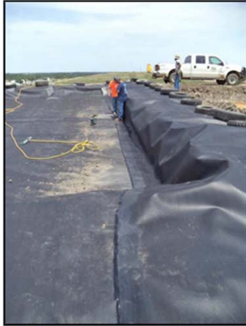
Figure A.103: Construction of the sidewall geomembrane for the middle lysimeter.
