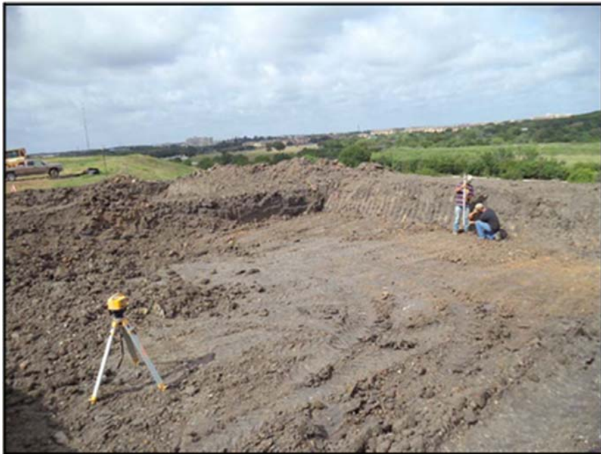
Figure A.69: Slope verification by the laser level.
