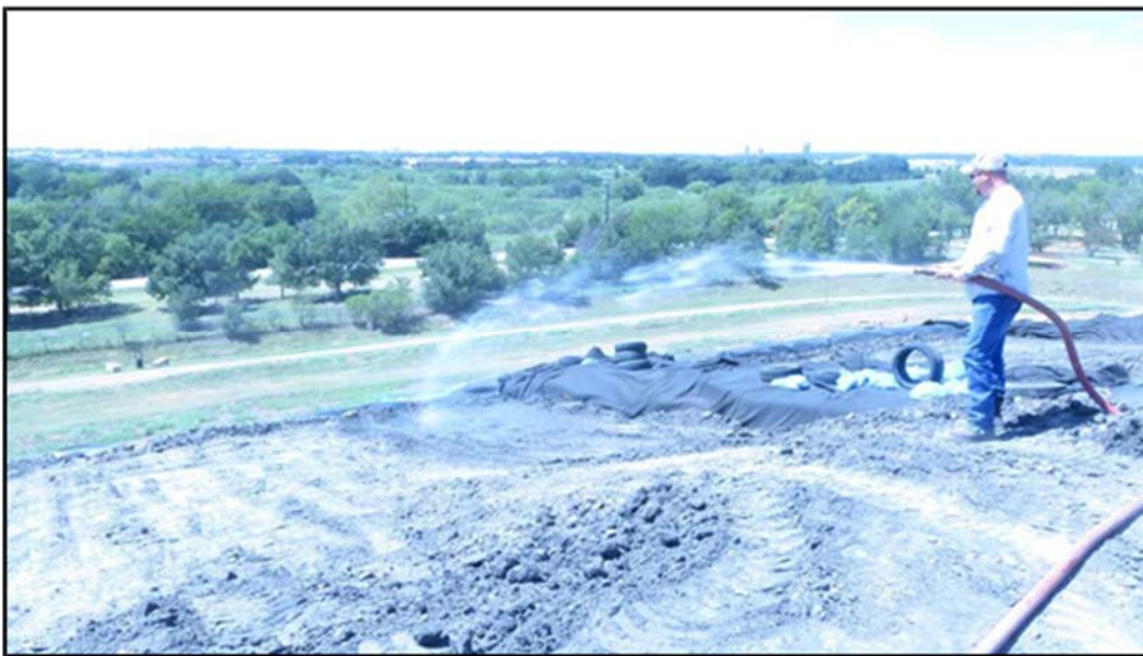
Figure A.317: Applying water to an inclined selection.
