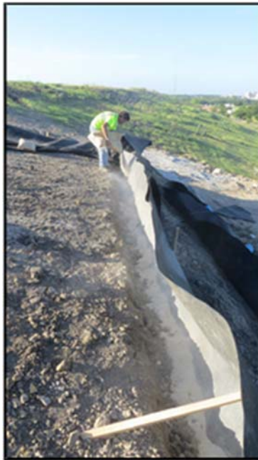
Figure A.336: Placing sodium bentonite around the edges of a lysimeter-two (2).
