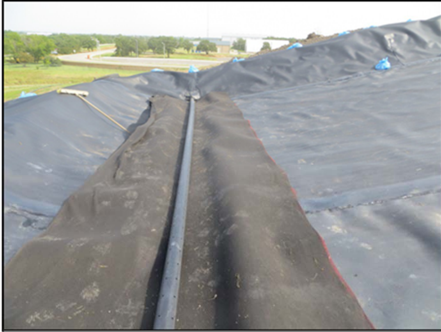
Figure A.286: Geocomposite drain and sandbag placement for the "burrito wrap."
