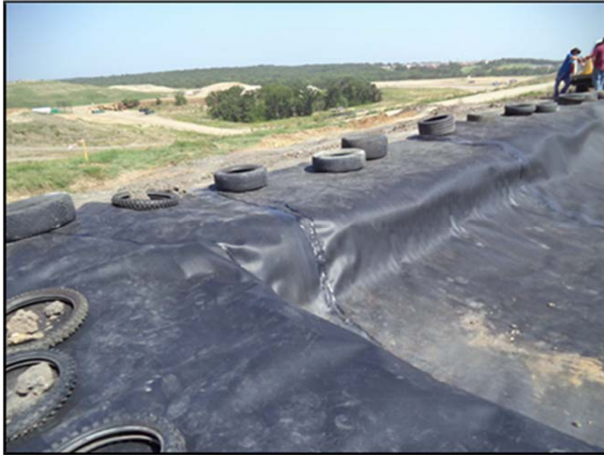
Figure A.92: Geomembrane placed in the North top section lysimeter-two (2).
