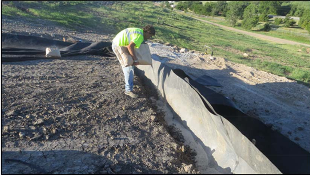
Figure A.335: Placing sodium bentonite around the edges of a lysimeter-one (1).
