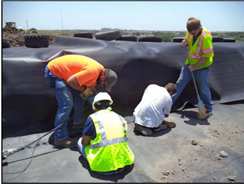
Figure A.86: Sidewall geomembrane welding and cleaning of welding area.
