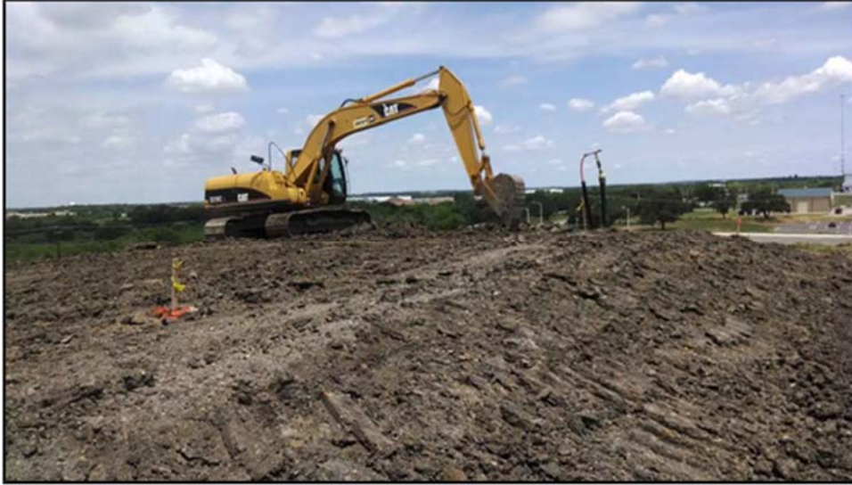
Figure A.45: Beginning of the excavation of the top section.
