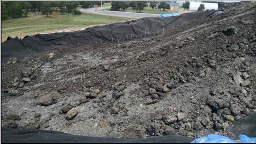
Figure A.308: 1 st soil layer placed in the north inclined section.
