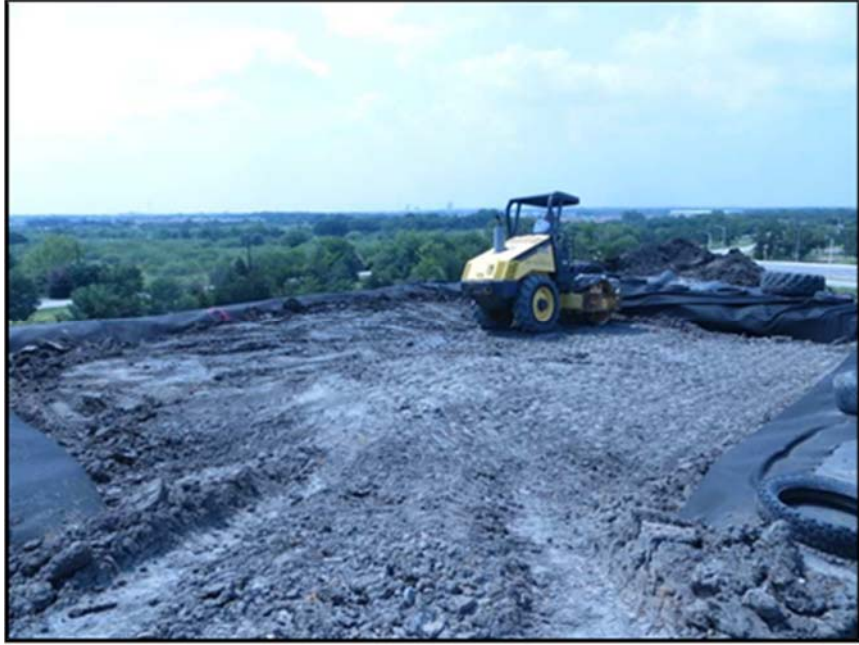
Figure A.232: Sheep-footed compactor used in north top section.
