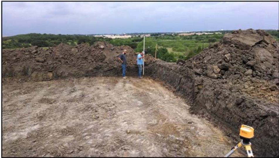
Figure A.50: Subgrade slope and height verification by laser level.
