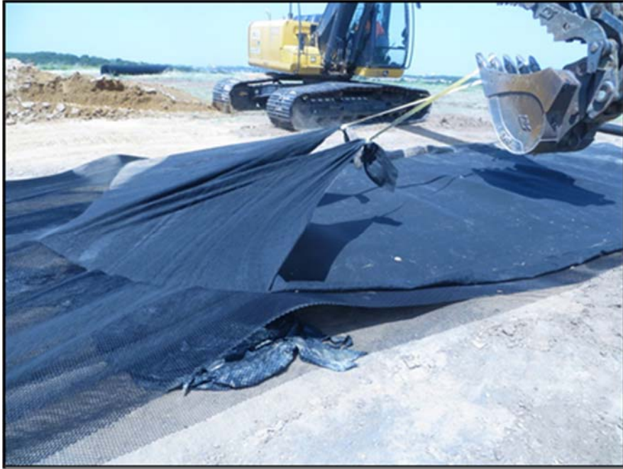
Figure A.300: Removal of the geotextile from the geocomposite drain.
