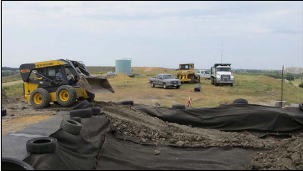
Figure A.156: Ramp construction in the south top section lysimeter.
