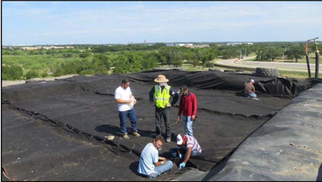
Figure A.140: Joining adjacent geocomposite sheets by COD and UTA personal.
