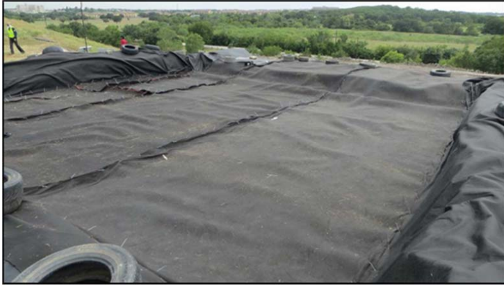
Figure A.146: South top section lysimeter ready for soil placement-two (2).
