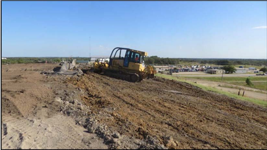
Figure A.377: Placing soil near the sidewalls and adjusting the embankment.
