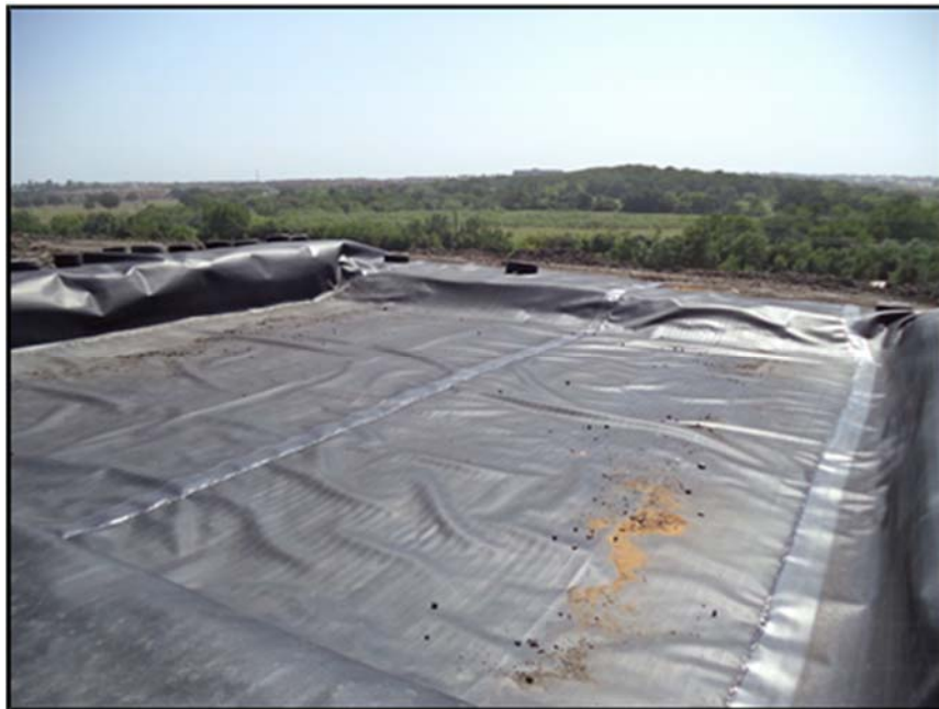
Figure A.91: Geomembrane placed in the North top section lysimeter-one (1).
