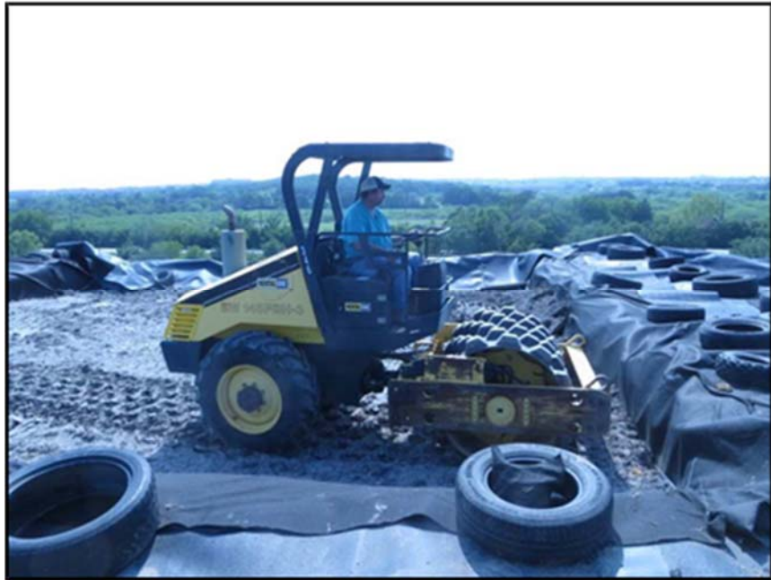
Figure A.226: Sheep-footed compactor on the south top section-one (1).
