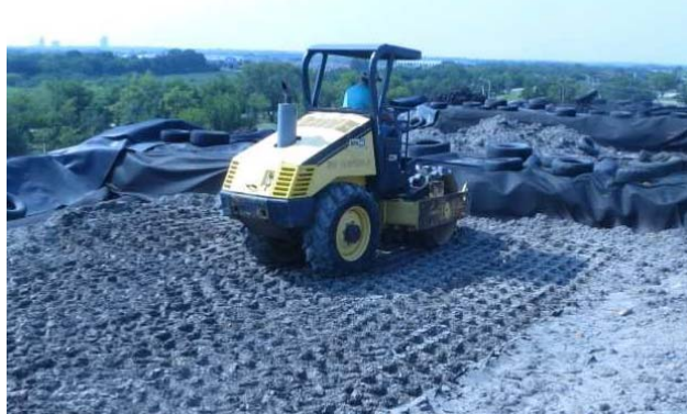
Figure 4.14: Compacted clay placement a) placement of clay by a skid-steer, b) water application for compaction purposes, c) sheep-footed compactor utilization.
