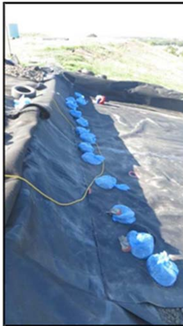
Figure A.276: Sandbag placement along the middle berm.
