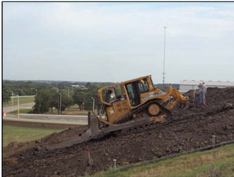
Figure A.29: Inclined section embankment construction and water application.
