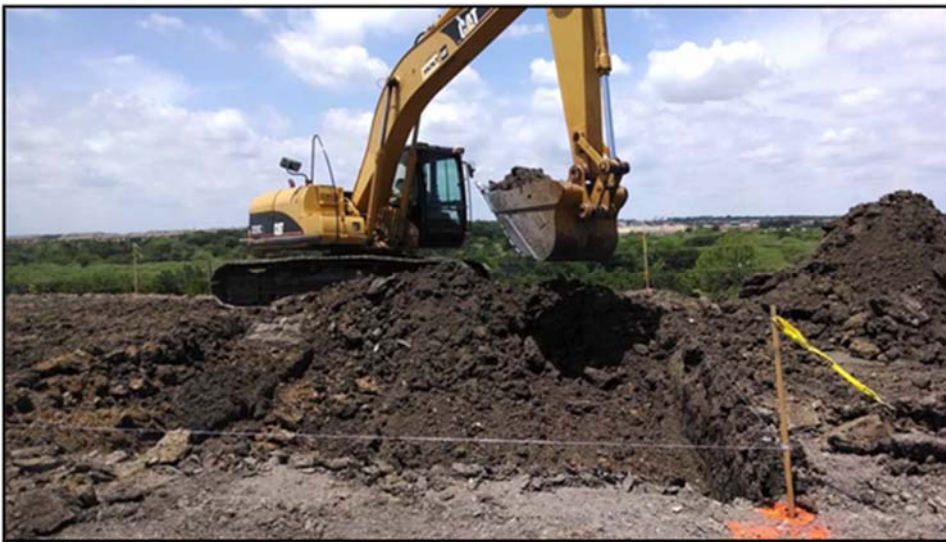
Figure A.46: Excavation and placement of soil on the embankment.
