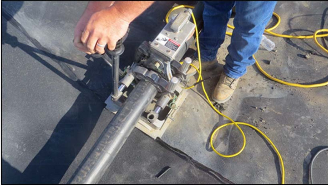
Figure A.279: Cutting the HDPE pipe in preparation for welding.
