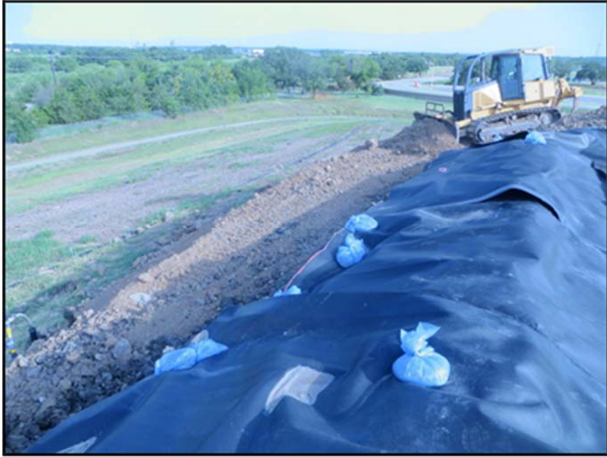
Figure A.289: Roadway constructed below the north inclined section.
