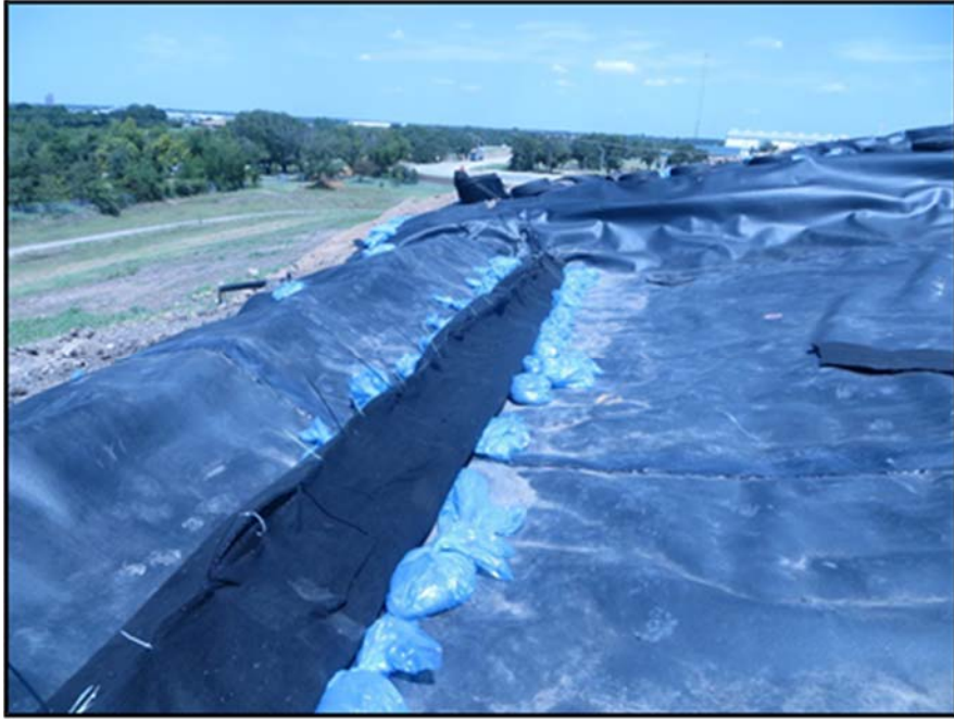
Figure A.295: Completed “burrito wrap” in the middle inclined section.
