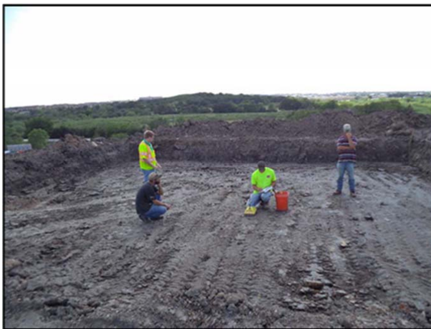
Figure A.70: Nuclear density test on the subgrade by D&S.
