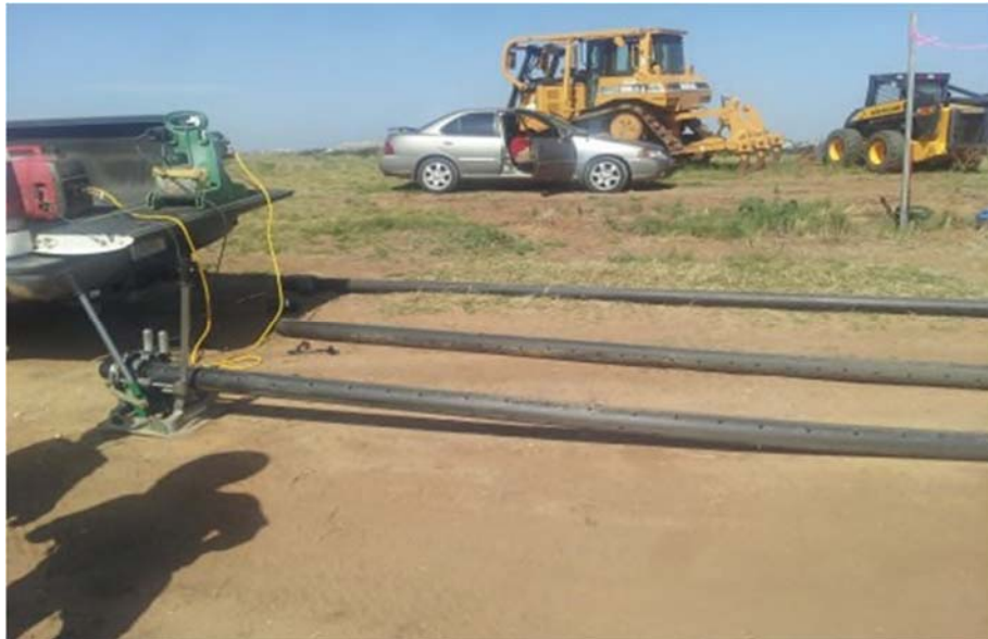
Figure A.133: Perforated pipes on site, the caps being welded.
