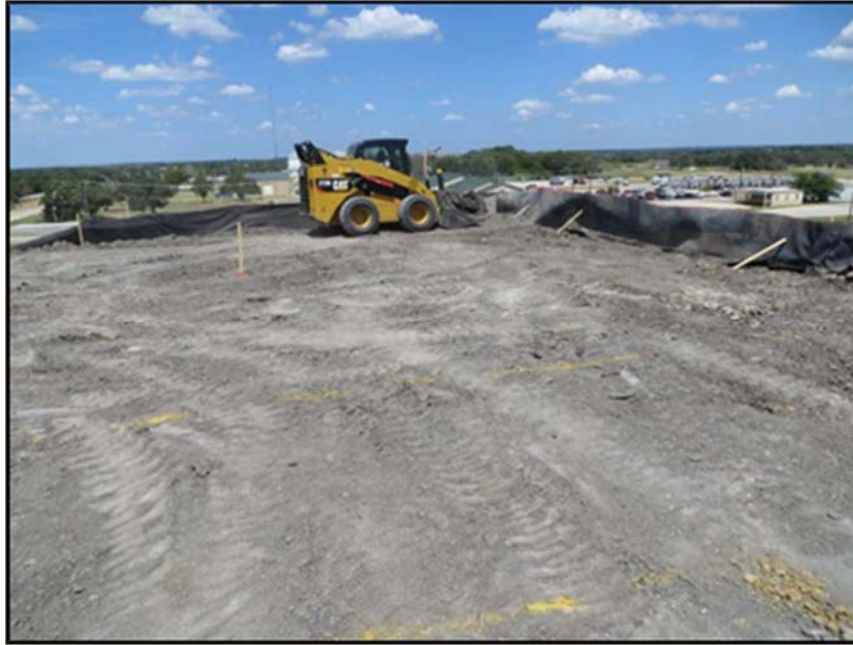
Figure A.344: Adjusting the compacted clay in the north top section.
