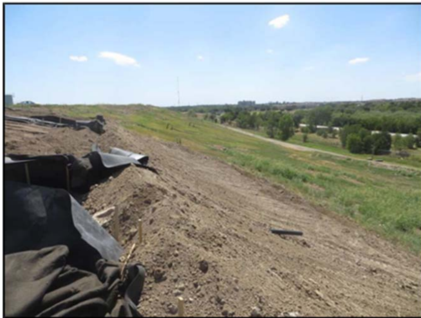
Figure A.378: Embankment below the lysimeters after adjustment.
