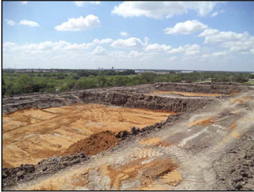
Figure A.78: Nearly completed top section subgrades.
