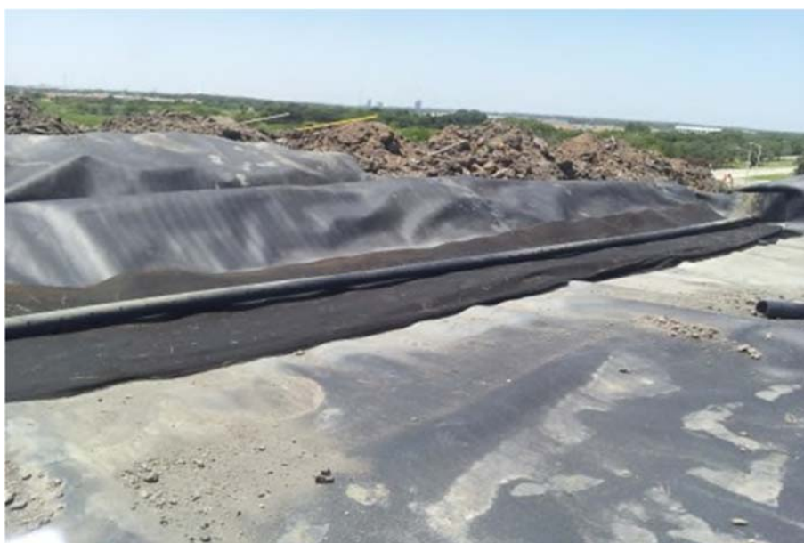
Figure A.135: The geotextile placed below the perforated pipes. Burritos to be made tomorrow.
