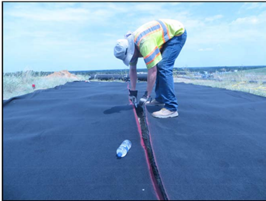
Figure A.285: Cutting the geocomposite drain.
