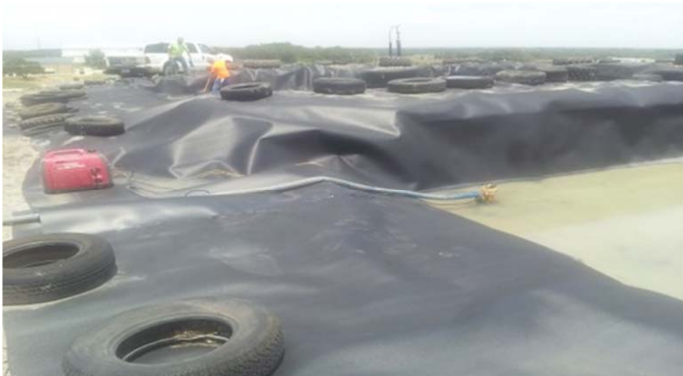
Figure A.131: Middle Top Section lysimeters (pumping out water).
