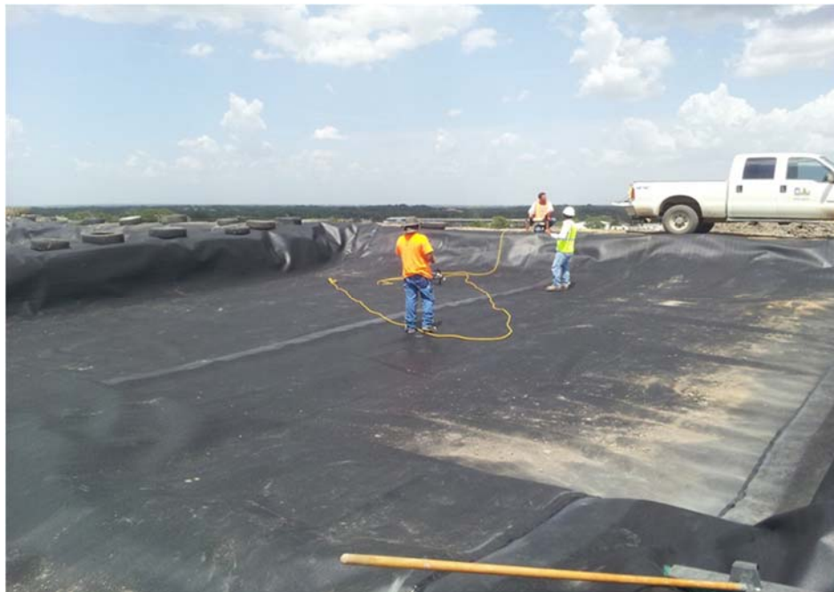
Figure A.121: South Top Section lysimeters (after completion)
