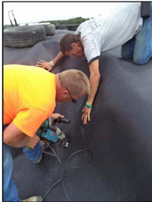
Figure A.102: Welding of the sidewall geomembrane.
