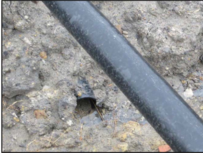
Figure A.184: Flow of water from the middle top section.
