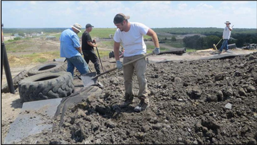
Figure A.328: Removing soil from the lysimeter boundaries-one (1).
