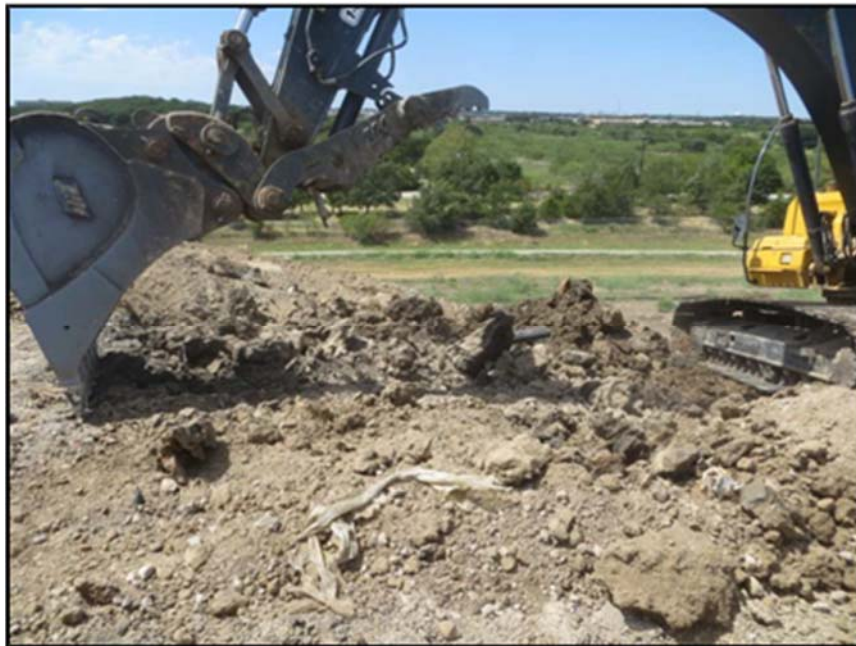
Figure A.380: Removing soil near the percolation pipes.
