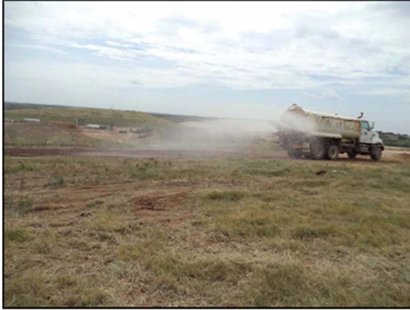
Figure A.18: Water application to the temporary access road.
