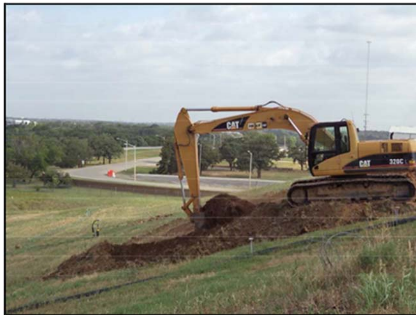
Figure A.4: Removal of top soil from the inclined section.
