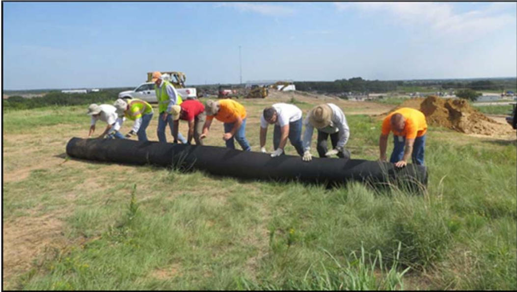
Figure A.267: Rolling of geomembrane to the appropriate length.
