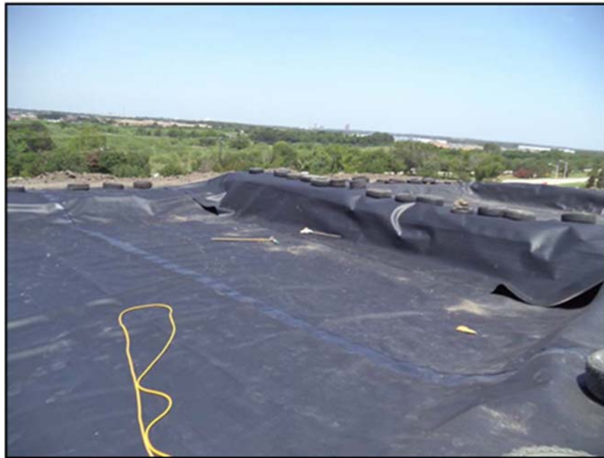
Figure A.95: Geomembrane placed during the thirteenth day and welding details.
