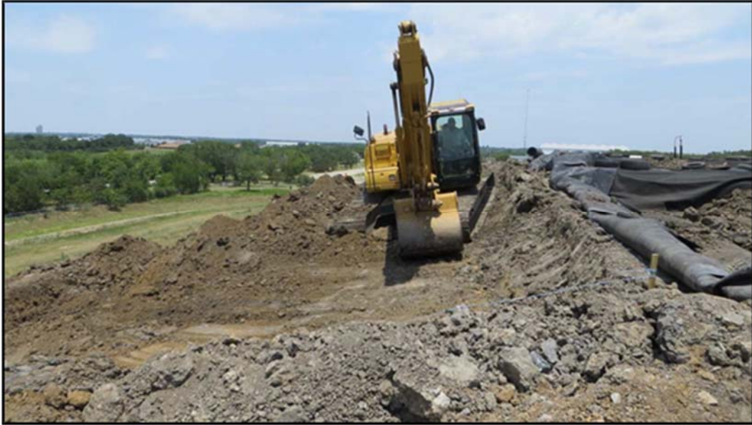
Figure A.154: Excavation of the south inclined section lysimeter-two (2).
