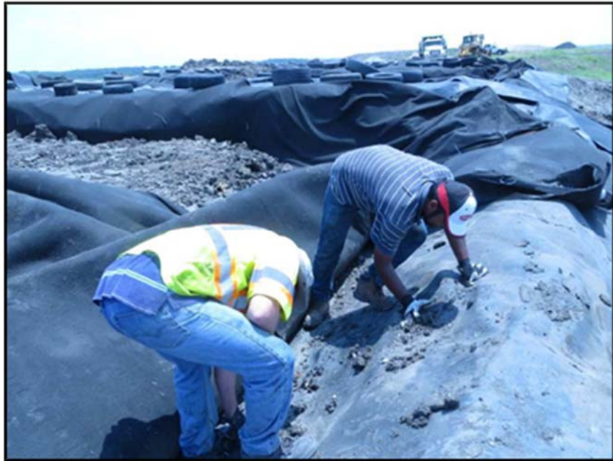
Figure A.239: Removal of soil near the percolation pipe.
