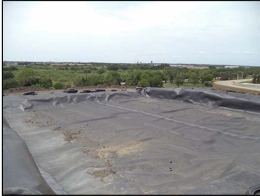
Figure A.107: North top section geomembrane details from the Southeast.
