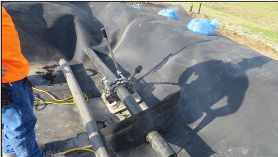
Figure A.280: Welding of the HDPE pipe.
