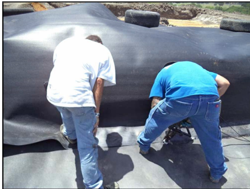
Figure A.85: Sidewall geomembrane welding to subgrade geomembrane by COD staff.
