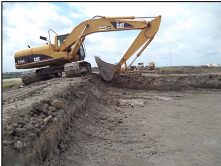
Figure A.73: Subgrade berm finalization for a top section.
