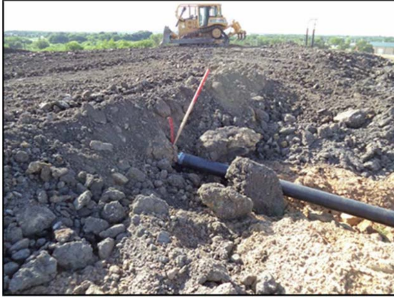
Figure A.24: Leachate injection well slightly covered by the embankment.
