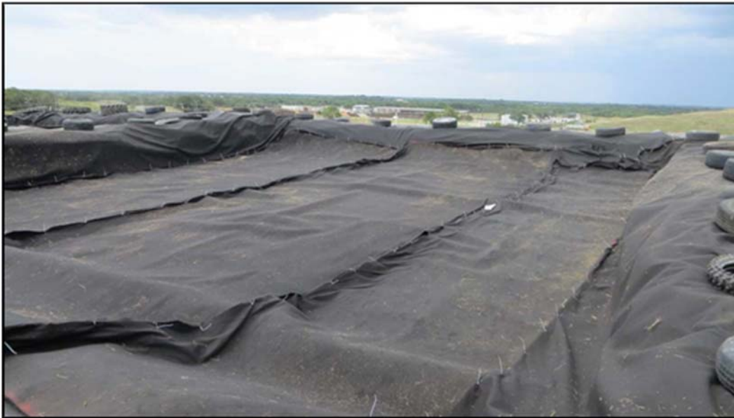
Figure A.147: Middle top section lysimeter ready for soil placement-one (1).
