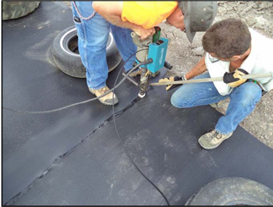
Figure A.96:Welding of the subgrade geomembrane.
