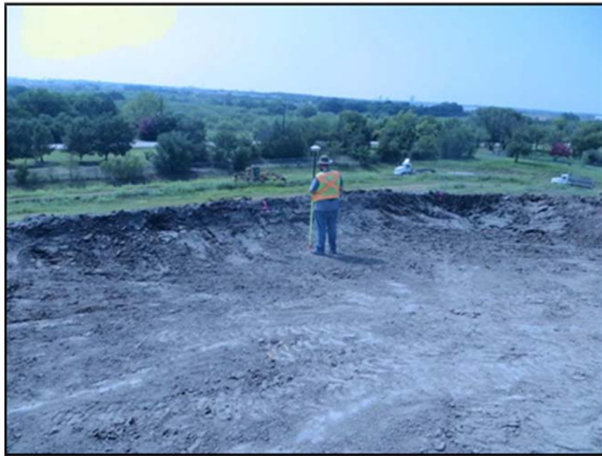
Figure A.259: Surveyor taking a subgrade elevation in an inclined section.
