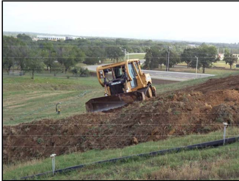
Figure A.3: Stripping of top soil from the inclined section.
