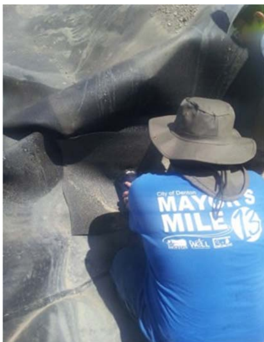
Figure A.134: Boots placed in the north lysimeters.
