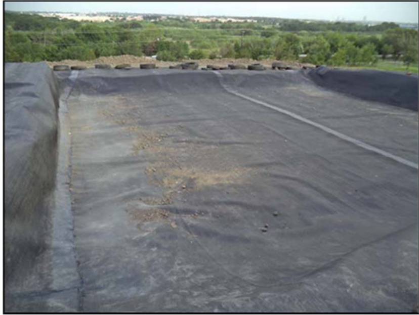
Figure A.98: North top lysimeter geomembrane details-one (1).
