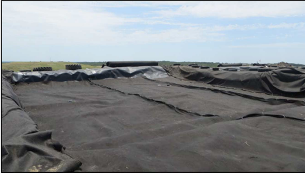
Figure A.136: Placement of the geocomposite drain in a lysimeter-one (1).
