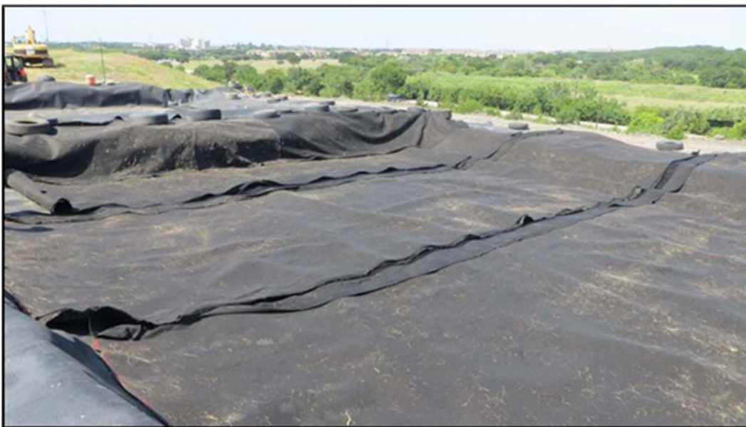
Figure A.137: Placement of the geocomposite drain in a lysimeter-two (2).
