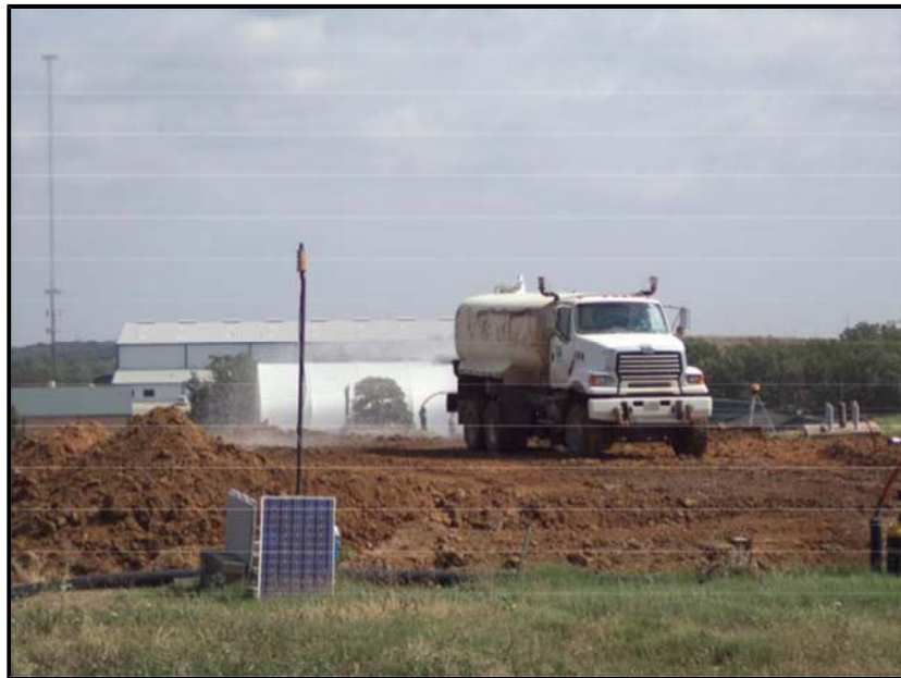
Figure A.6: Water application to the top section for compaction purposes.
