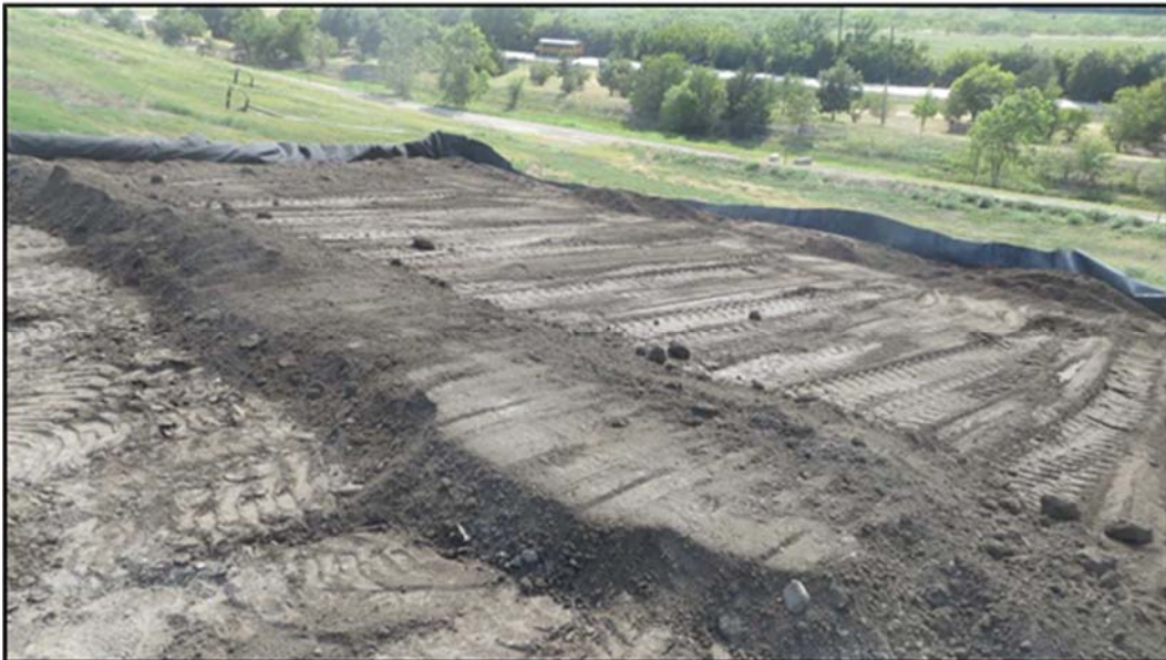
Figure A.373: Topsoil placed in the south inclined section.
