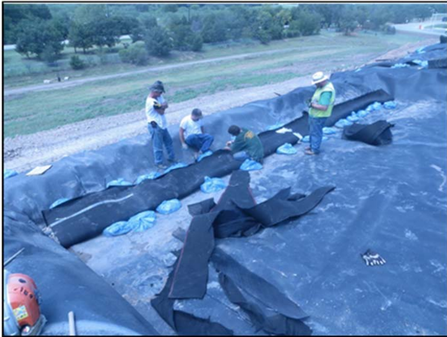
Figure A.296: Nearly completed “burrito wrap” in the south inclined section.
