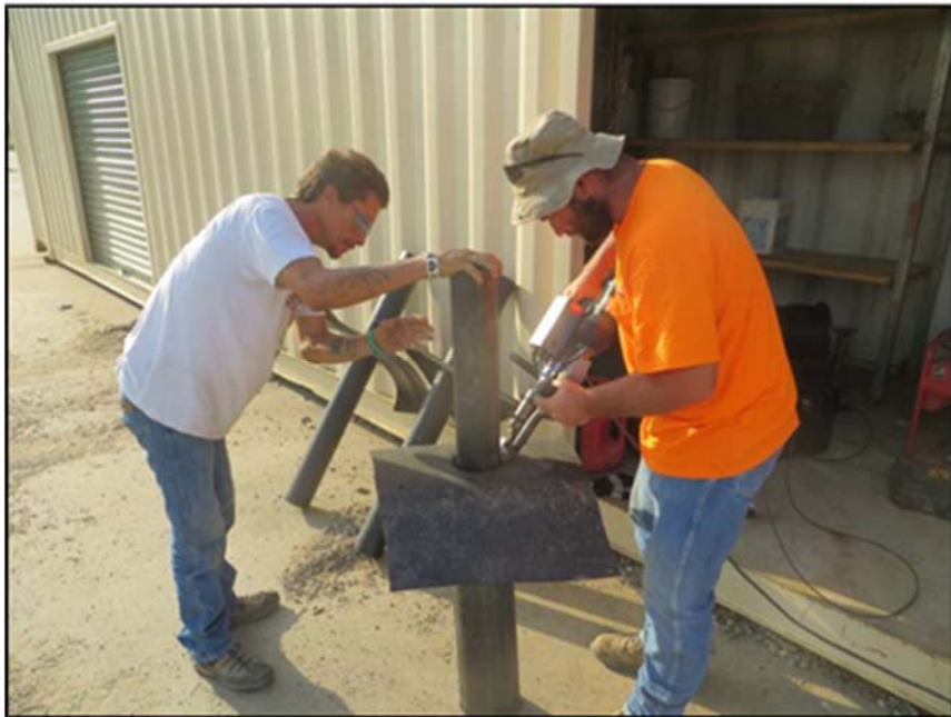
Figure A.274: Welding the geomembrane sheet to the 4-inch HDPE pipe.
