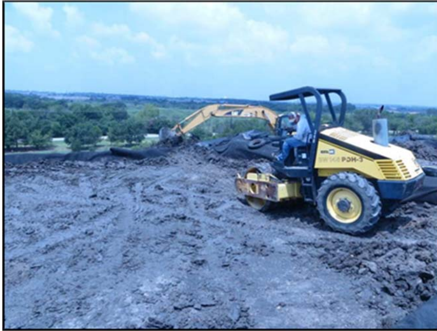
Figure A.230: Sheep-footed compactor used in middle top section.
