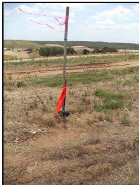
Figure A.10: Marker placed to avoid hitting a vertical leachate injection pipe.
