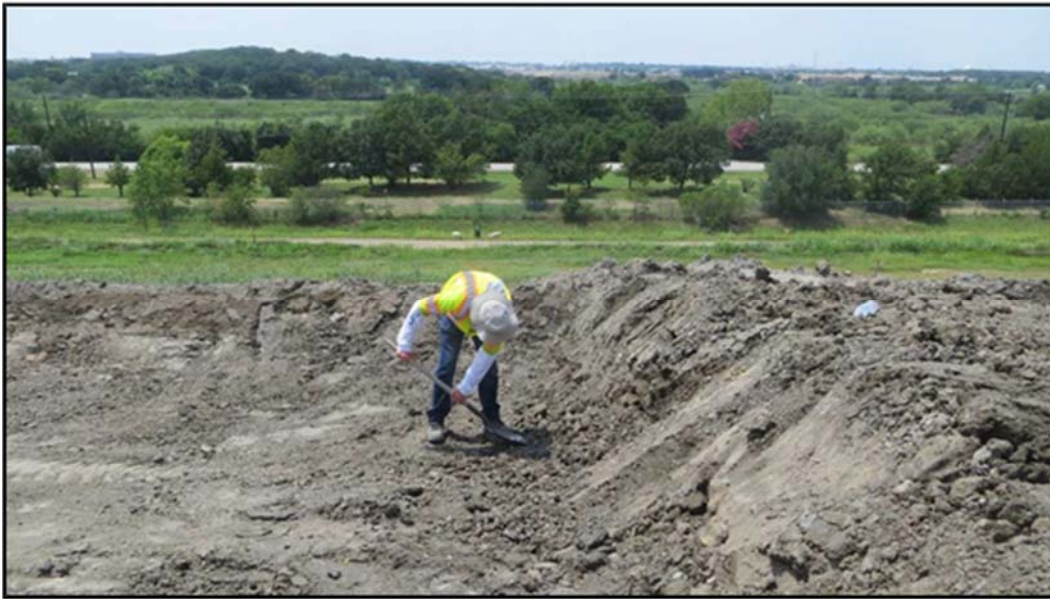
Figure A.257: Removal of subgrade imperfections in an inclined section.
