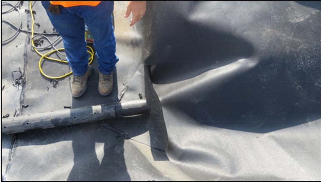
Figure A.281: Boot placement in an inclined section.
