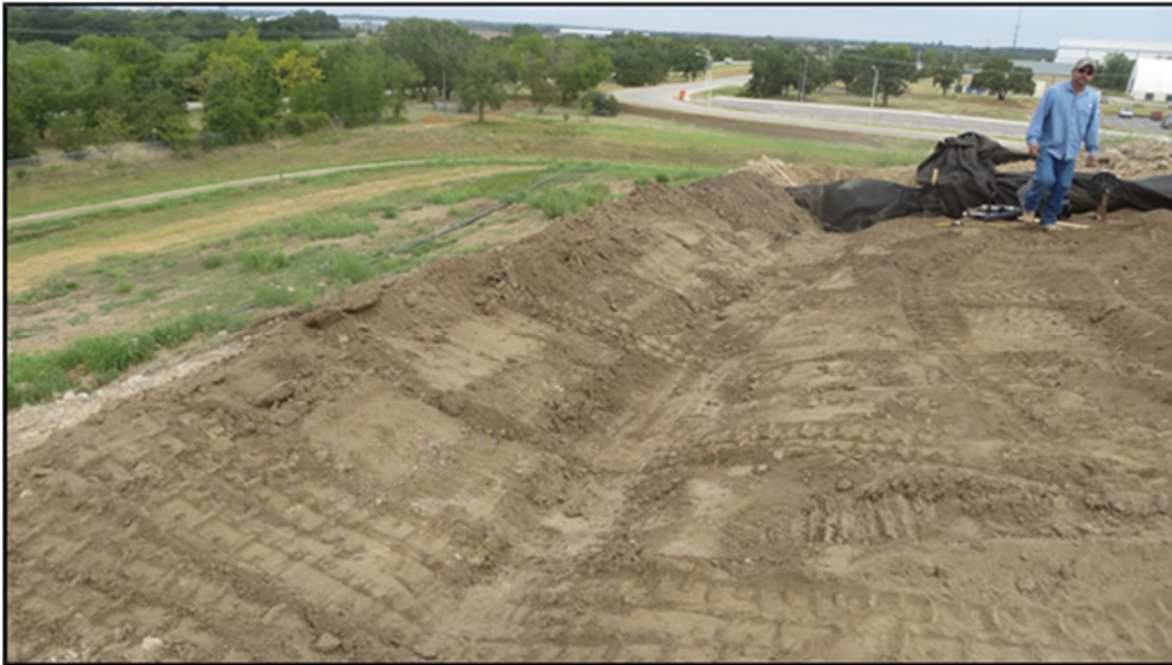
Figure A.381: Berm constructed in an inclined section.
