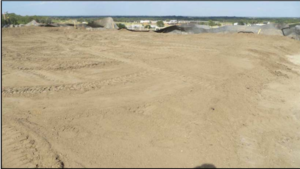
Figure A.372: Topsoil placed in the middle top section.
