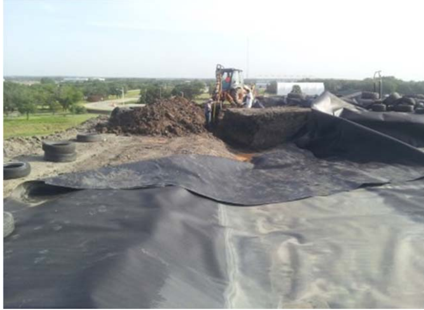
Figure A.132: North Top Section lysimeters, the membranes are pulled to dig the drainage.
