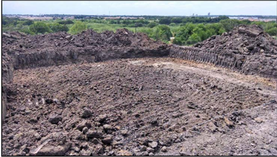
Figure A.47: Test section excavation nearing completion.
