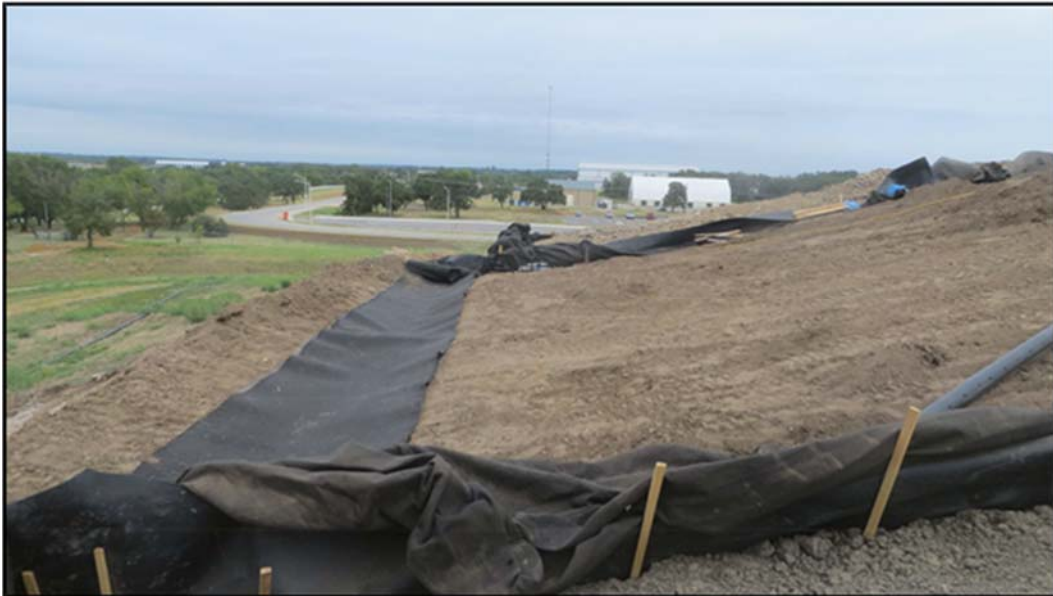
Figure A.383: Liner and geocomposite drain placement.
