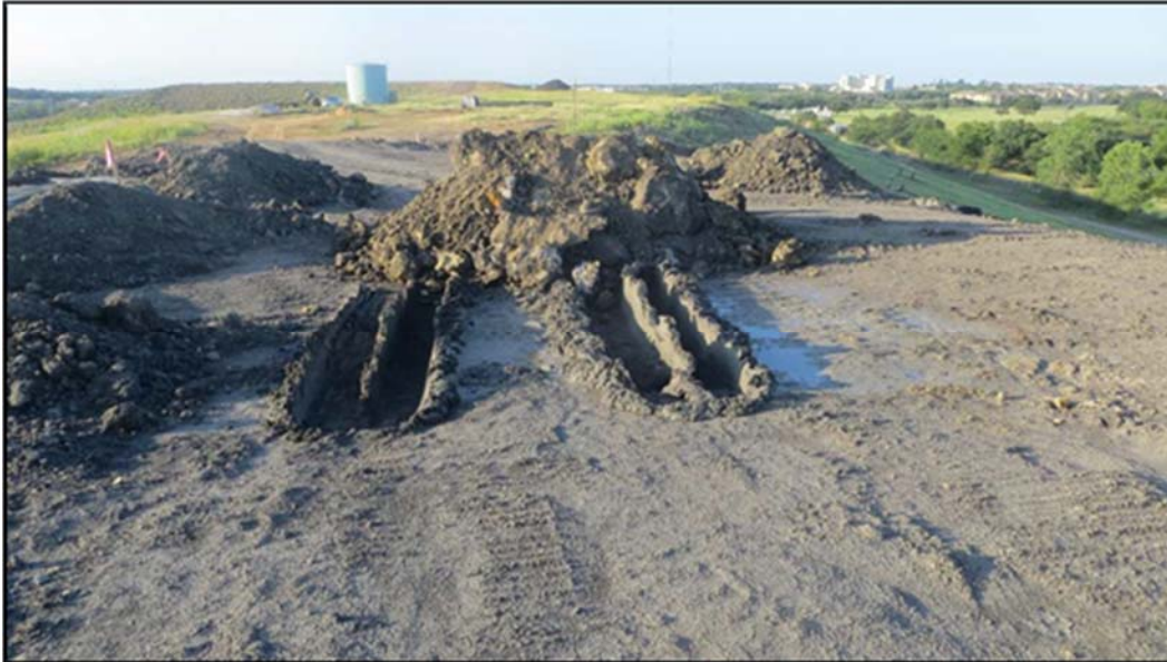
Figure A.331: Results of the dump truck running into a wet spot.
