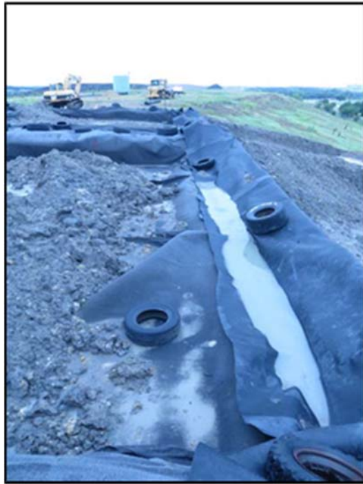
Figure A.199: Details of the north top section lysimeter (near piping system).
