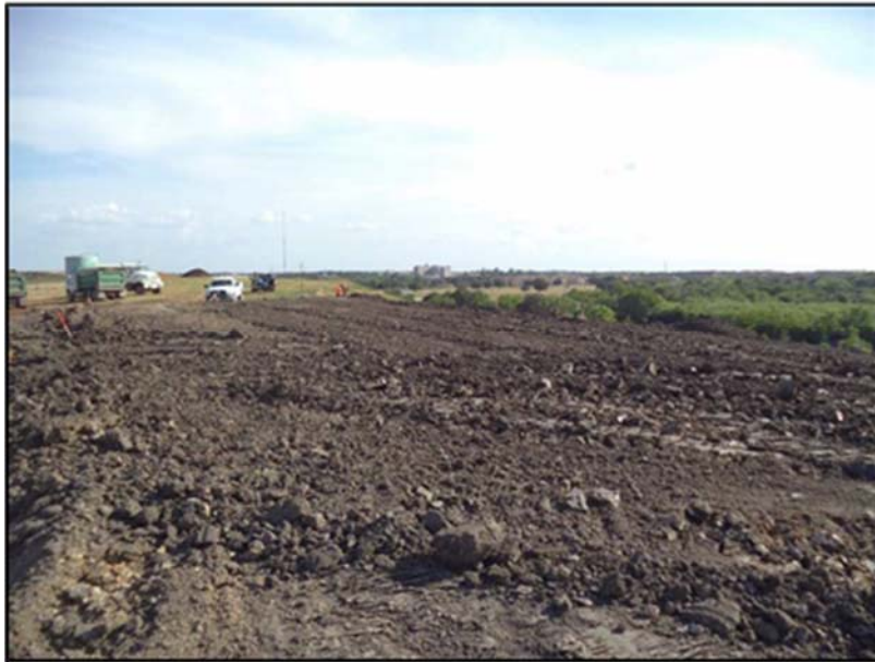
Figure A.21: Top section embankment completion two (2).
