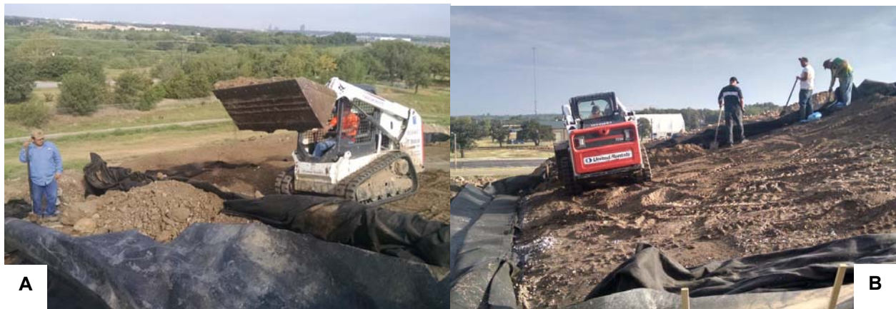
Figure 4.20: Berm construction a) between two (2) lysimeters and b) within a lysimeter.
