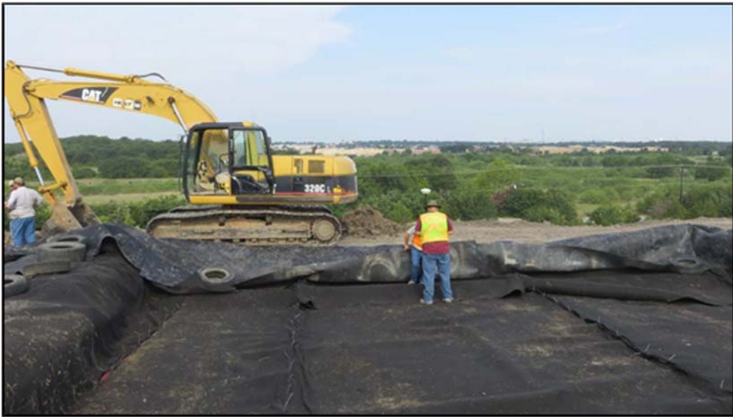
Figure A.155: Surveyors taking an elevation in the bottom of a lysimeter.
