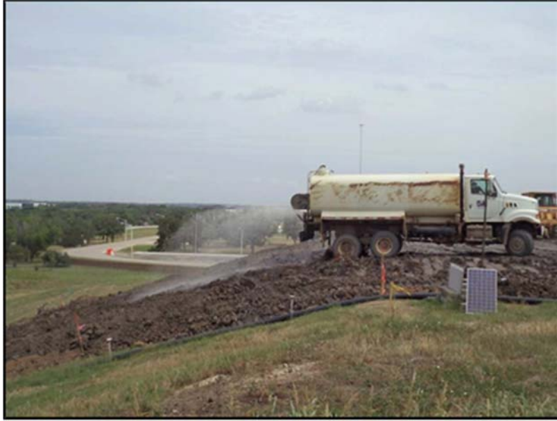
Figure A.16: Water application to ensure adequate compaction.
