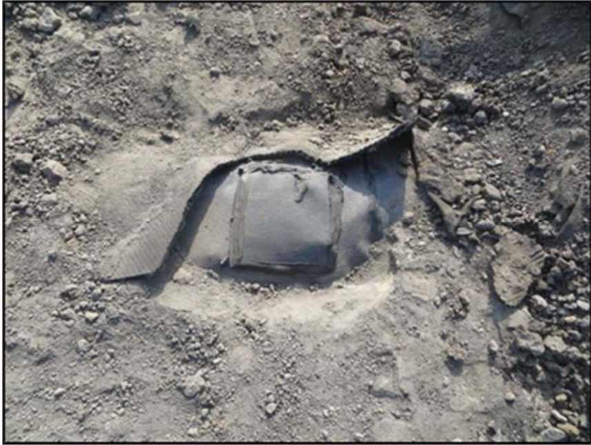
Figure A.367: Repair of the cut in the liner.
