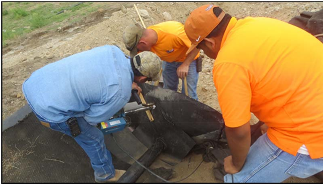
Figure A.384: Welding the boot and liner to the sidewall.
