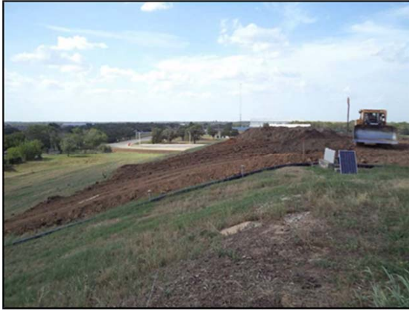
Figure A.14: Embankment construction on the inclined section.
