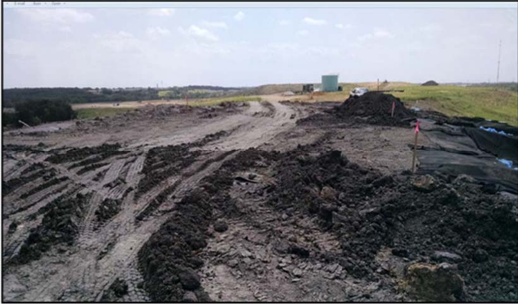
Figure A.306: Geosynthetic protection soil placed on the top sections.
