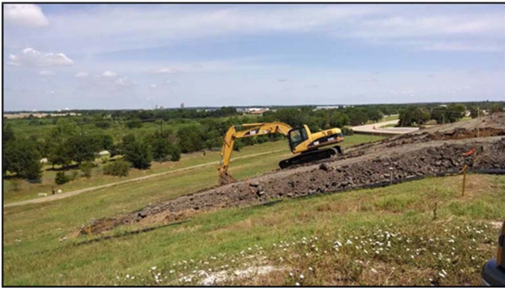
Figure A.42: Embankment edge modification by the excavator.
