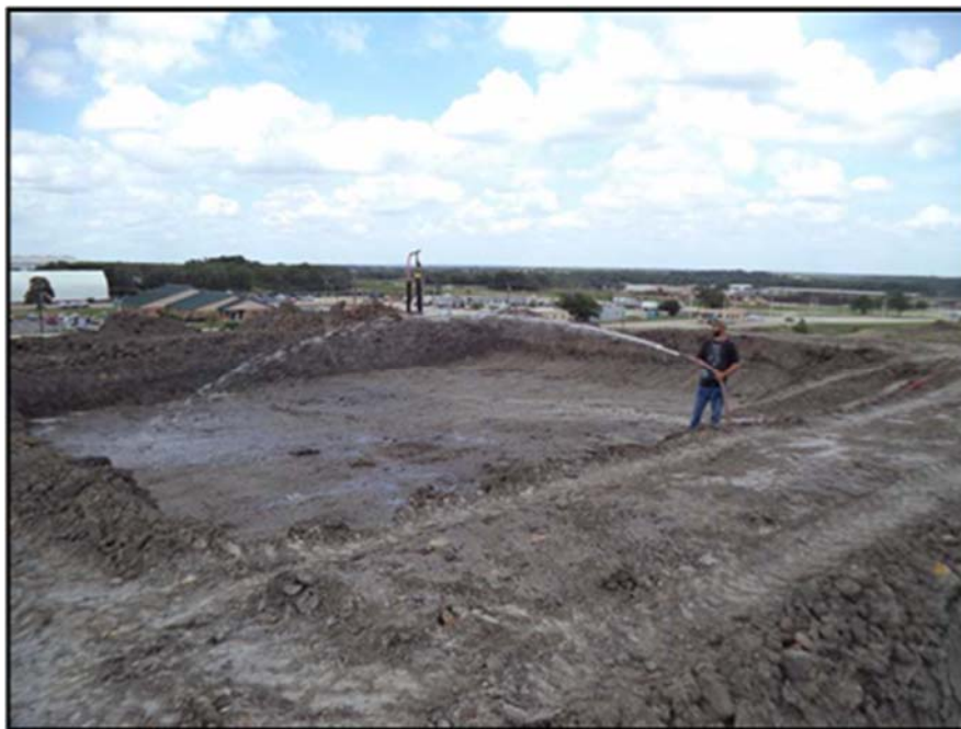
Figure A.66: Water application to the subgrade of the north top section lysimeter.
