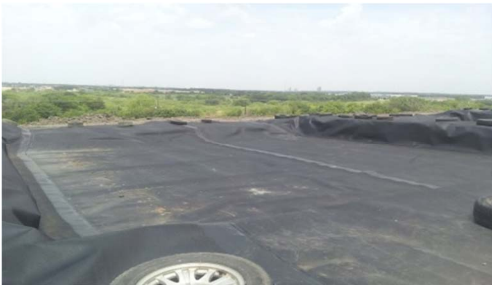
Figure A.129: South Top Section lysimeter on Wednesday.
