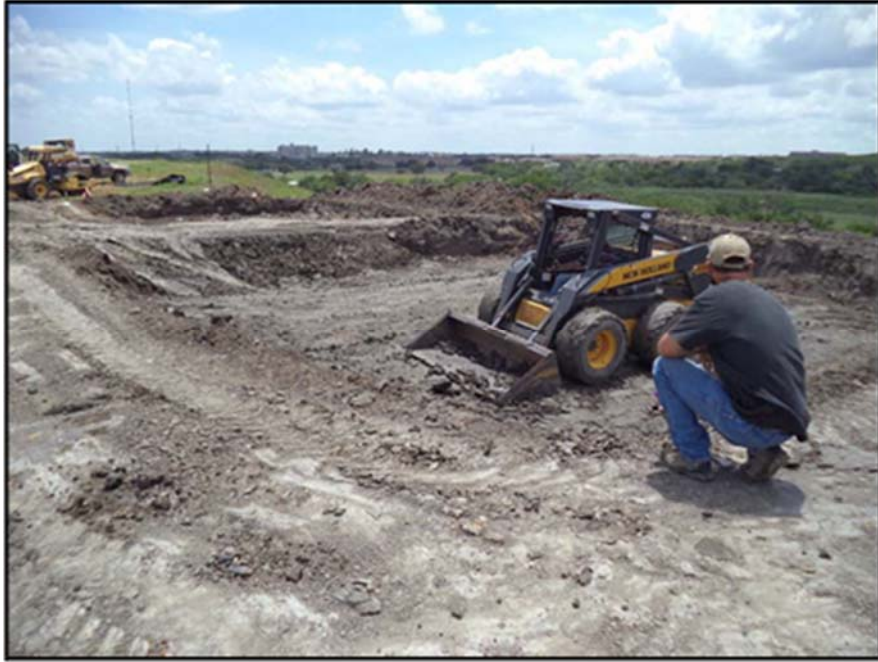
Figure A.68: Subgrade finalization by a skid-steer.
