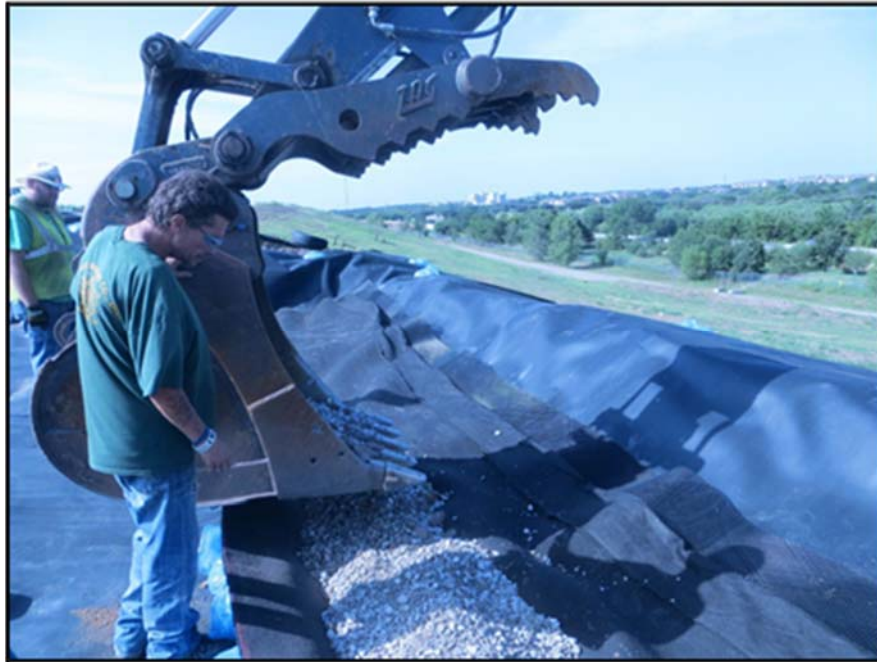
Figure 8: Granular material placement in a "burrito wrap."
