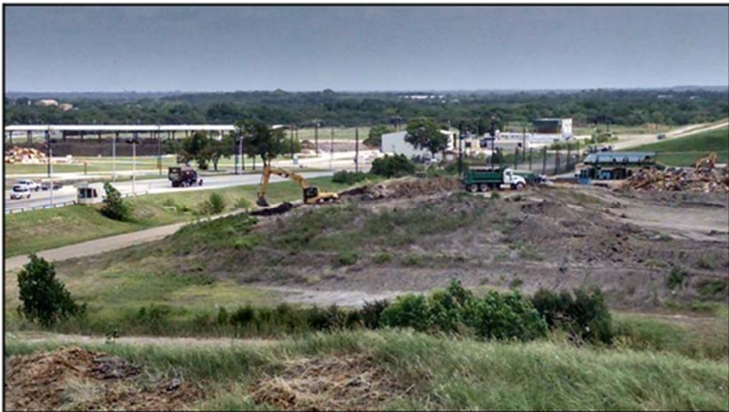
Figure A.309: Obtaining soil from the borrow pit.
