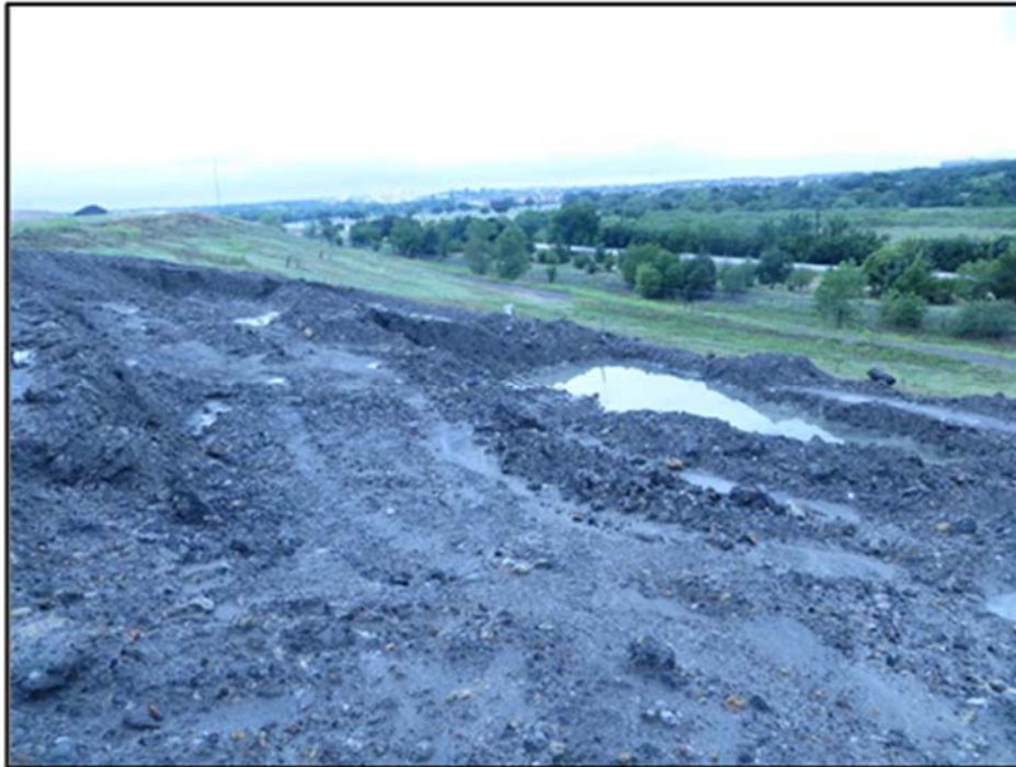
Figure A.207: Middle inclined section details after a rainfall event.
