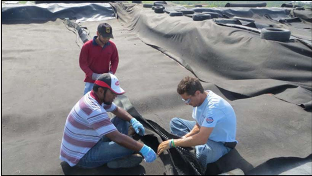
Figure A.138: Placing adjacent geocomposite sheets together in preparation for zip-ties.
