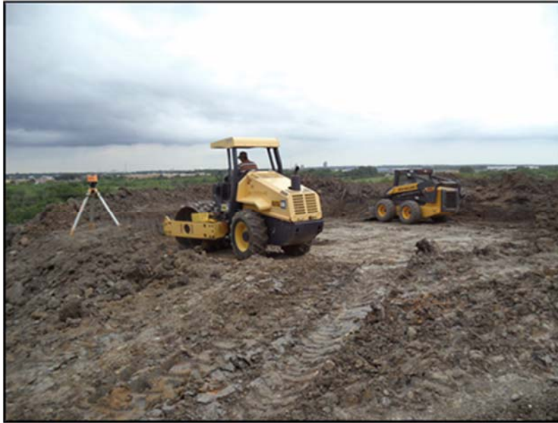
Figure A.59: Compaction and gradation of the south top section.
