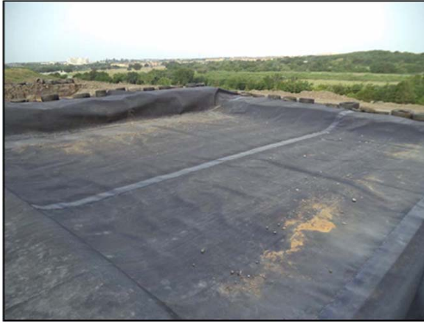
Figure A.100: North top lysimeter geomembrane details-three (3).
