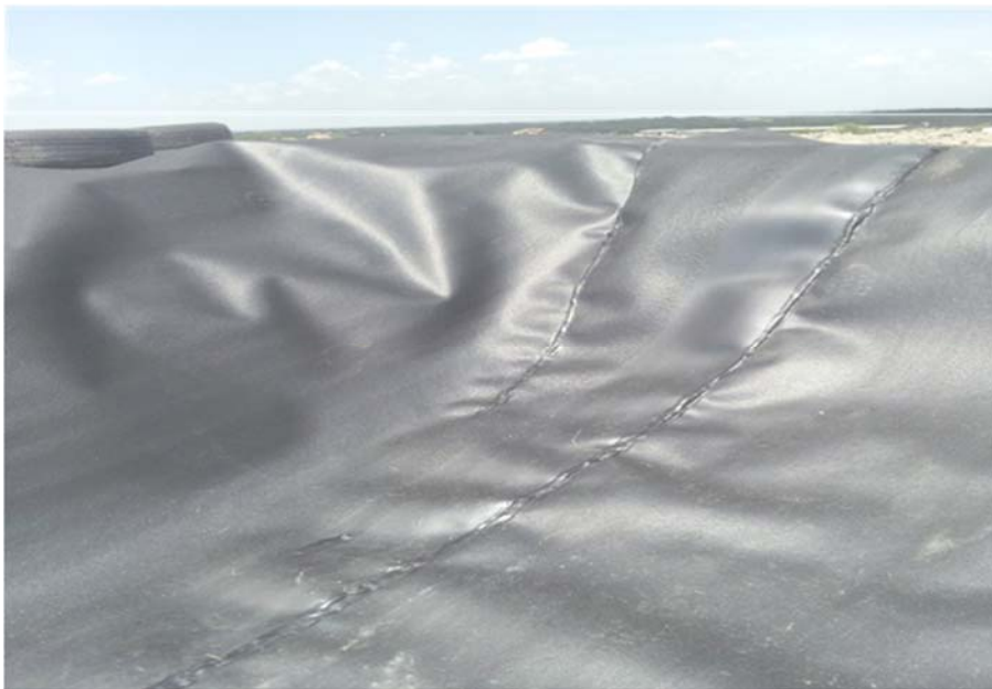
Figure A.125: South Top Section lysimeters (after completion) corner 4
