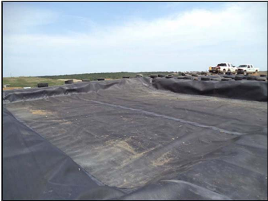
Figure A.106: North top section geomembrane details from the Northwest.
