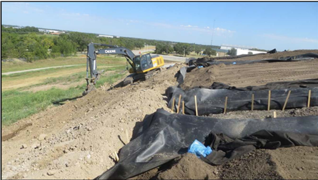
Figure A.376: Placing soil near the sidewalls.
