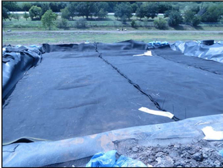
Figure A.299: Geocomposite drain placed in the south inclined section.
