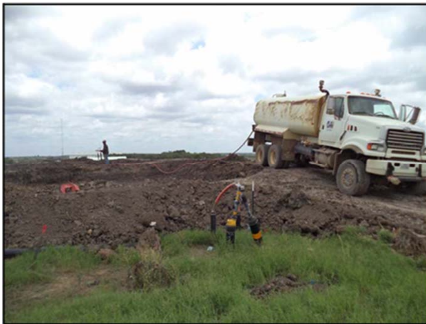
Figure A.65: Water application to the subgrade of the middle and south top section lysimeters.
