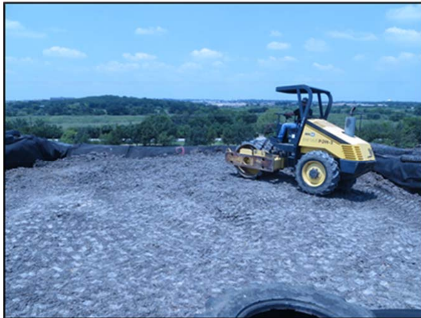
Figure A.244: 1st soil layer compacted by the sheep-footed compactor.
