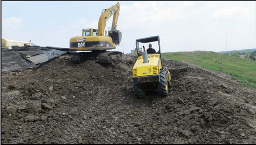
Figure A.247: Compaction of the subgrade by the sheep-footed compactor.
