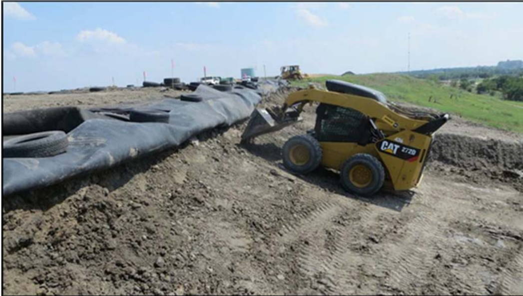
Figure A.252: Middle berm adjustment by a skid steer.
