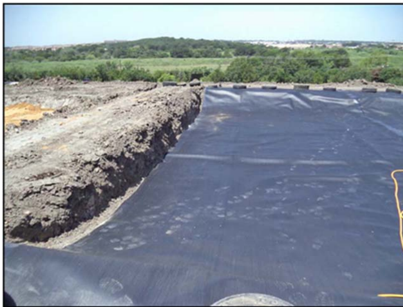
Figure A.97: Geomembrane placed during the thirteenth day.
