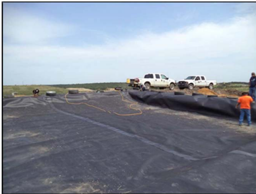
Figure A.104: Middle top section geomembrane details from the Northwest.
