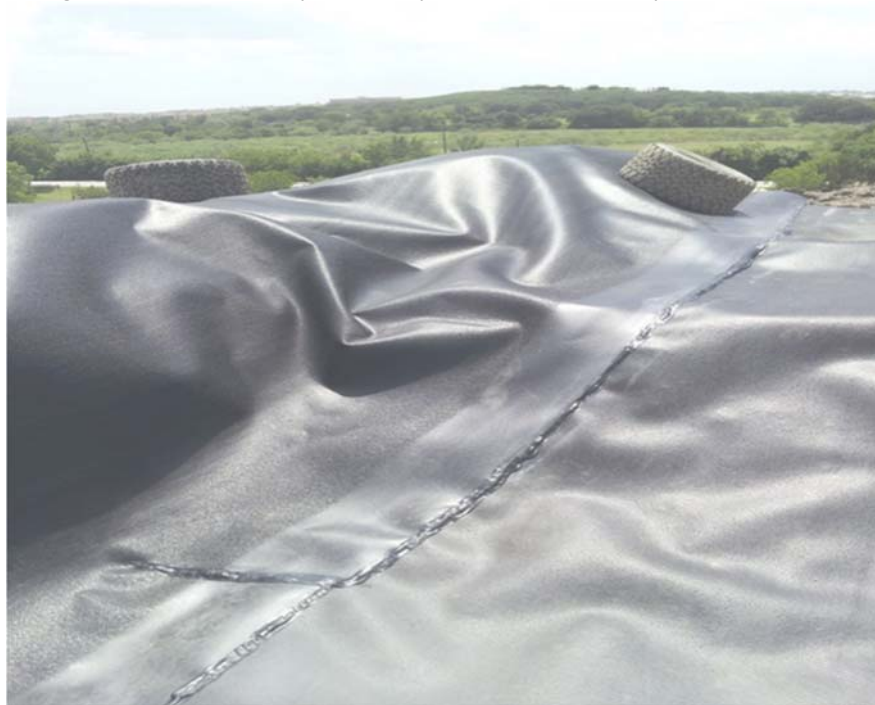
Figure A.123: South Top Section lysimeters (after completion) corner 2.
