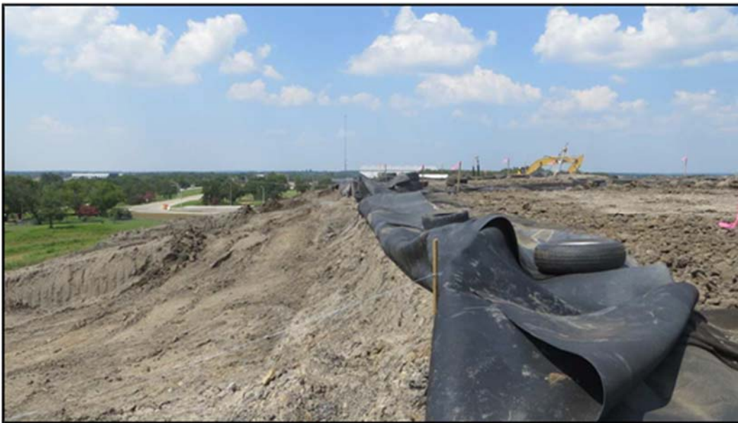
Figure A.251: Geomembrane placement for subgrade and middle berm completion
