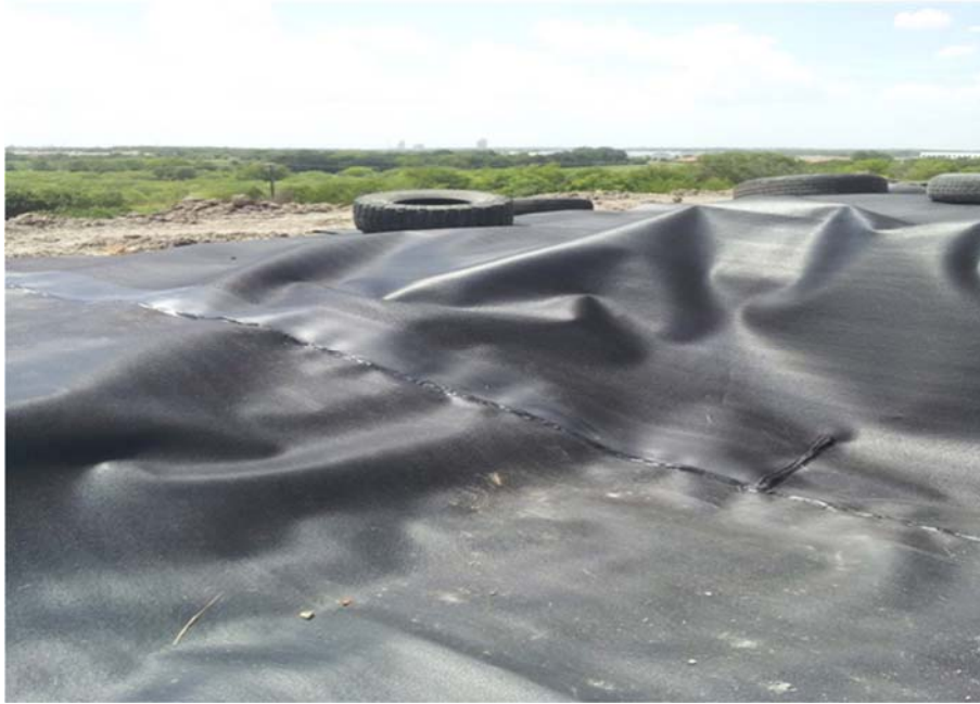
Figure A.122: South Top Section lysimeters (after completion) corner 1.
