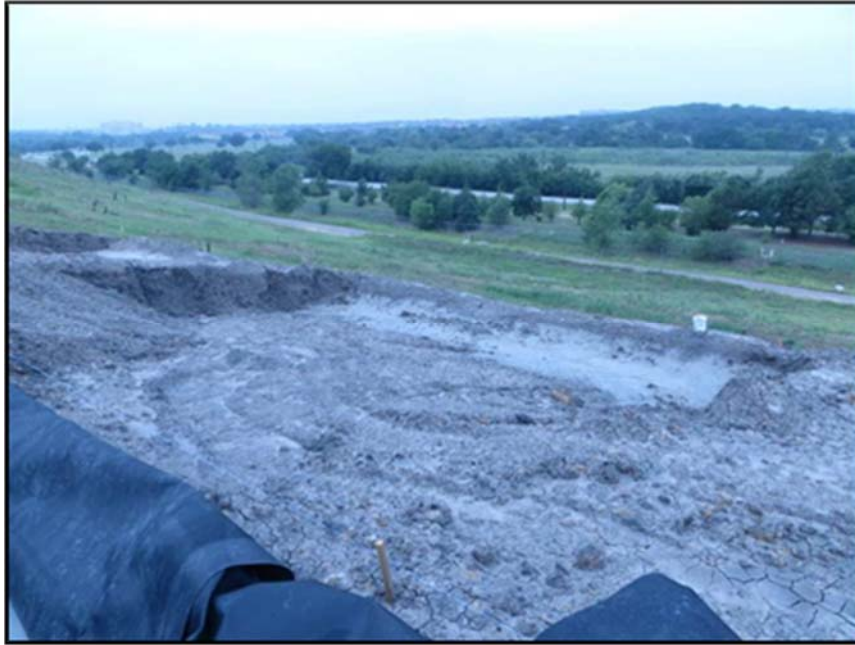
Figure A.217: Middle inclined test section current excavation progress.
