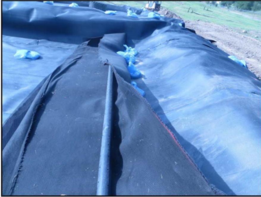
Figure A.287: Sandbag placement for the "burrito wrap."
