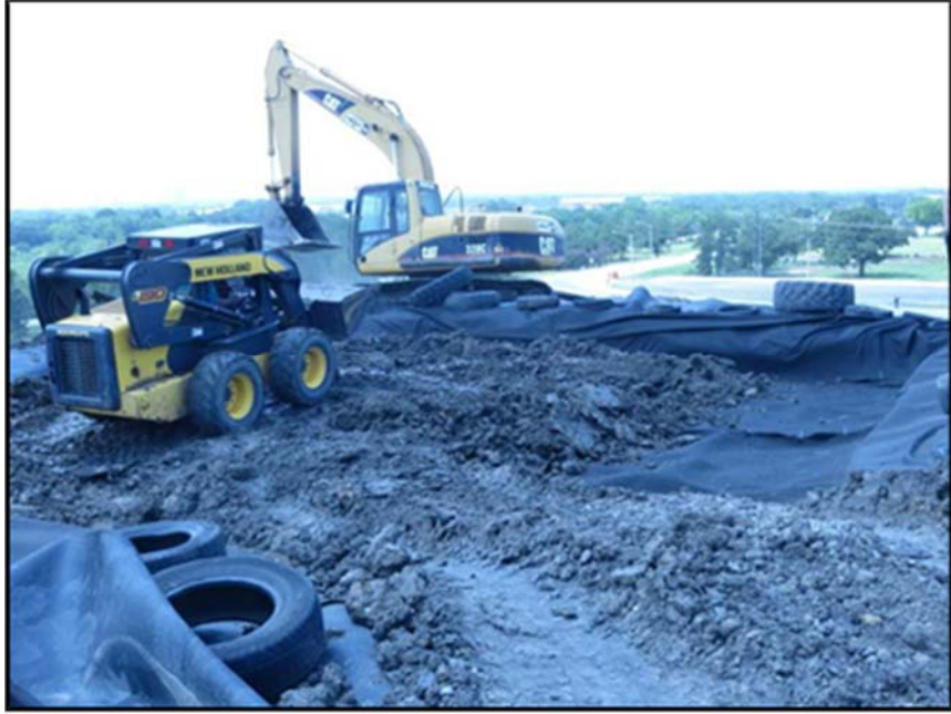
Figure A.225: First soil layer placement on the north top section.
