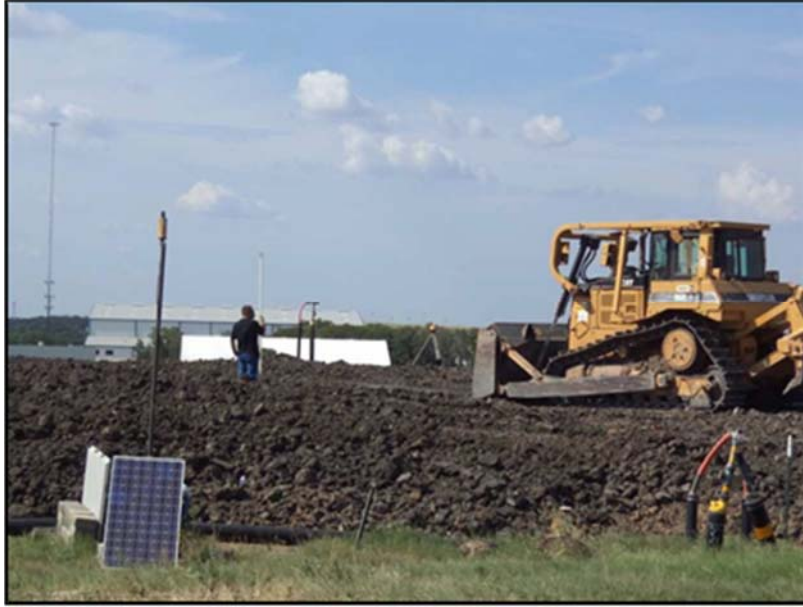
Figure A.22: Embankment height verification one (1).
