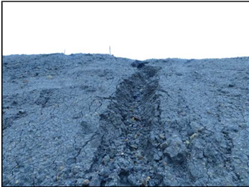
Figure A.220: Drainage gully from the south inclined section.
