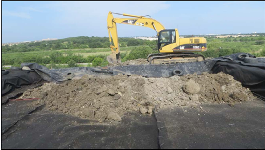
Figure A.152: Excavation of an inclined section and soil placement in the top section lysimeter.
