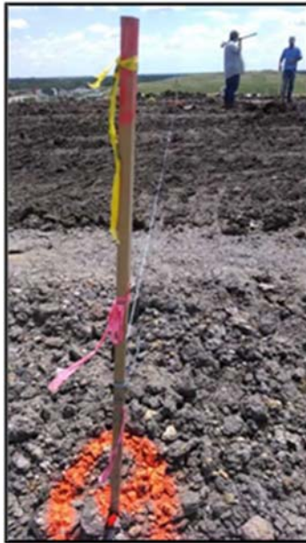
Figure A.44: Staking and marking the edges of the excavation area.
