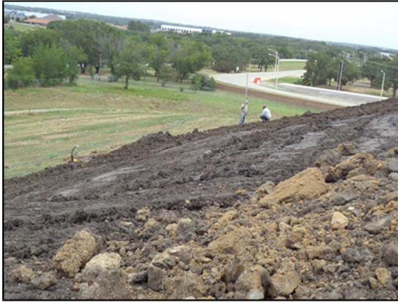
Figure A.32: Embankment height verification.
