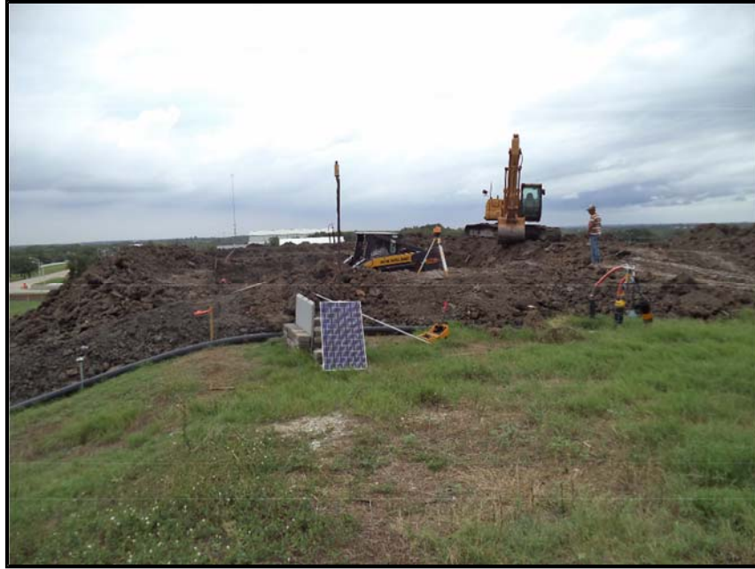
Figure A.61: Construction of the test section on the ninth day.
