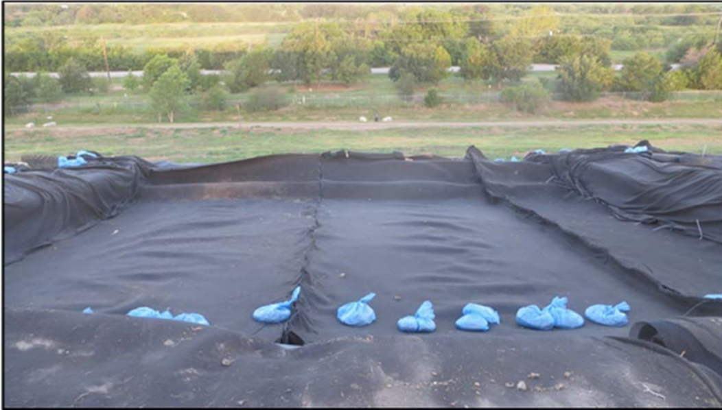
Figure A.302: All of the geosynthetics placed in the middle inclined section.
