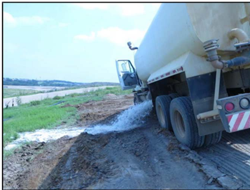
Figure A.241: Removal of water from the water truck to avoid flipping.
