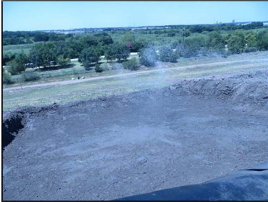
Figure A.277: Water application to the middle inclined section.
