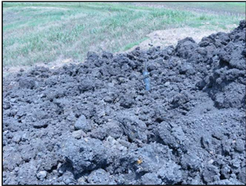
Figure A.233: Percolation pipe outlets.
