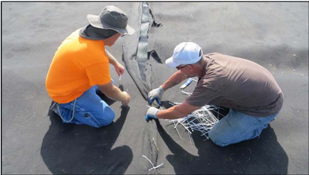
Figure A.139: Joining adjacent geocomposite sheets together with zip-ties.
