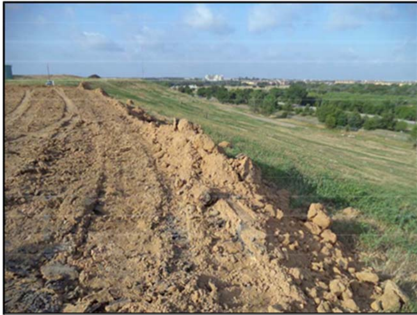
Figure A.1: Top soil stripped and base embankment constructed after day 1.
