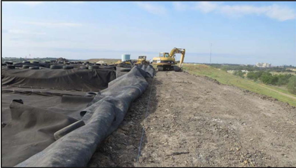
Figure A.151: Folding of the geomembrane and string line placement.
