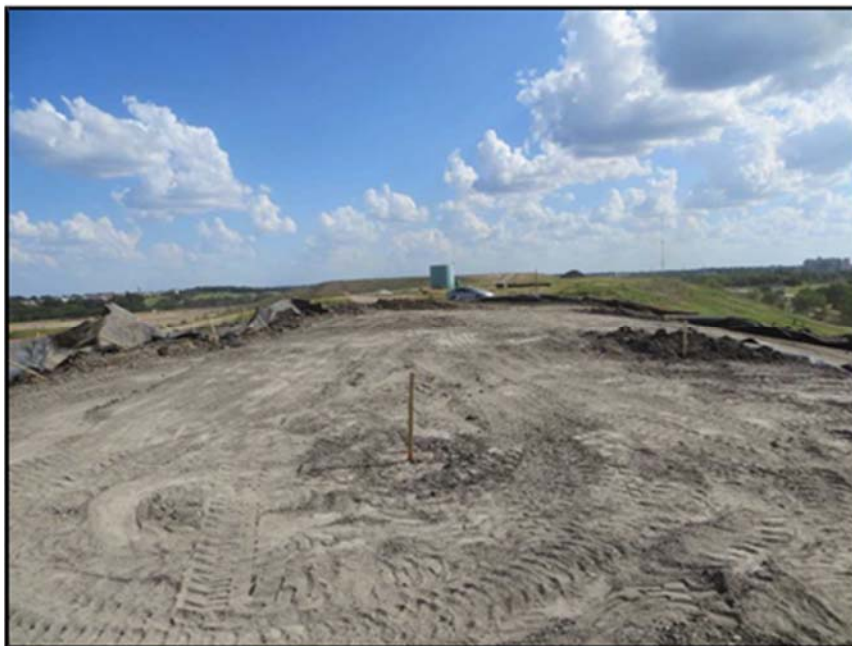
Figure A.356: End of the day details of the top sections.
