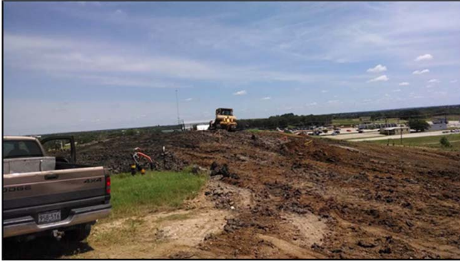
Figure A.43: Embankment modification by bulldozer.
