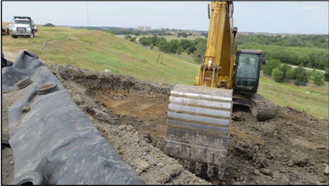
Figure A.153: Excavation of the south inclined section lysimeter-one (1).
