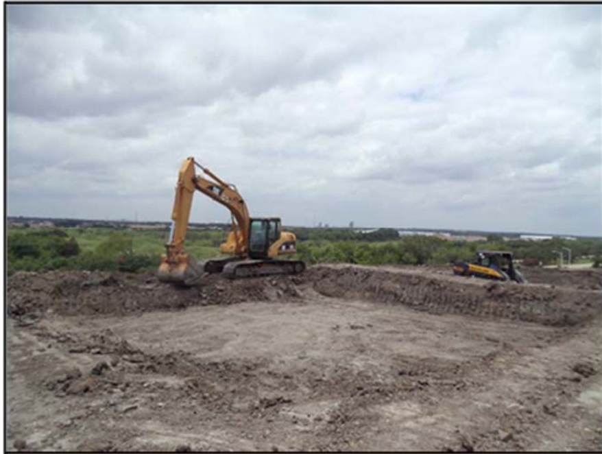
Figure A.72: Construction of the middle berm.
