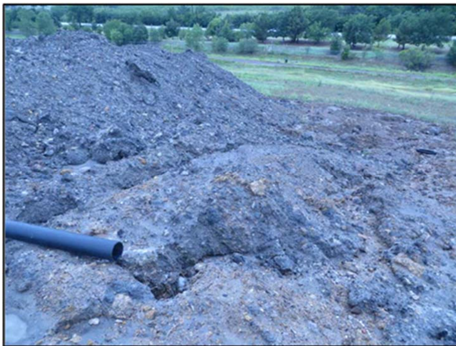
Figure A.194: Pipe details from the north top section lysimeter (no flow seen).
