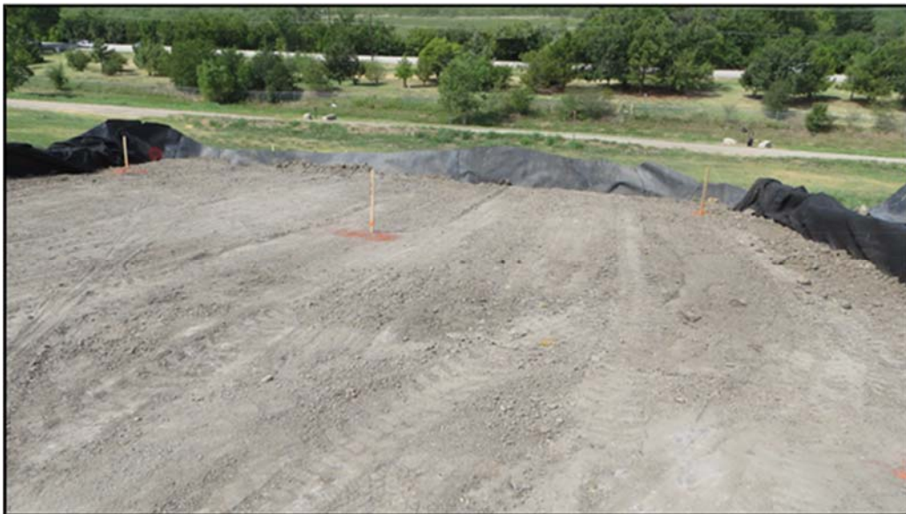
Figure A.359: End of the day details of the south inclined section.
