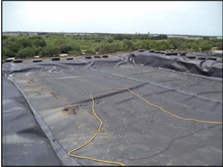
Figure A.105: Middle top section geomembrane details from the Southeast.
