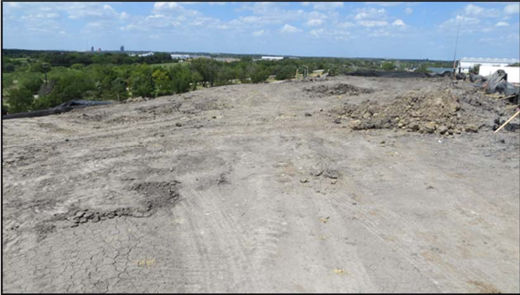
Figure A.339: End of the day details of the top sections.
