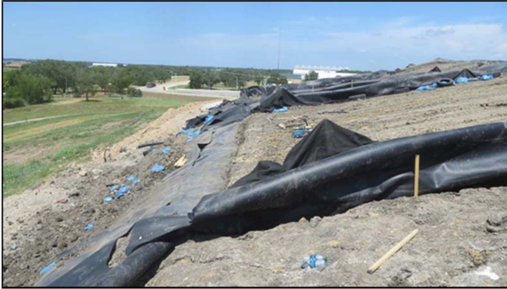
Figure A.334: Soil removal in an inclined section boundary.
