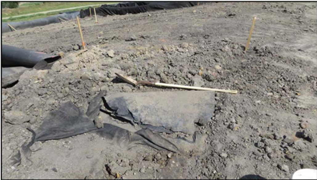
Figure A.350: Cut in the liner between the south and middle top sections.
