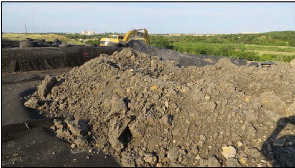
Figure A.170: Details of the soil placed in the middle top section (morning).
