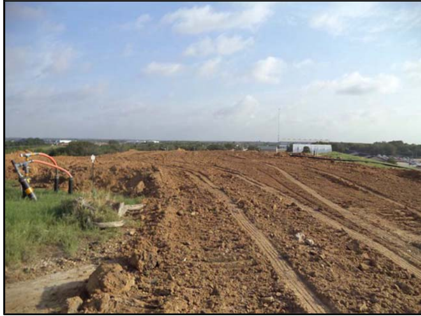
Figure A.2: Embankment base after day 1.
