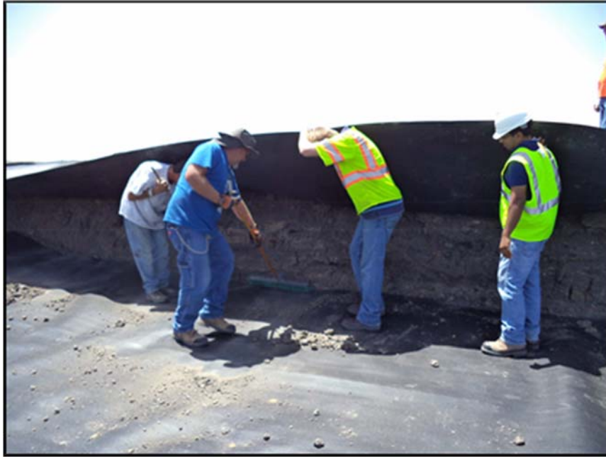
Figure A.88: Sweeping away soil from welding area.
