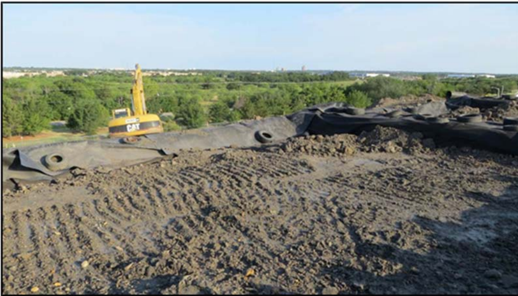
Figure A.168: Details of the soil placed in the south top section (morning).
