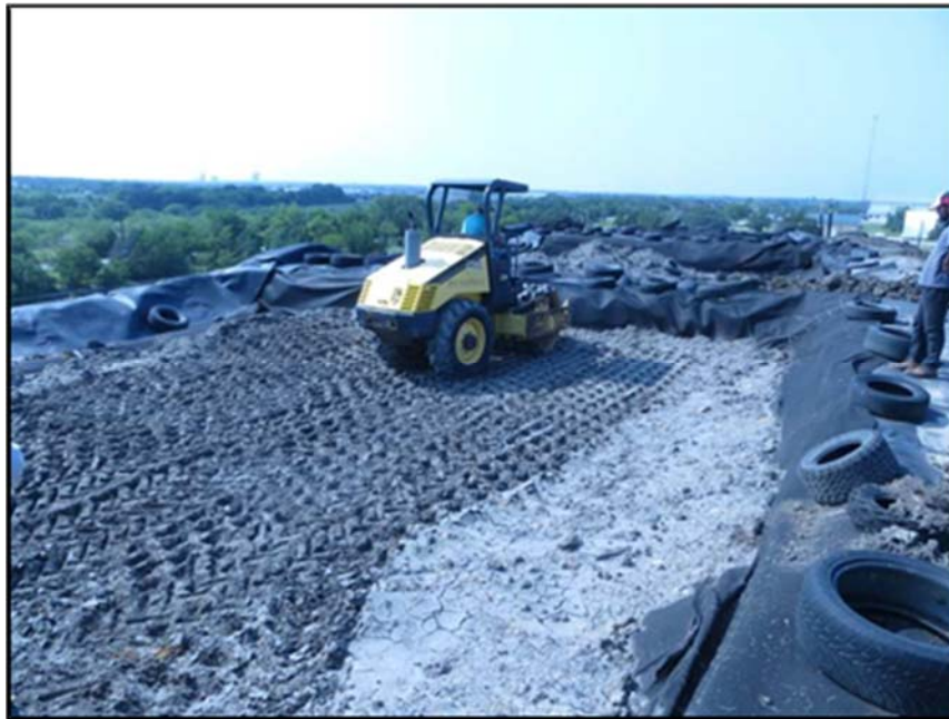
Figure A.227: Sheep-footed compactor on the south top section-two (2).
