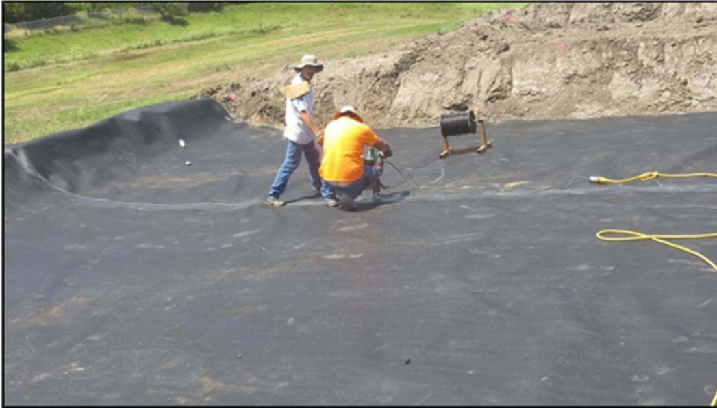
Figure A.269: Welding of the geomembrane in the south inclined section.
