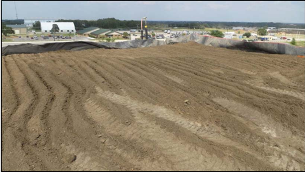
Figure A.369: Topsoil placed in the north top section.
