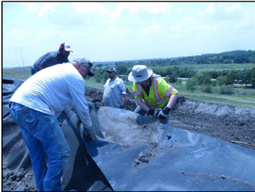
Figure A.235: Pulling over the geosynthetics into the inclined sections.
