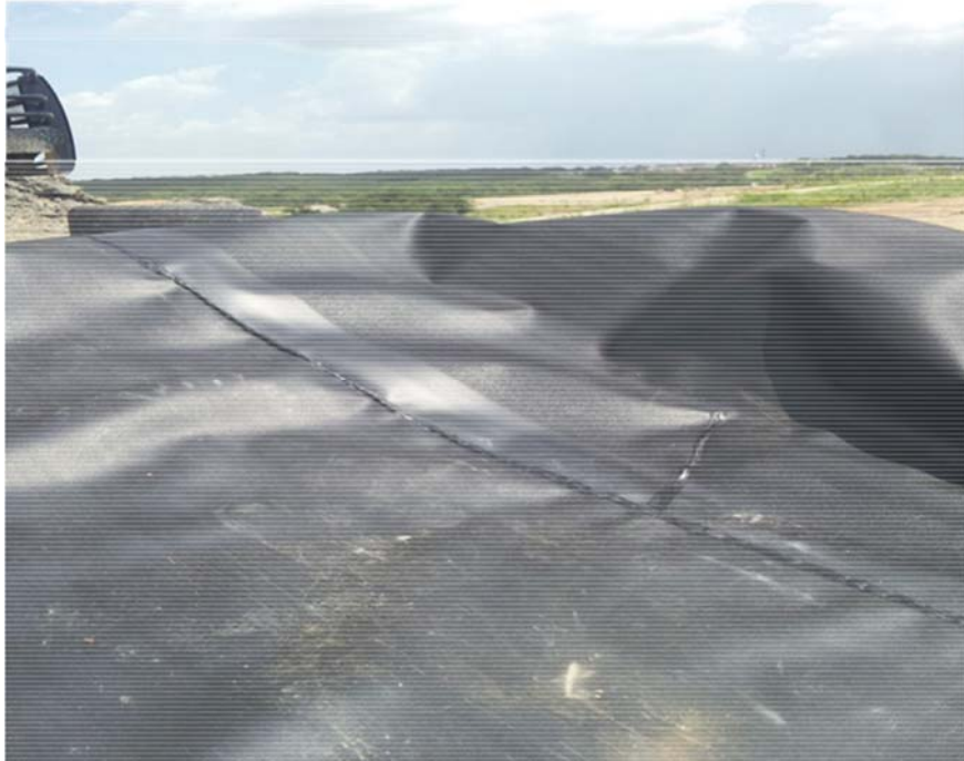
Figure A.124: South Top Section lysimeters (after completion) corner 3
