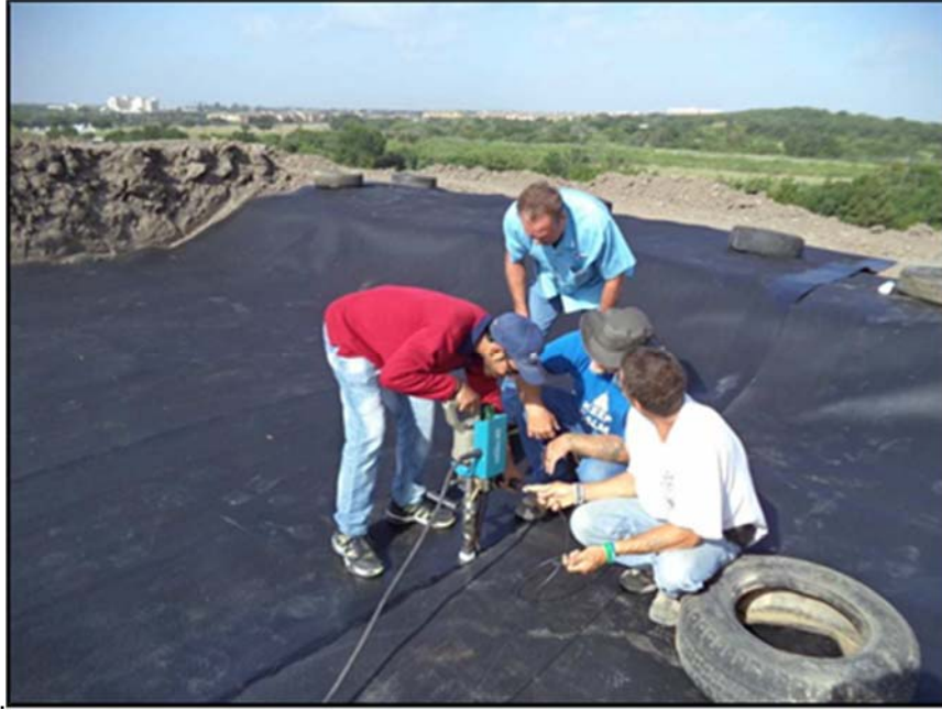
Figure A.82: Welding of the geomembrane by UTA-two (2).
