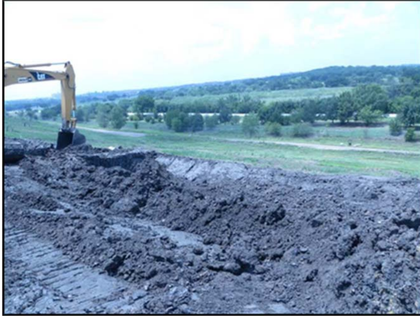
Figure A.228: Reconstruction of the lower berms in the inclined sections.
