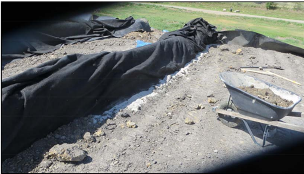
Figure A.338: Placing soil on the sodium bentonite.
