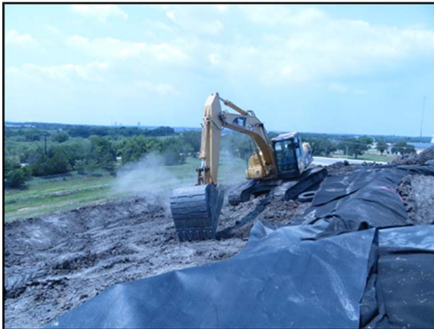
Figure A.246: Modification of the inclined section subgrade by the excavator.
