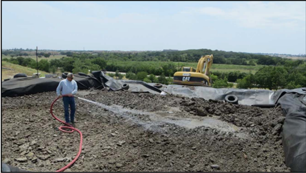
Figure A.160: Water placement on the 1 st layer of the south top section
