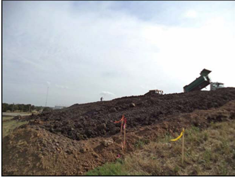
Figure A.28: View of the inclined section from the south.
