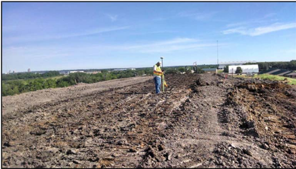
Figure A.40: Surveyor marking the edges of the embankment/lysimeter.
