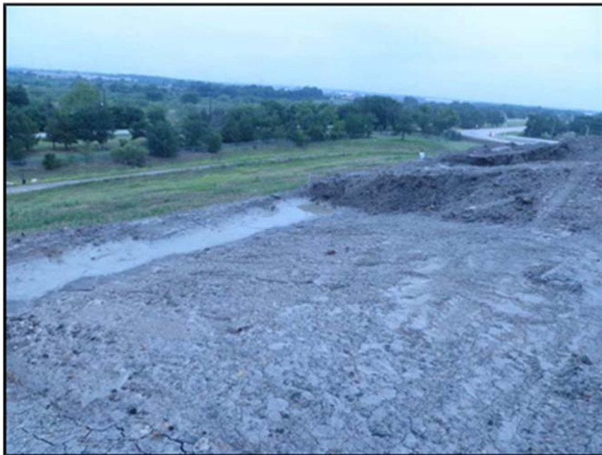
Figure A.218: South inclined test section current excavation progress.
