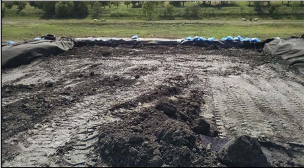
Figure A.310: 1 st soil layer placed in the south inclined section.
