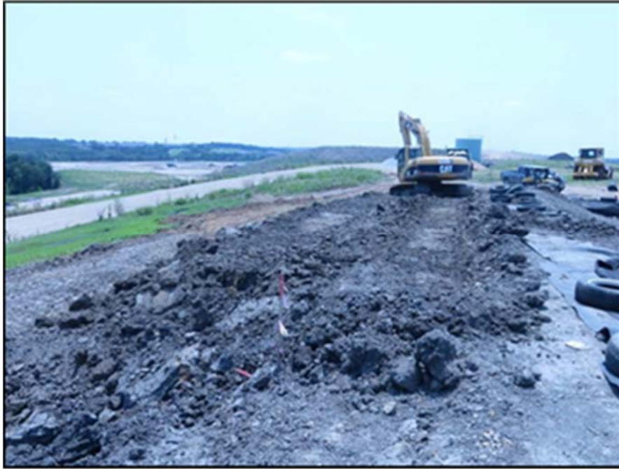
Figure A.243: Roadway construction for the water truck.
