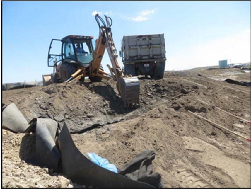
Figure A.379: Removing soil for sidewall construction.
