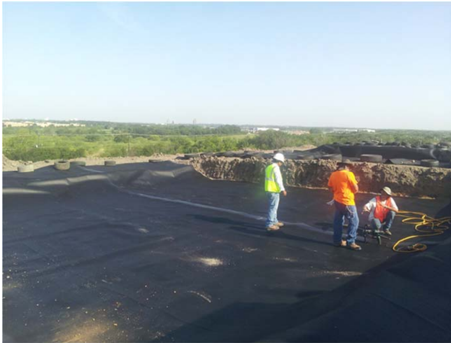
Figure A.118: South Top Section lysimeter (Construction has begun).
