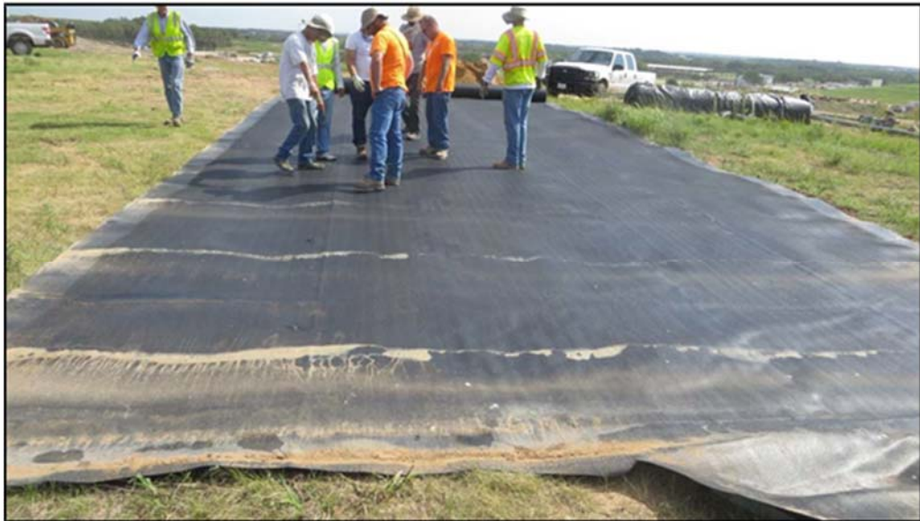
Figure A.268: Checking for holes and imperfections in the geomembrane.
