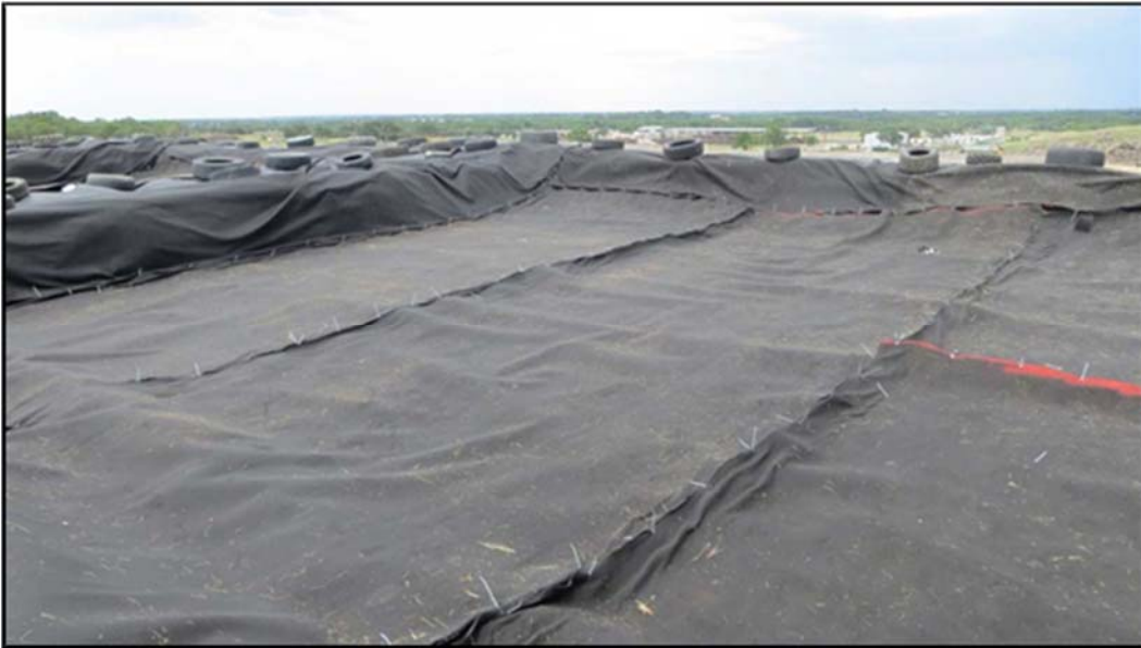
Figure A.145: South top section lysimeter ready for soil placement-one (1).
