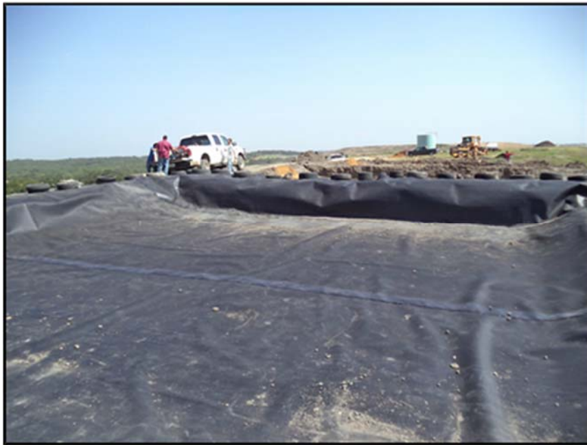
Figure A.93: Geomembrane placed in the North top section lysimeter-three (3).
