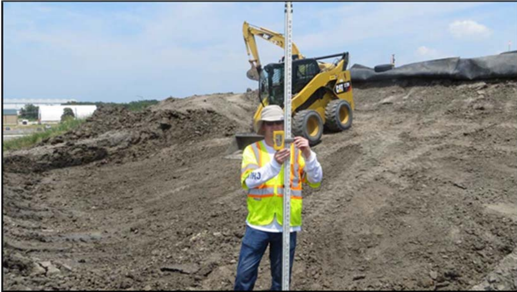
Figure A.258: Slope verification in the bottom of an inclined section by a laser-level.
