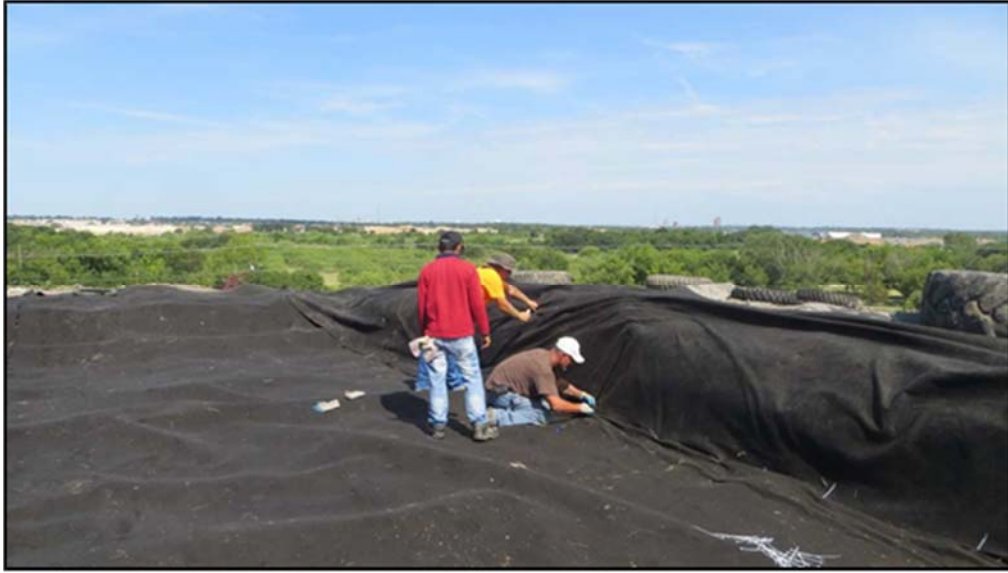
Figure A.142: Placement of the geotextile on the sidewall.
