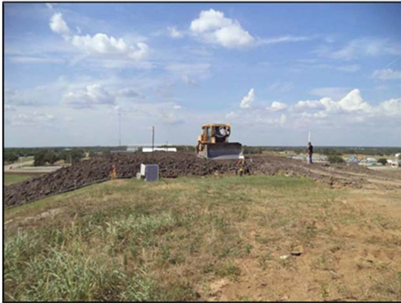
Figure A.23: Embankment height verification two (2).
