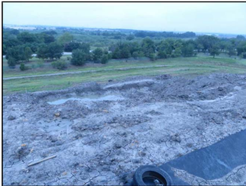
Figure A.216: North inclined test section current excavation progress.
