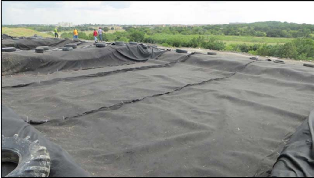
Figure A.150: North top section lysimeter ready for soil placement-two (2).
