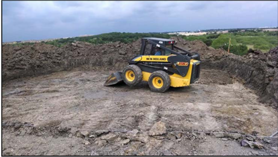
Figure A.49: Finalizing the lysimeter subgrade by a skid-steer.
