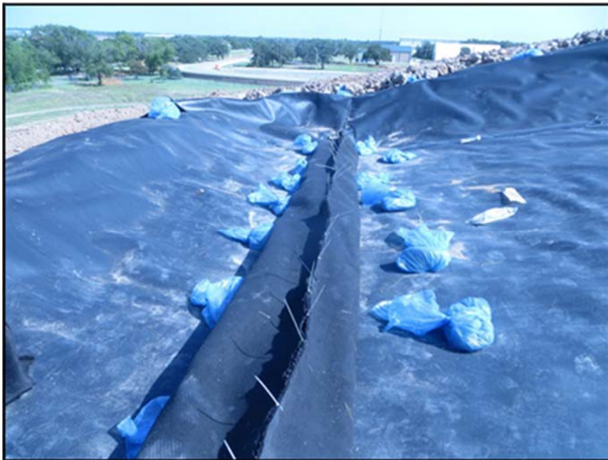
Figure A.294: Completed "burrito wrap" in the north inclined section.
