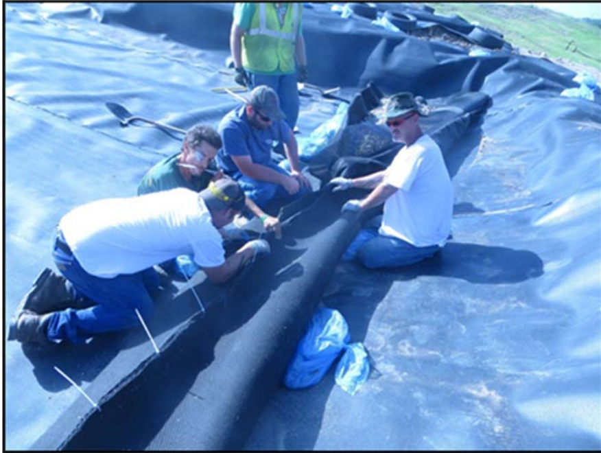
Figure A.293: Placing zip-ties to secure the "burrito wrap."
