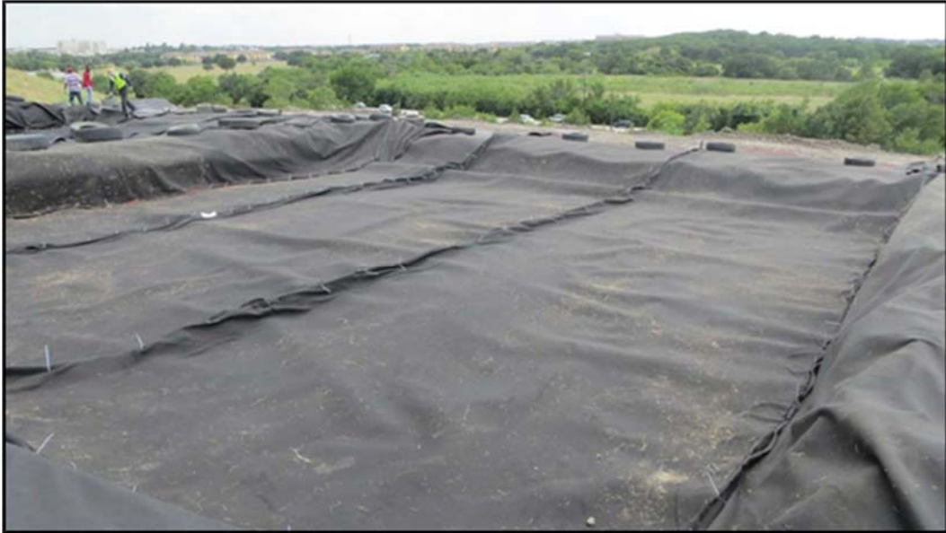
Figure A.148: Middle top section lysimeter ready for soil placement-two (2).
