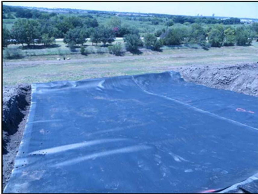
Figure A.278: Geomembrane placement in the middle inclined section.
