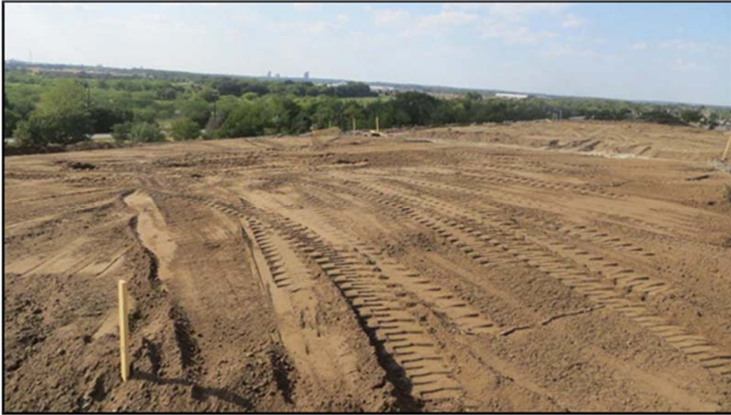
Figure A.374: Topsoil placed in the south top section.
