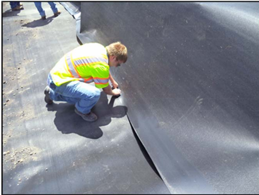
Figure A.89: Cleaning welding area.
