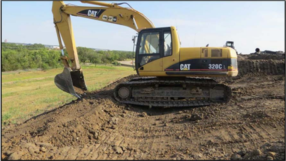
Figure A.165: Lower berm construction with an excavator.
