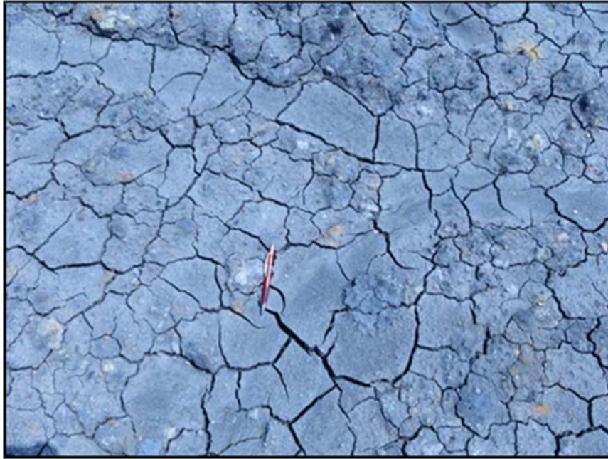
Figure A.213: Desiccation cracks present in the south top test section-two (2).
