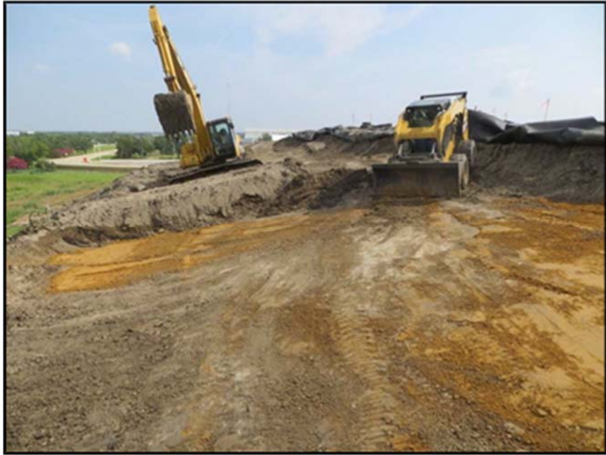
Figure A.255: Subgrade finalization in an inclined section by a skid-steer.
