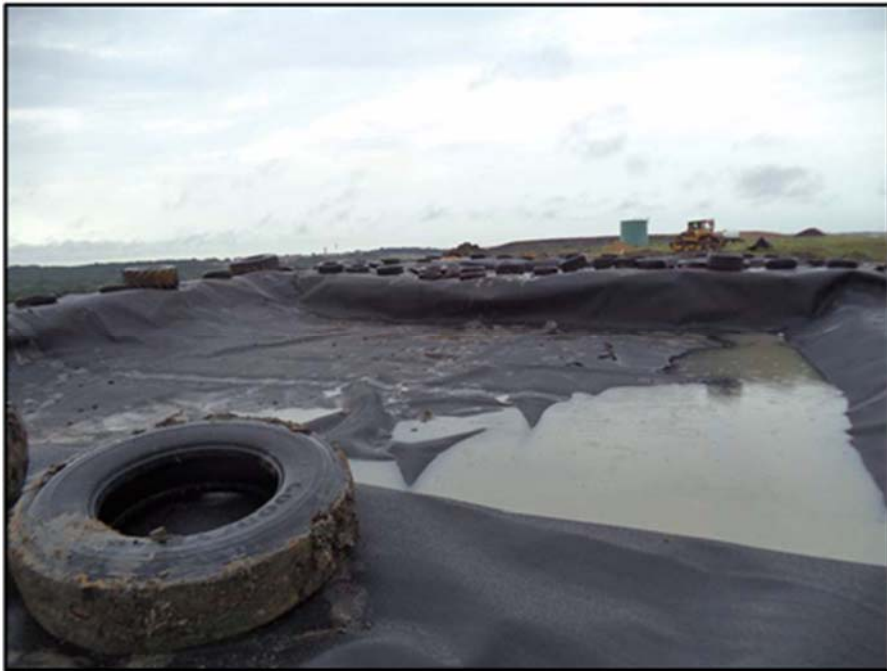
Figure A.110: North Top Section lysimeter after the morning rainfall event(s)-three (3).
