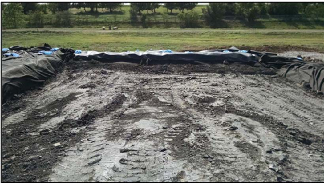
Figure A.311: 1 st soil layer placed in the north inclined section.
