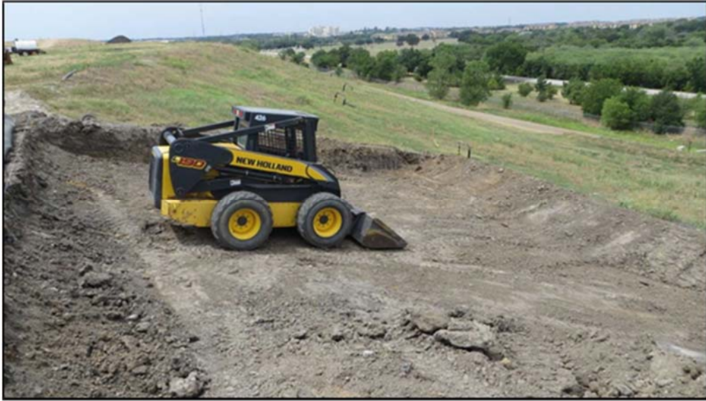
Figure A.167: South inclined test section preparation.
