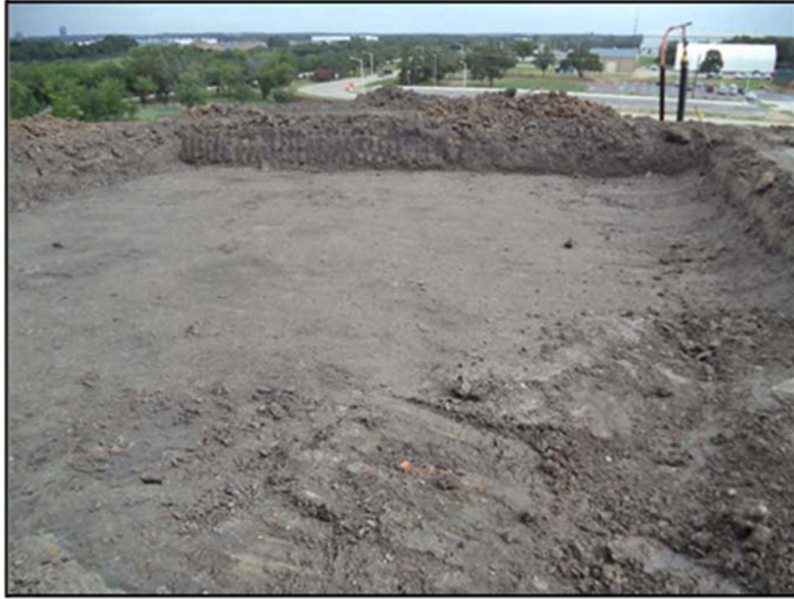
Figure A.74: Subgrade details at the beginning of the eleventh day.
