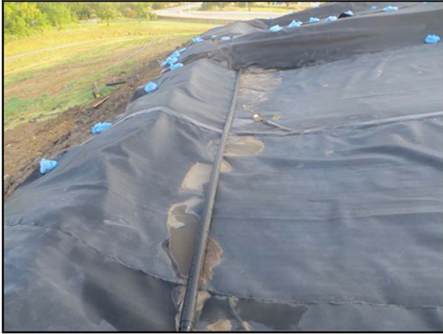
Figure A.291: After rainfall event details of the middle inclined section.
