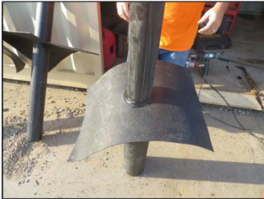
Figure A.275: Results of the welding procedure.
