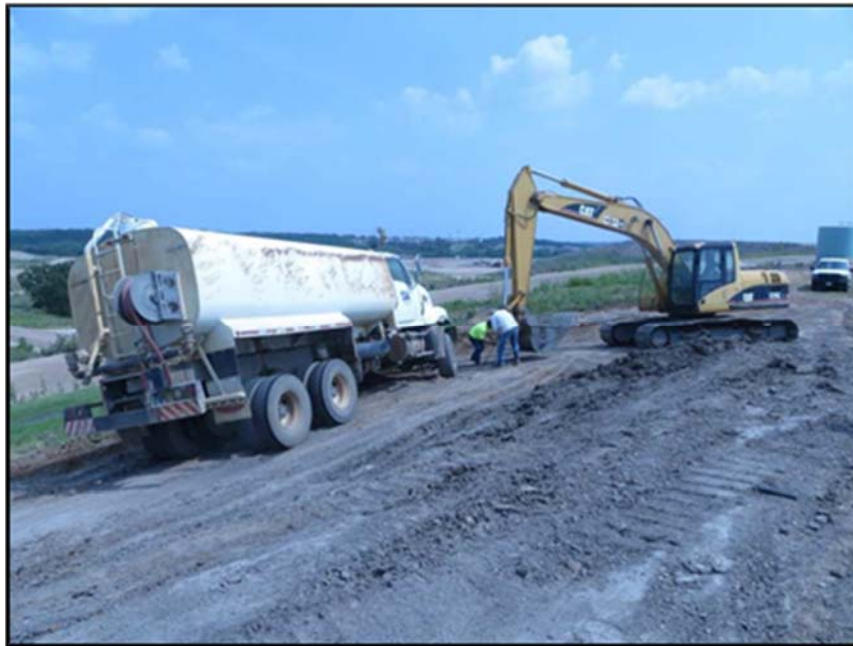
Figure A.242: Excavator used to move the water truck.
