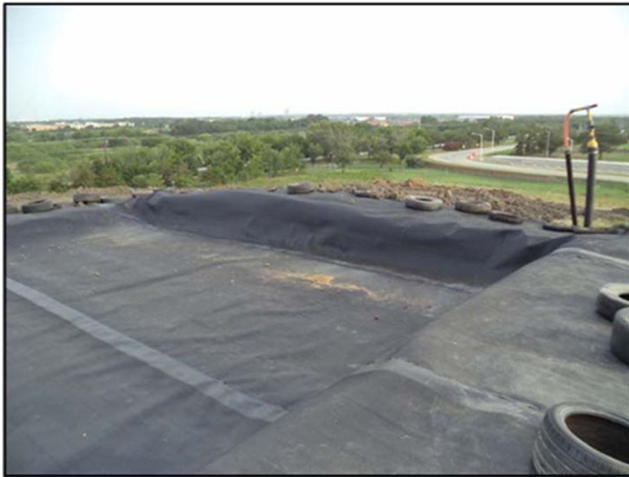
Figure A.99: North top lysimeter geomembrane details-two (2).
