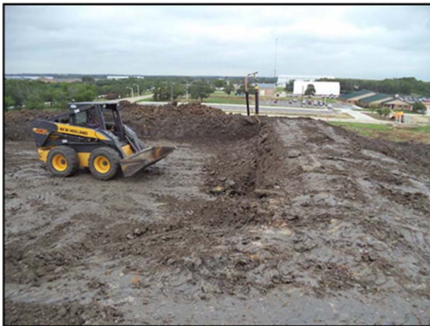
Figure A.64: Berm construction by a skid-steer.
