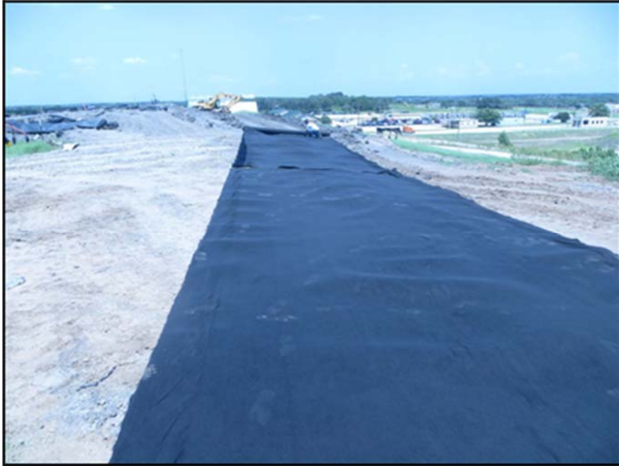
Figure A.297: Cutting the geocomposite drain to appropriate size.
