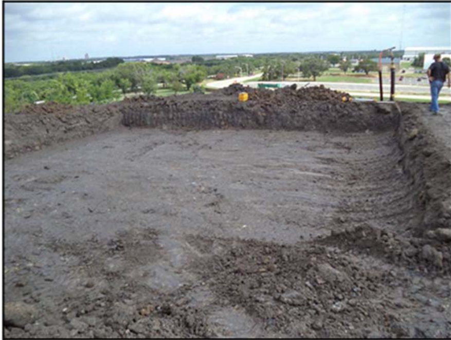
Figure A.63: Nearly completed lysimeter subgrade.
