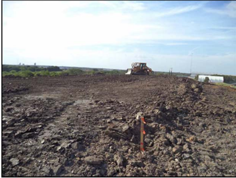
Figure A.20: Top section embankment completion one (1).
