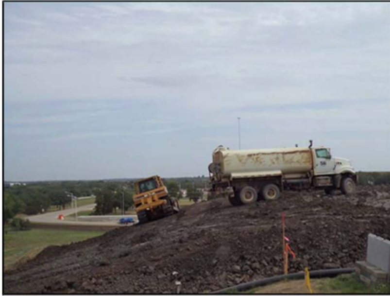
Figure A.30: Inclined section embankment construction one (1).
