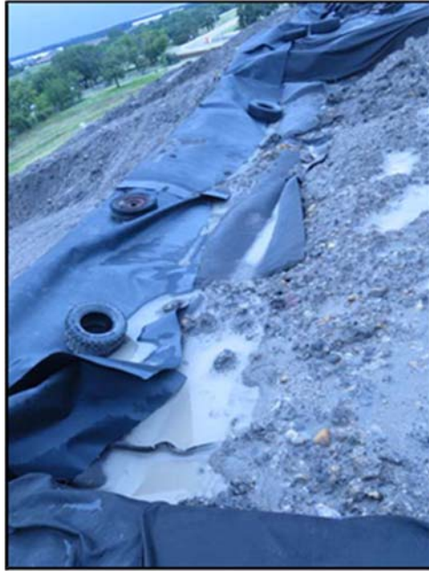
Figure A.200: Details of the middle top section lysimeter (near piping system).
