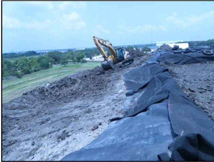
Figure A.234: Geosynthetics pulled over into an inclined section.
