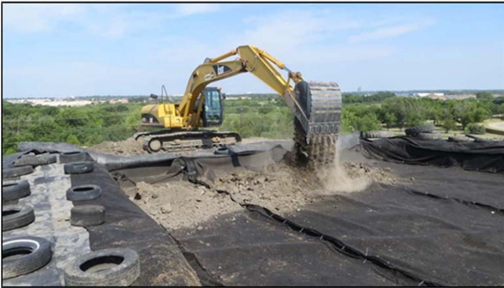
Figure A.172: Soil placement in the north top section.
