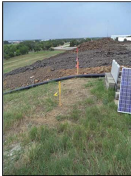
Figure A.15: 10-foot boundary offset stakes placed by the surveyor.
