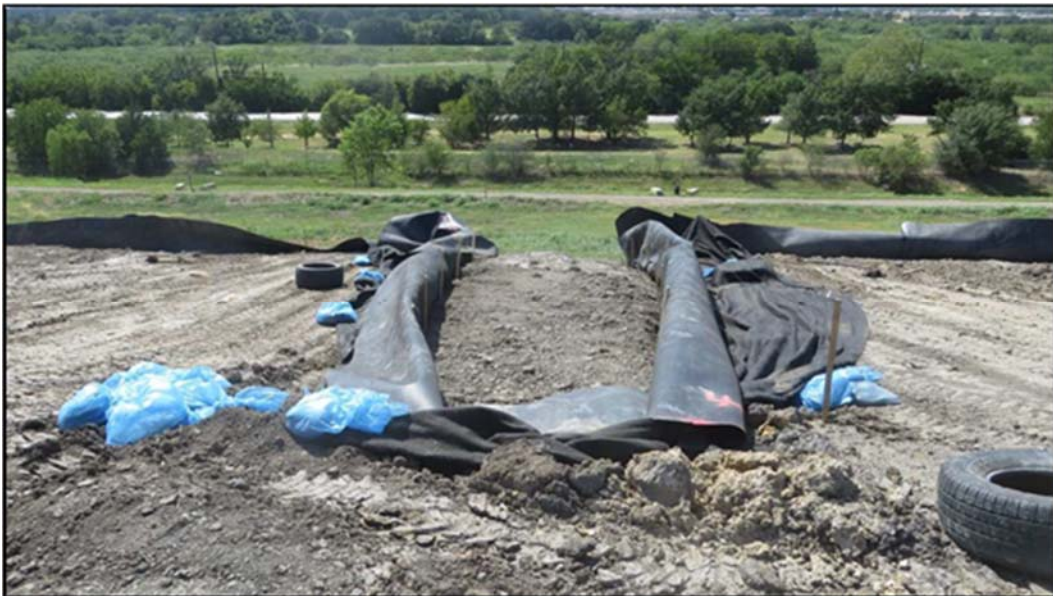
Figure A.333: Topsoil sidewalls placed vertical between inclined sections.
