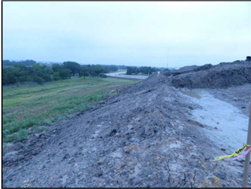
Figure A.219: Embankment below the inclined sections.
