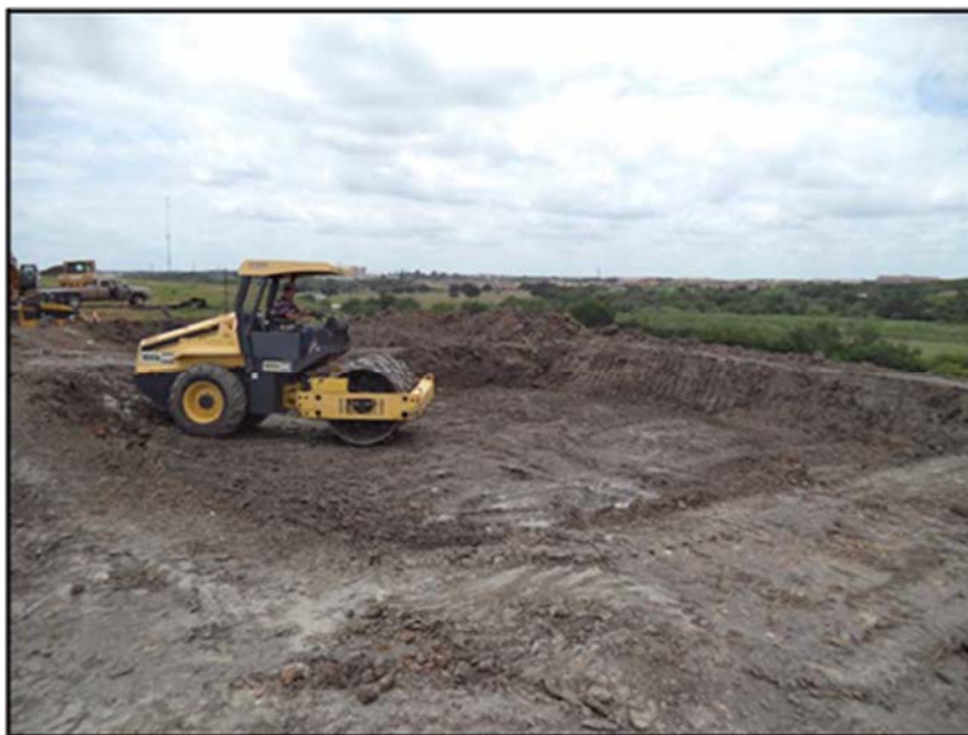
Figure A.67: Subgrade compaction by a sheep-footed compactor.
