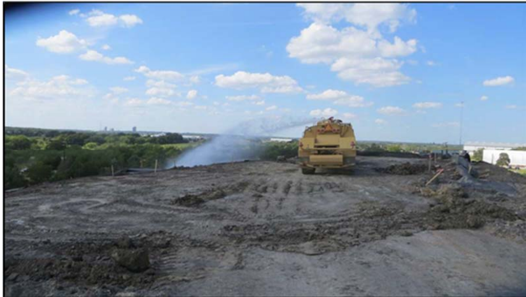
Figure A.345: Applying water to the north inclined section.
