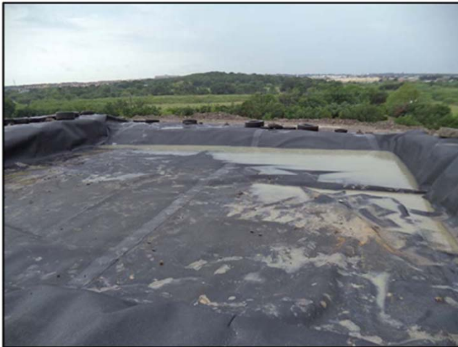
Figure A.108: North Top Section lysimeter after the morning rainfall event(s)-one (1).
