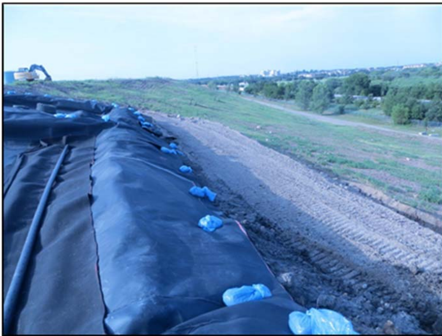
Figure A.288: Roadway constructed below the south and middle inclined sections.
