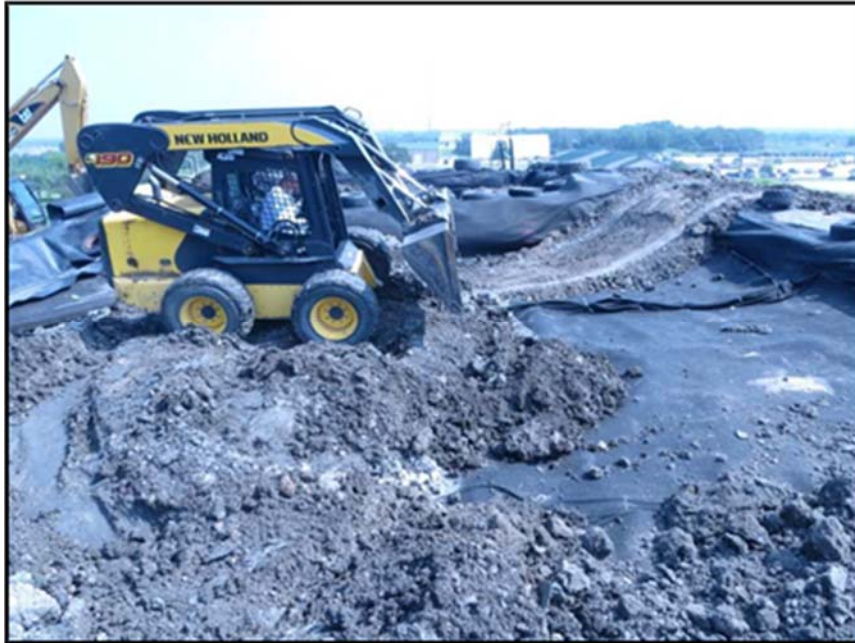
Figure A.229: Skid-steer used to spread the first soil layer.
