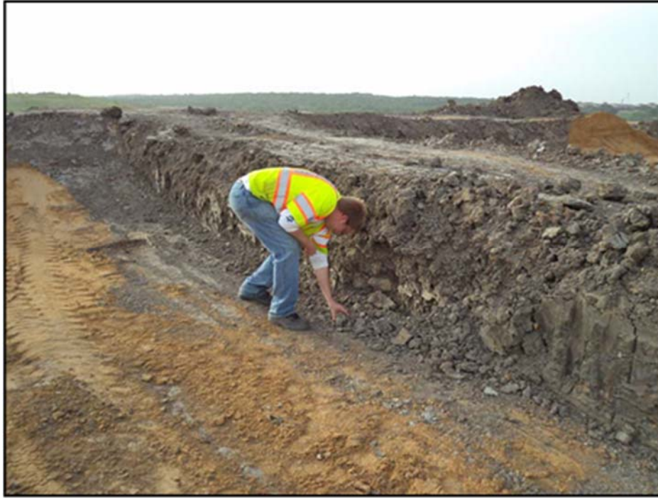
Figure A.94: Removing soil clots and rocks from the subgrade.
