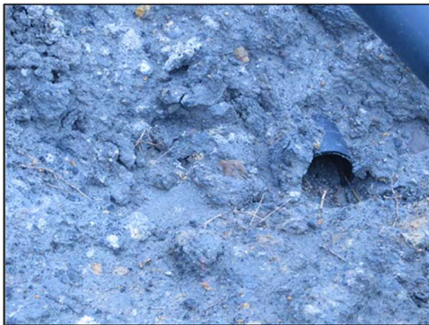
Figure A.195: Pipe details from the middle top section lysimeter (no flow seen).
