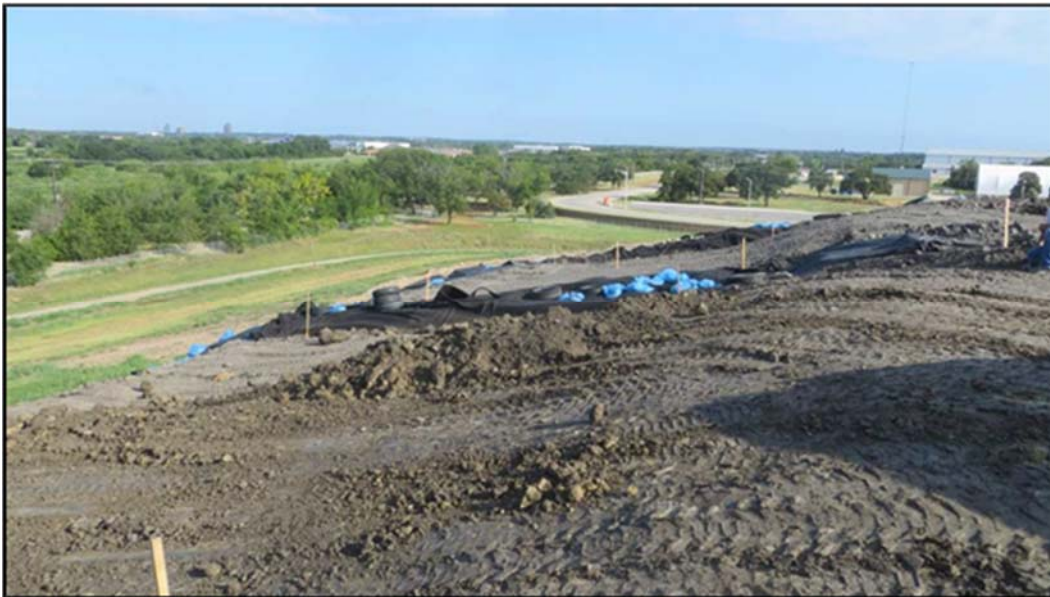
Figure A.330: Stake and soil placement in the inclined sections.
