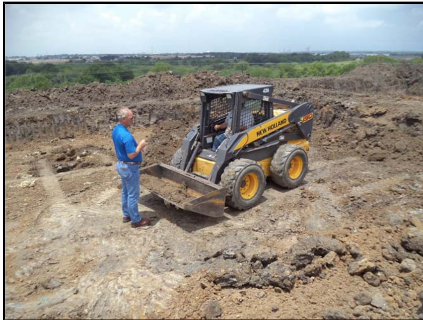
Figure A.62: Mr. Dugger (City of Denton) speaking with the contractors.
