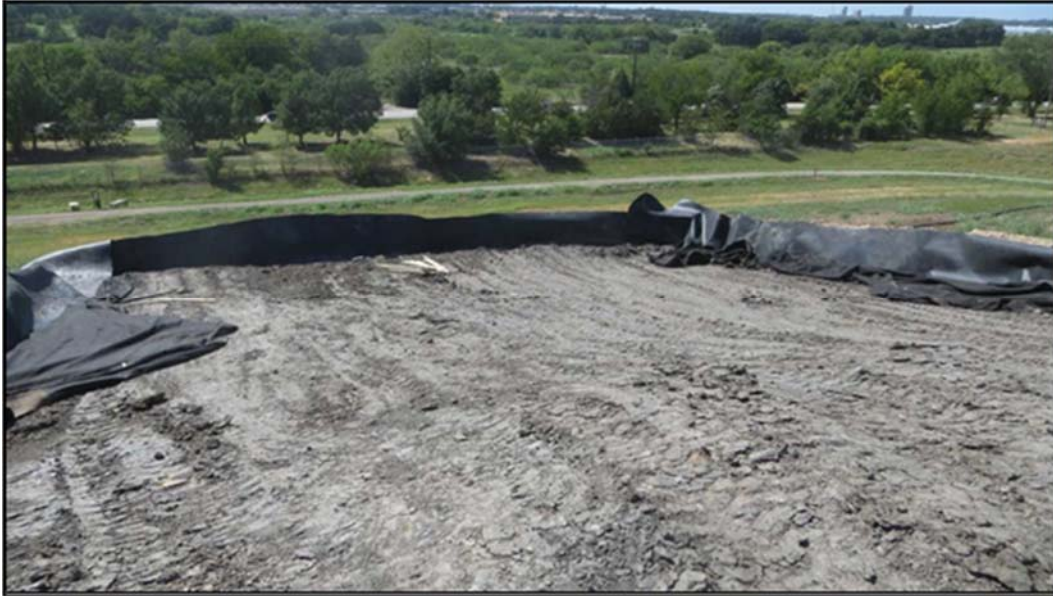
Figure A.332: Topsoil sidewall placement in an inclined section.
