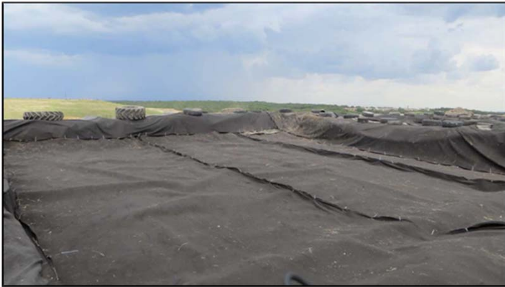
Figure A.149: North top section lysimeter ready for soil placement-one (1).
