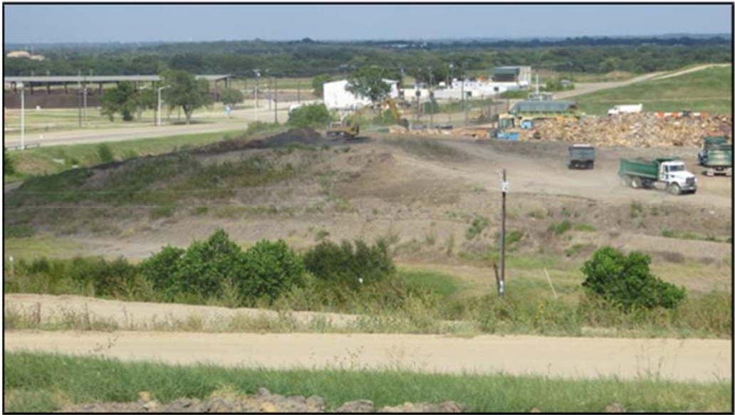
Figure A.324: Location of soil removal from the borrow pit.
