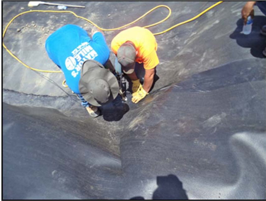
Figure A.90: Geomembrane welding in the Southwest corner.
