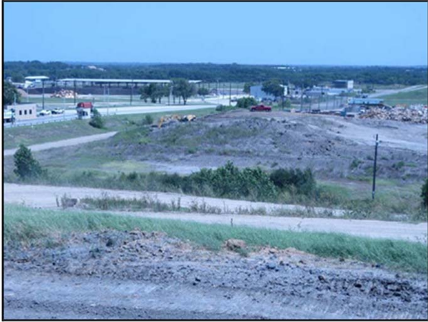
Figure A.313: Obtaining soil from the borrow pit.
