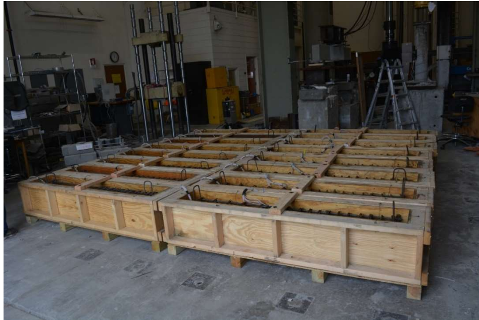
Figure 26 Formworks for large-scale beams
