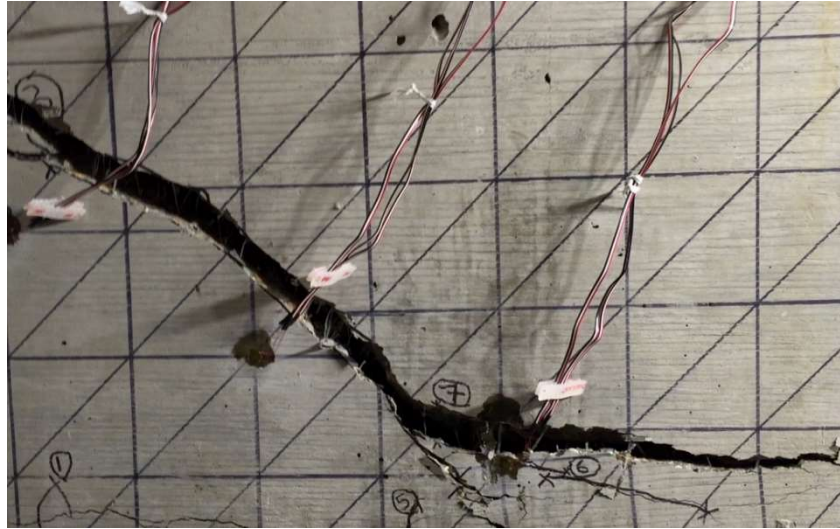
Figure 43 Typical shear crack on a large-scale Beam
