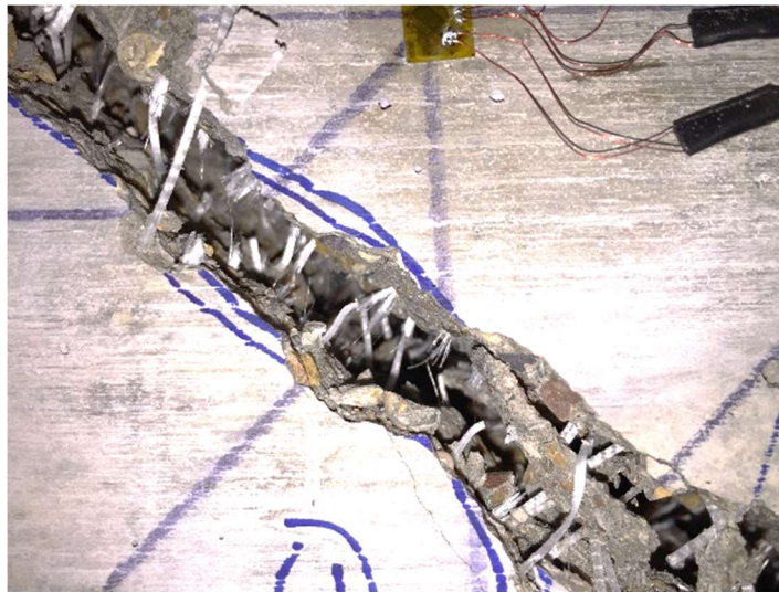
Figure 44 Failure crack widening and pullout resistance of fibers
