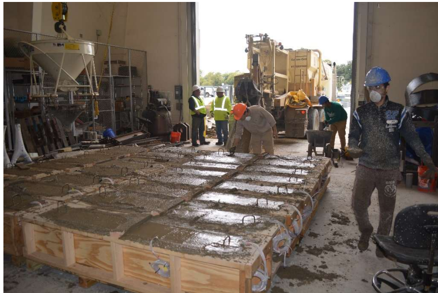
Figure 31 Poured large-scale concrete beams
