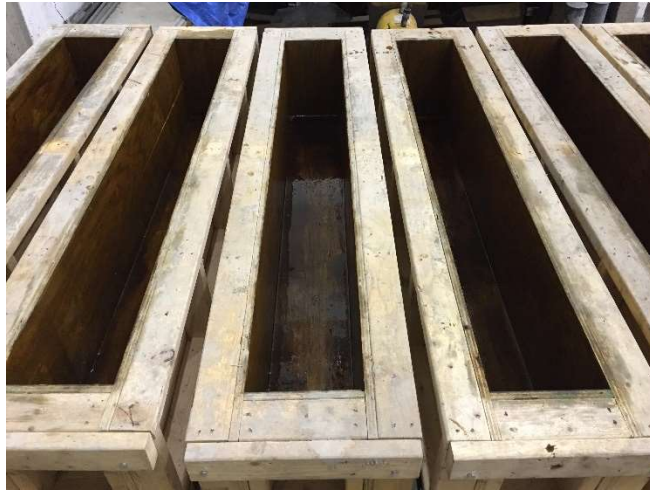
Figure 7 Typical Formwork for large-scale specimens
