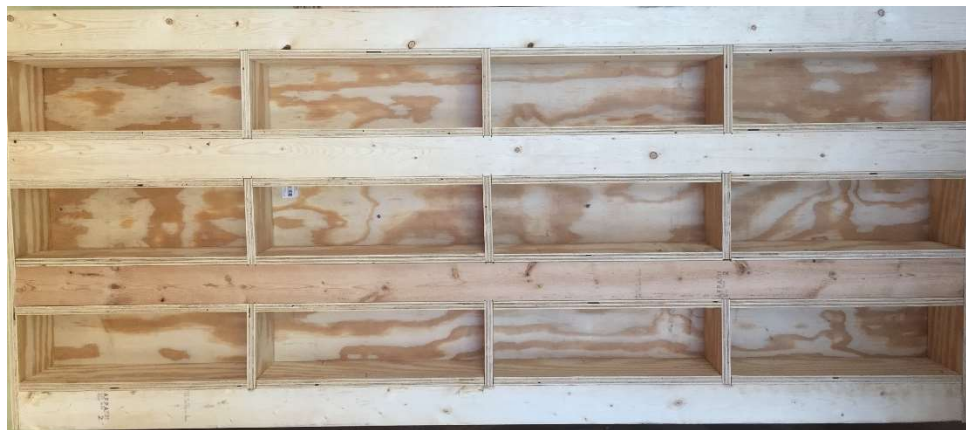
Figure 8 Formwork for Small-Scale Flexure Beams
