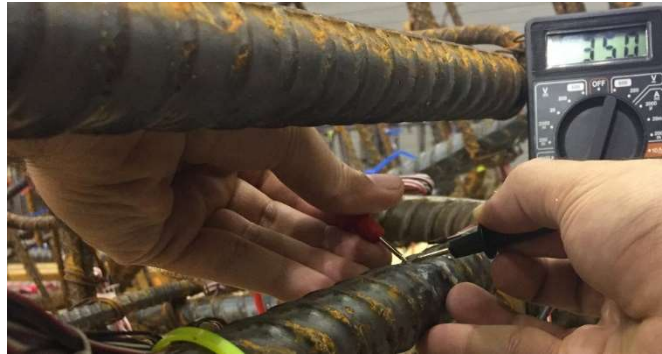
Figure 15 Inspection of an installed steel strain gauge
