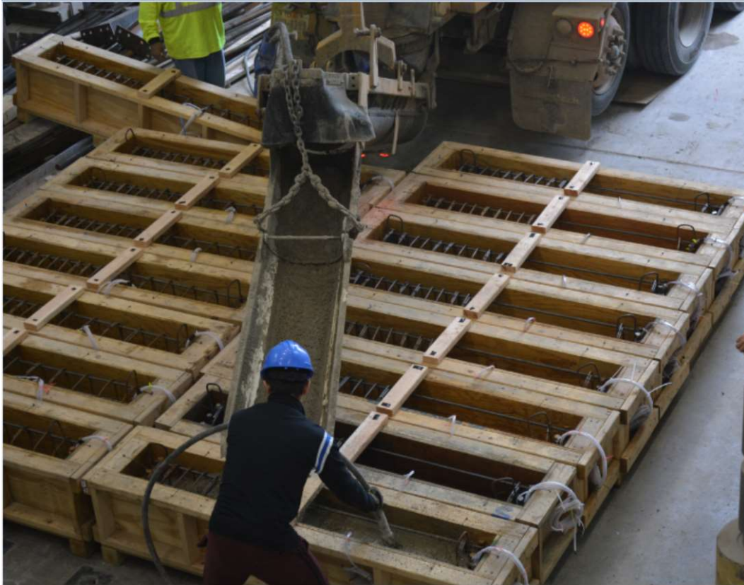
Figure 27 Concrete Pouring and vibrating
