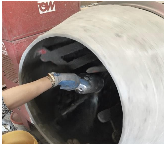
Figure 2.3 - Adding cementations material to the mixer
