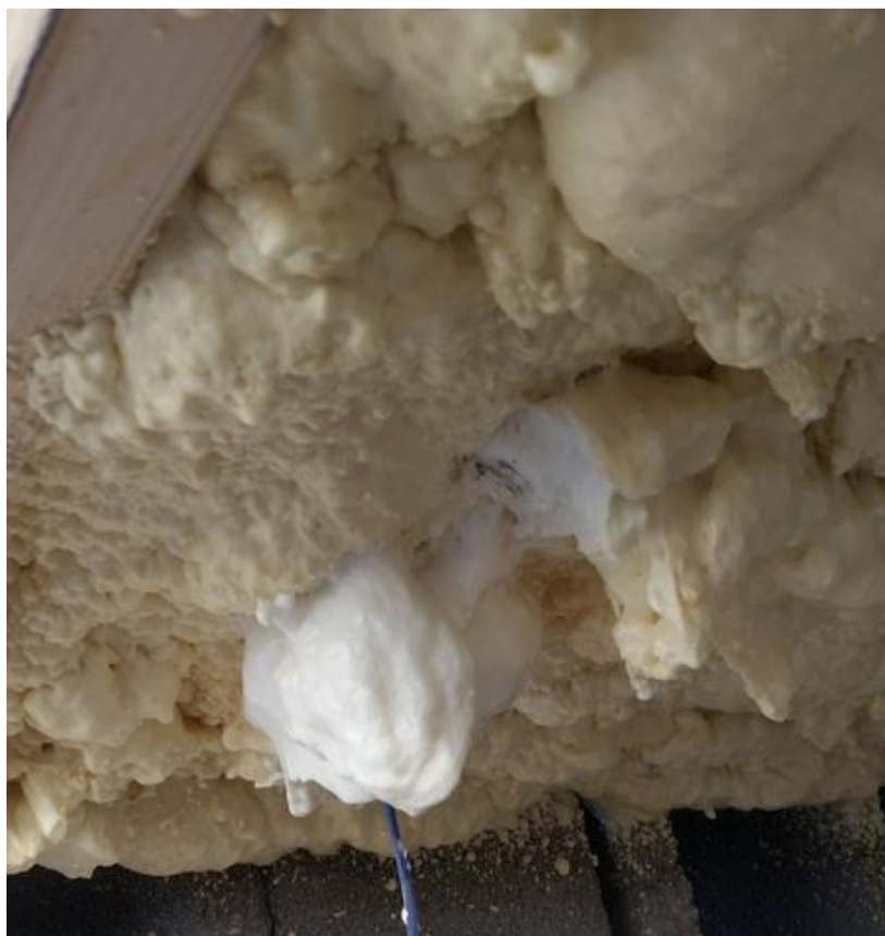
Figure 3.4 Closed cell spray foam application within peripheral wooden framework
