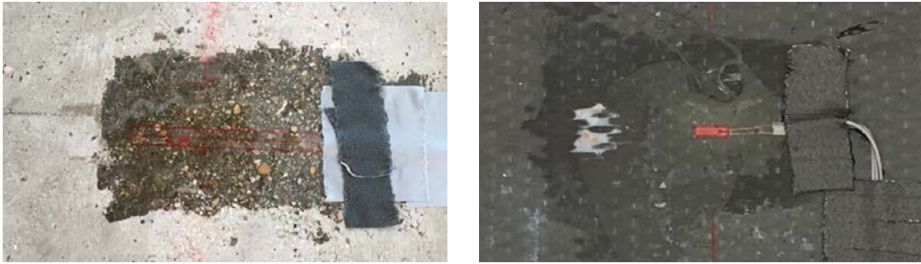
Figure 4-16 Installation of strain gage for concrete (left) and FRP (right)
