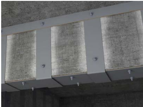
(a) Strengthened RC beam
