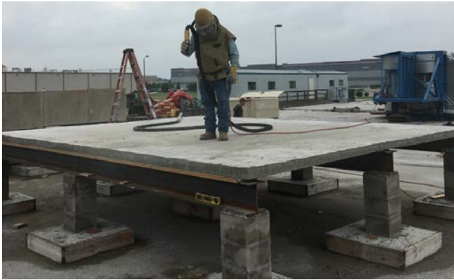
(a) Sandblasting operation
