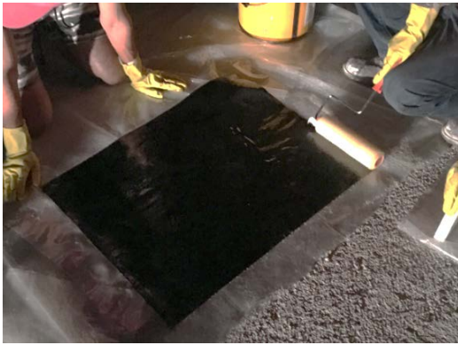
(c) Saturating CFRP with Sikadur 300
