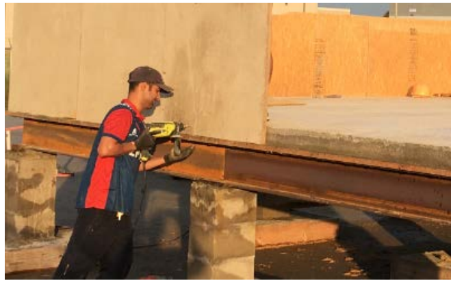
Figure 4-11 Attaching OSB sheathing
