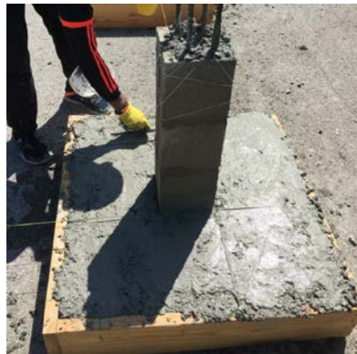
(e) Concrete pouring (f) Concrete finishing
