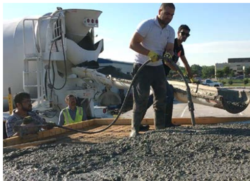
(b) Concrete pouring (left) and concrete vibration (right)
