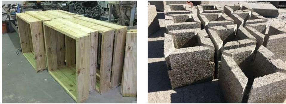
Figure 4-3 Column base formwork (left) and CMU with open corner (right)
