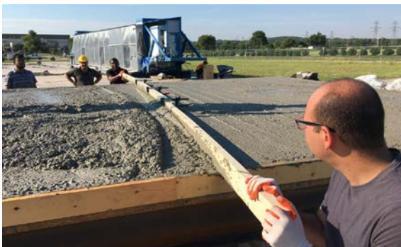
(c) Concrete finishing
