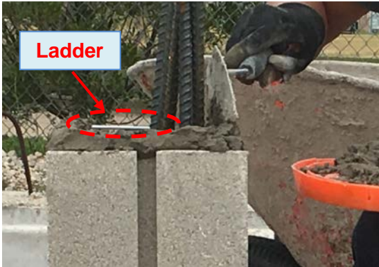
(a) CMU assembly with joist reinforcement (b) Ladder type
