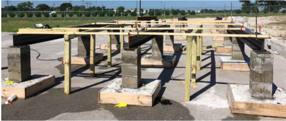
(a) Slab formwork support
