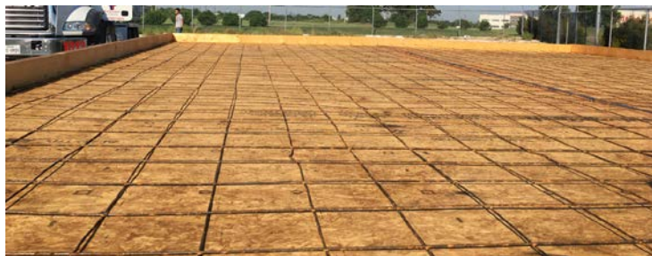
(c) Reinforcement placement
