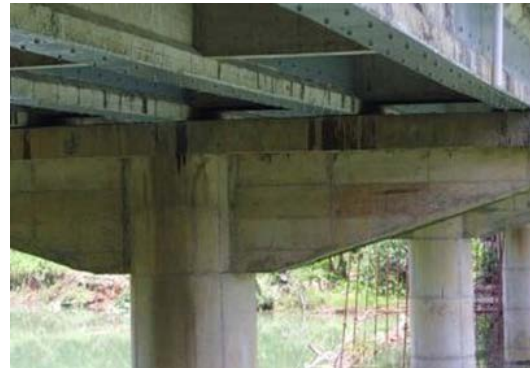
(b) Strengthened bridge girder
