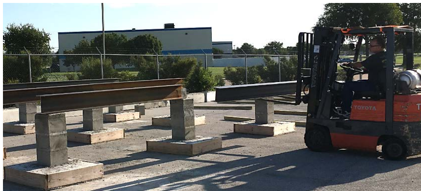
Figure 4-6 Steel beam placement
