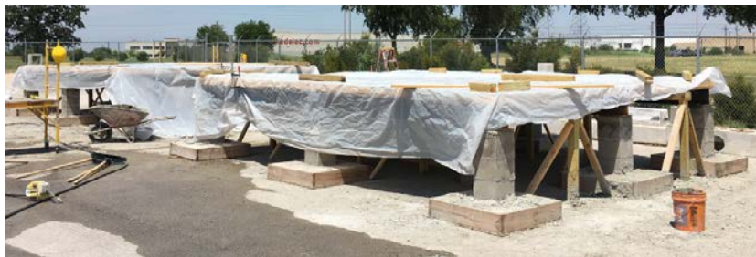
Figure 4-9 Curing concrete slabs
