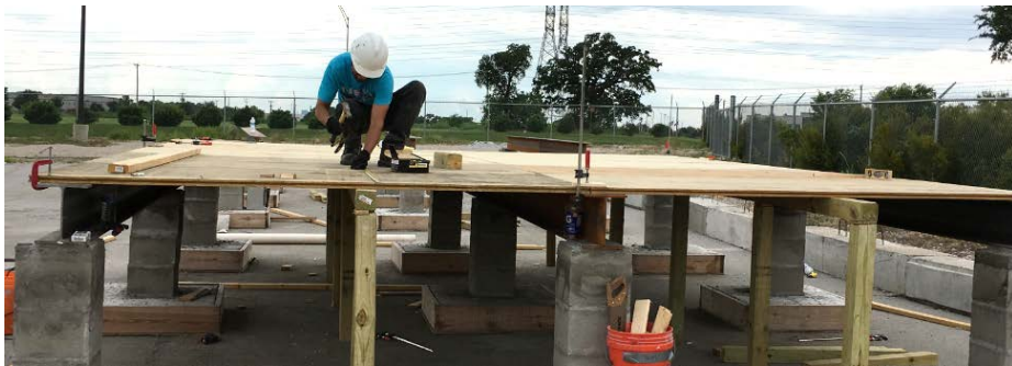
(b) Slab formwork
