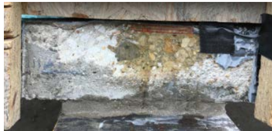
(c) Side surface at the middle support beam
