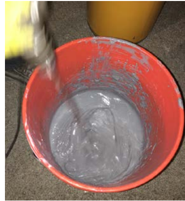
(b) Mixing of Sikadur 330
