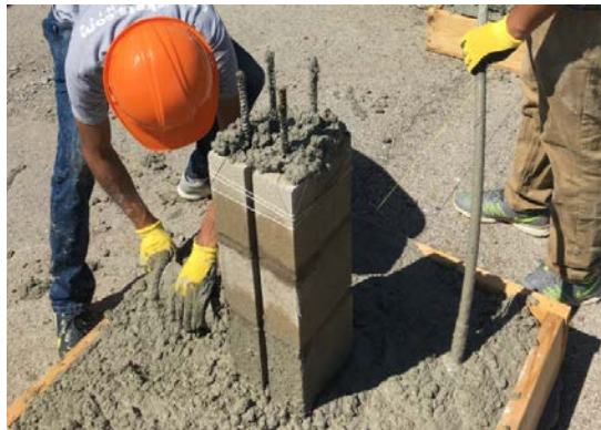
(e) Concrete pouring (f) Concrete finishing
