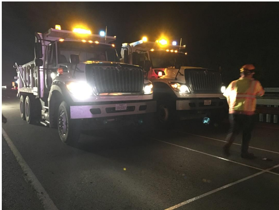
Figure 4-11 Trucks stopped at Bent cap 37
