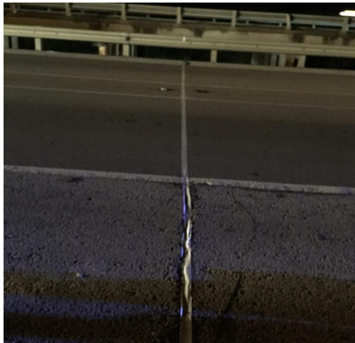
Figure 4-6 Marking the roadway
