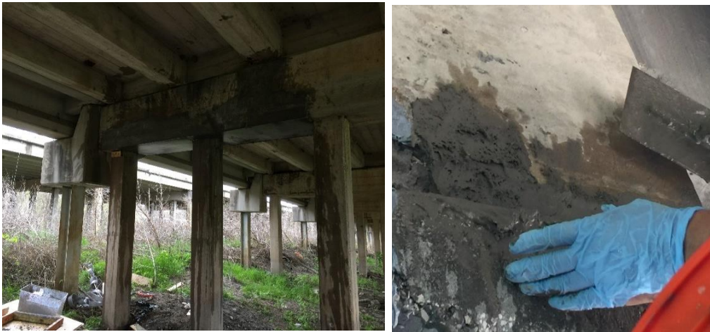
Figure 3-9 Patching mortar application
