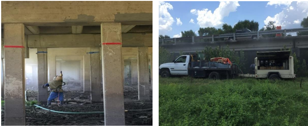
Figure 3-10 Sandblasting the repaired area
