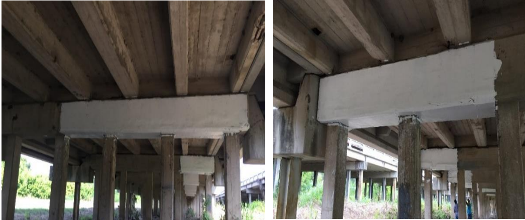
Figure 3-12 Protection top coat application
