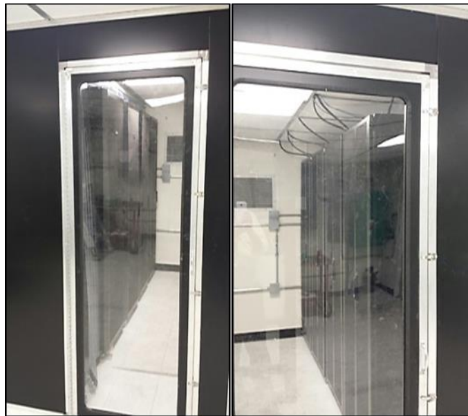
Figure 3-5 Experimental IT Pod Showing the Cold and Hot Aisles
