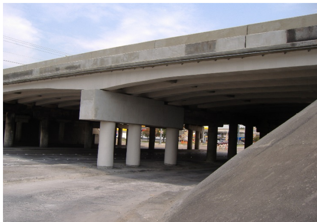
Figure 3-7 Post- repair MacArthur Bridge
