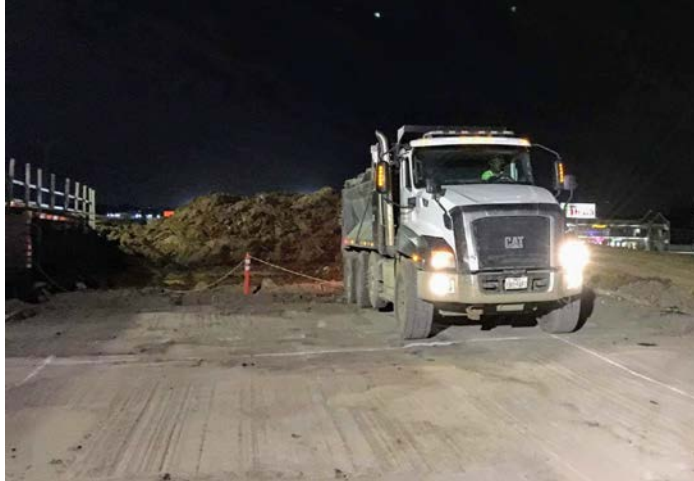
Figure 4-8 Truck in position for load test
