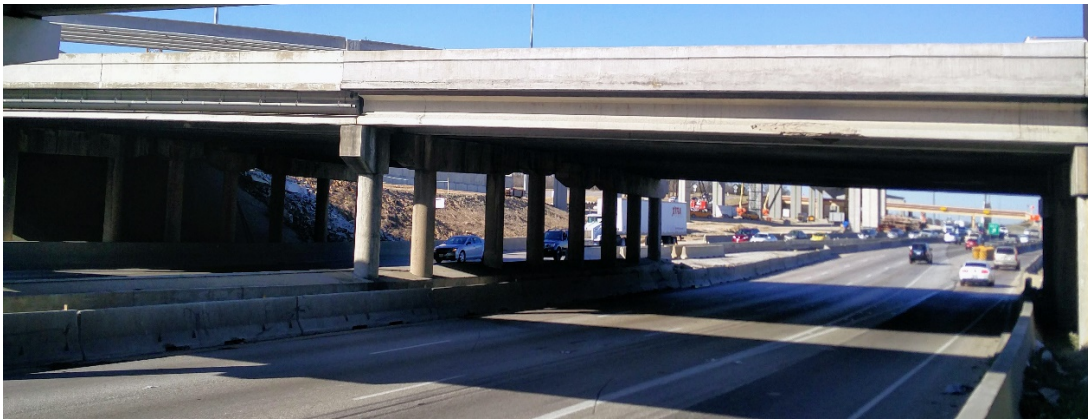
Figure 3-9 Loop 12 Bridge Side view
