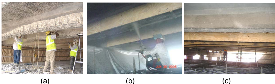
Figure 3-5 (a) Removing loose concrete (b) Applying repair mortar (c) Setting forms
