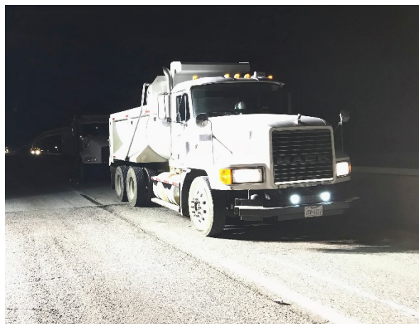
Figure 4-15 Truck in position for load test
