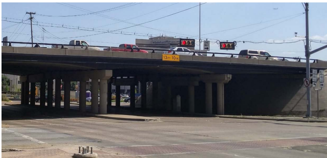
Figure 3-1 MacArthur Bridge Side view
