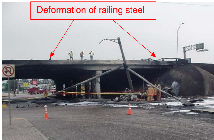
Figure 5-19 Deformation of Steel
