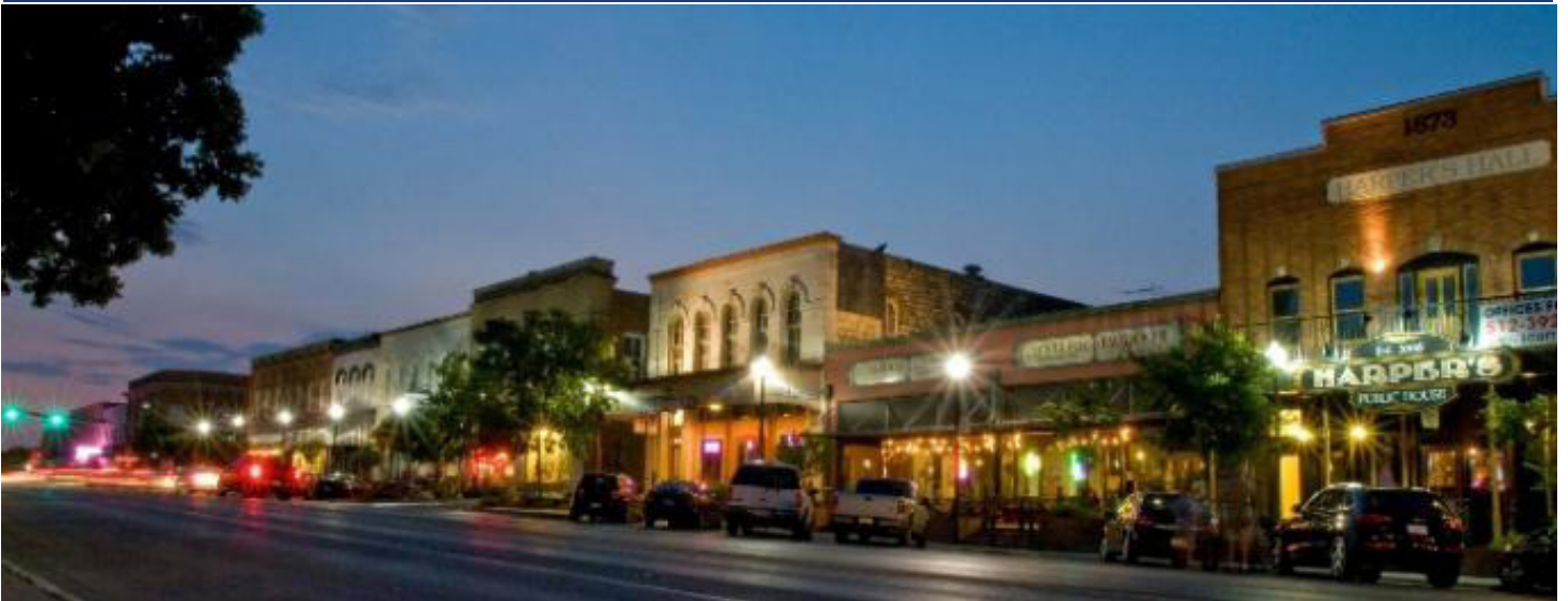
Figure 32. Picture of City of San Marcos, Texas downtown (Photo by City of San Marcos, Texas).
