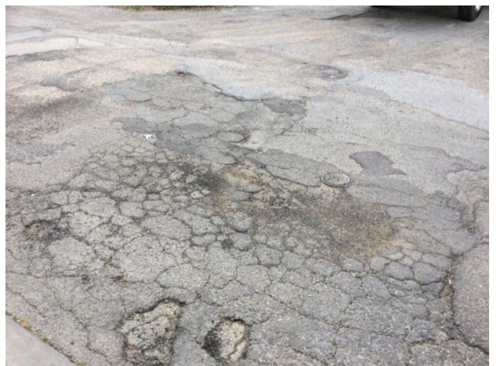
Figure 26. Poor conditioned street (Main Street) in downtown Commerce (picture taken on March 16, 2017 by Colby Collins).
