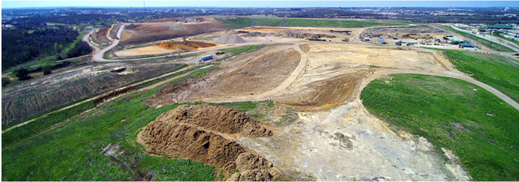
Figure 3-2 Aerial view of Cell 1590 A (cell 0) (photo courtesy: City of Denton)
