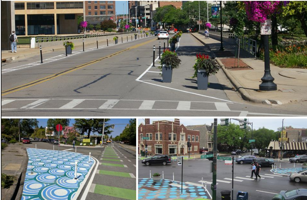
Photo Source: Farr Associates, City of Seattle, John Greenfield.
