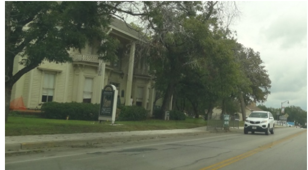
Picture 5: Existing side walk at front of apartment building
