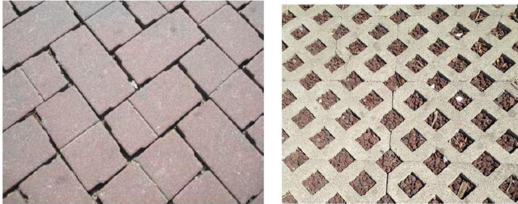
Figure 3: Types of Permeable Pavement. From top to bottom, clockwise; porous asphalt; pervious concrete; grid system; block pavers, (SARA, 2014)
