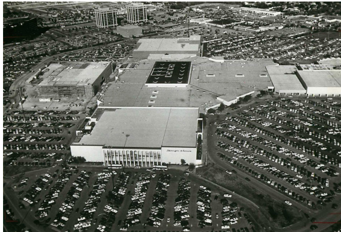
Figure 2: Valley View Center Photo (1982).
