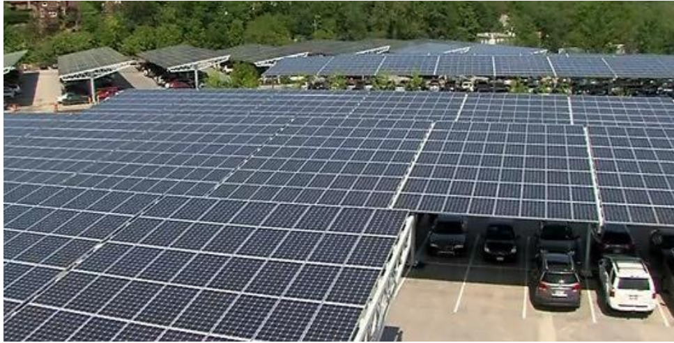
Figure 2.12 Cincinnati Zoo Cincinnati, OH; carport style solar energy system (Source: Largest Publicly Accessible Urban Solar Array (cincinnati-zoo.org, 2010))
