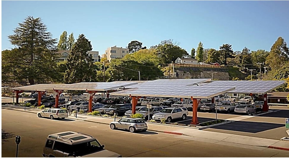
Figure 2.11 City of Santa Cruz, CA; carport style solar energy system (Source: The Registry News Press Release, 2013)
