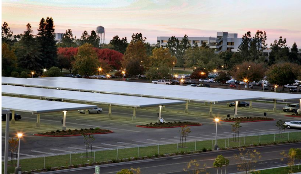
Figure 2.10 Fresno State University, CA; Solar parking canopy
