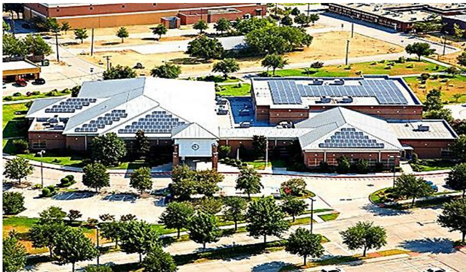
Figure 2.14 City of Duncanville, TX; rooftop solar PV energy systems
