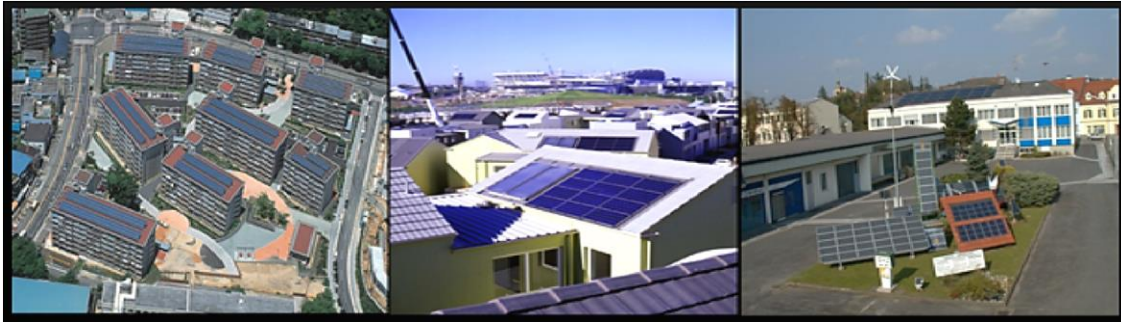
Figure 2.8 Examples of a solar PV system installation in urban areas
