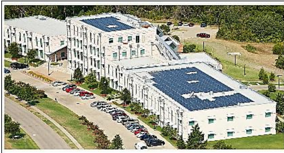
Figure 2.15 City of Cedar Hill, TX; rooftop solar PV energy systems
