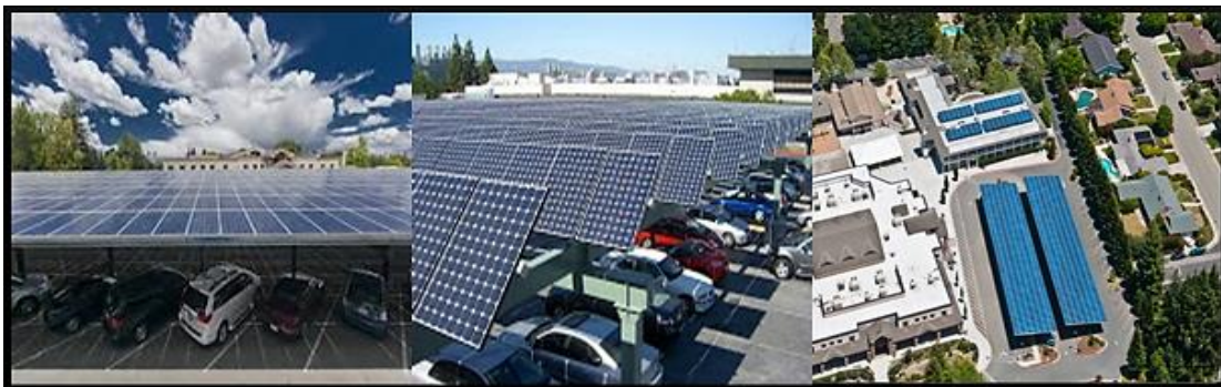
Figure 2.9 Solar parking lots providing shade for parked cars (Source: beforeitsnews)
