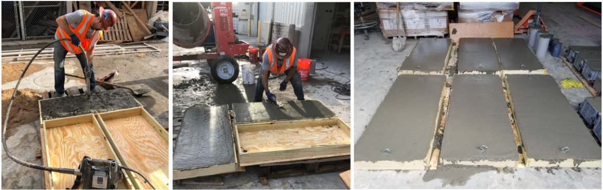
Figure 3- 28. Placing Concrete
