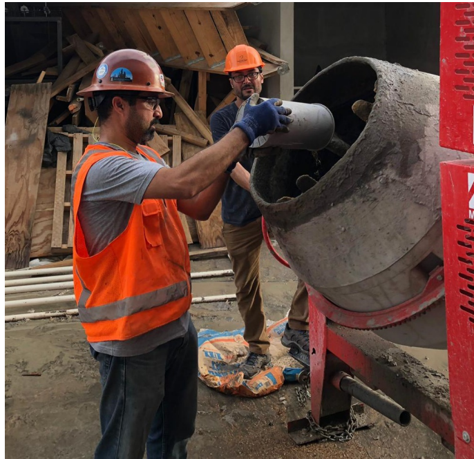
Figure 3- 3. On-site concrete mixer
