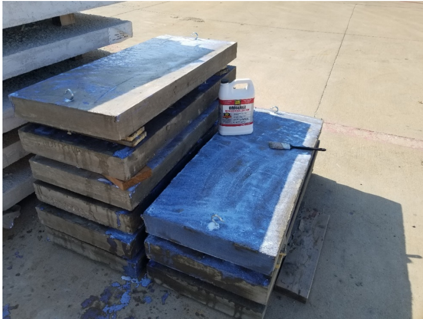
Figure 3- 29. Applied Curing Compound
