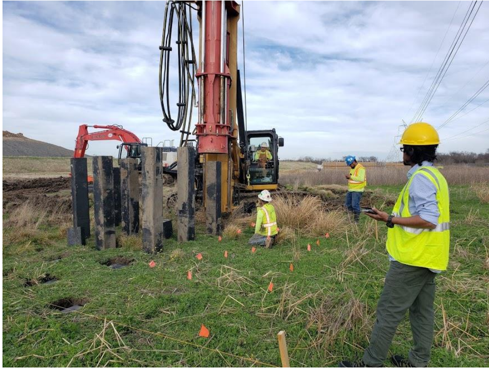
Figure 3.3: Collection of driving time data for 10 in x 10 in RPP section.
