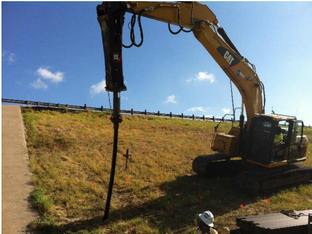
Figure 2.10: Buckling and Permanent Deformation of the RPP in Dry Soil (Hossain et al., 2017).
