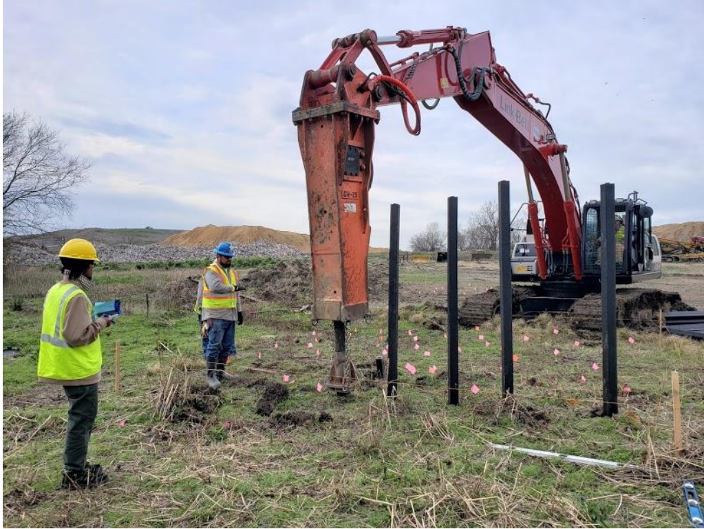
Figure 3.5: Collection of driving time data for 6 in x 6 in RPP section.
