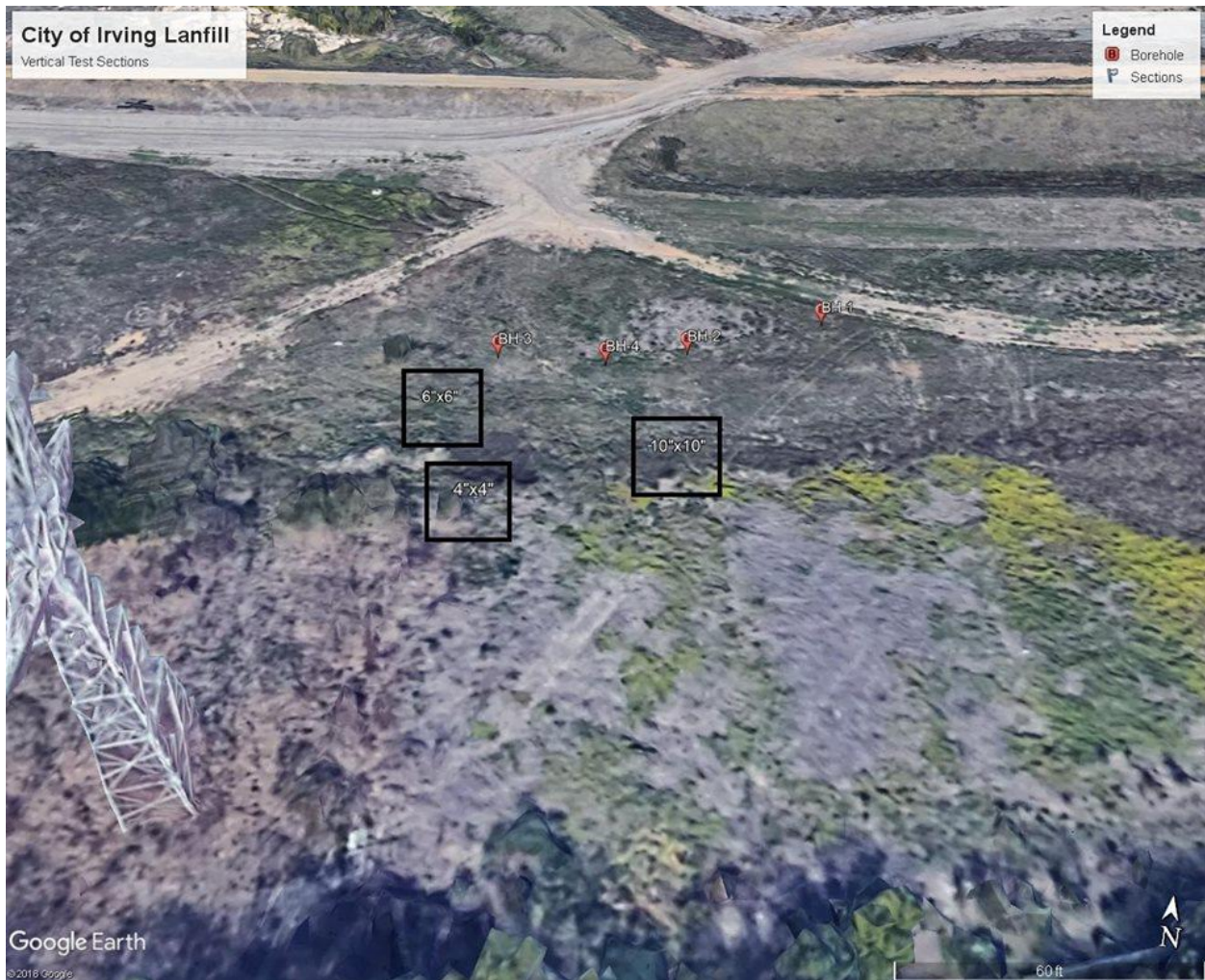
Figure 3.2: Borehole locations for Irving Vertical loaded sections.
