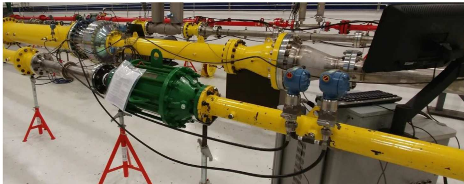
Figure 4-3 Four-inch detonation flame arrester (DFA) test setup photograph
