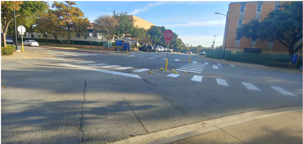
Figure 11 Intersection of Crosswalk 1 facing east.
