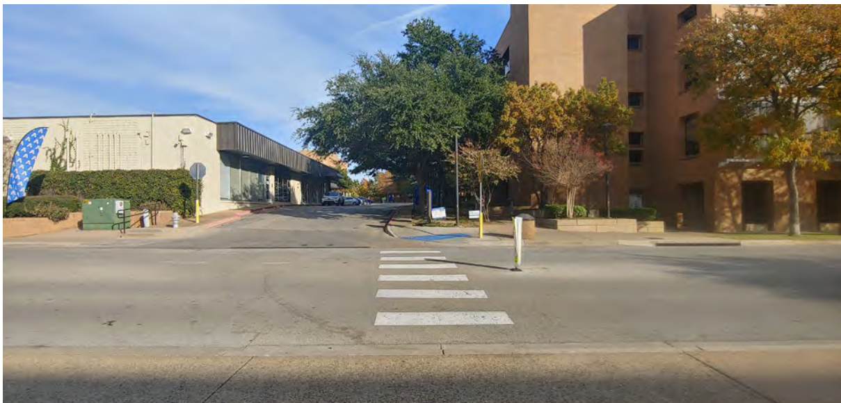
Figure 16 Crosswalk 3 facing east
