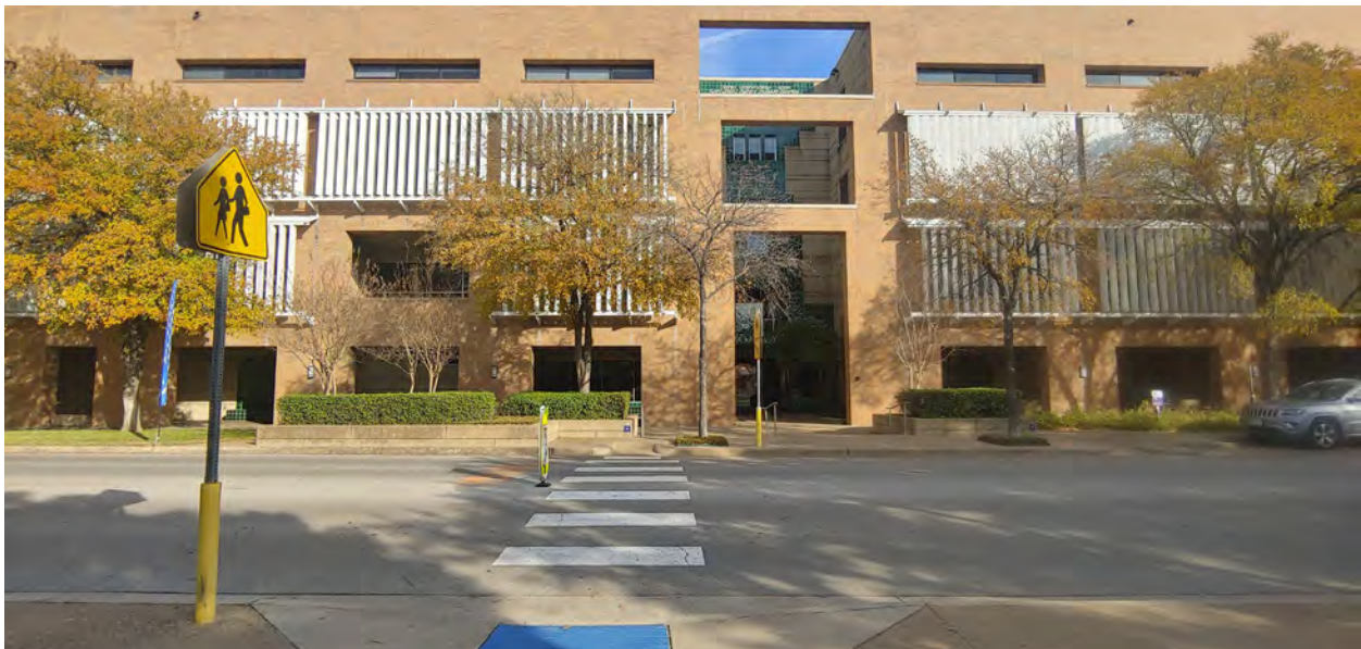
Figure 13 Crosswalk 2 Entrance to CAPP facing east.
