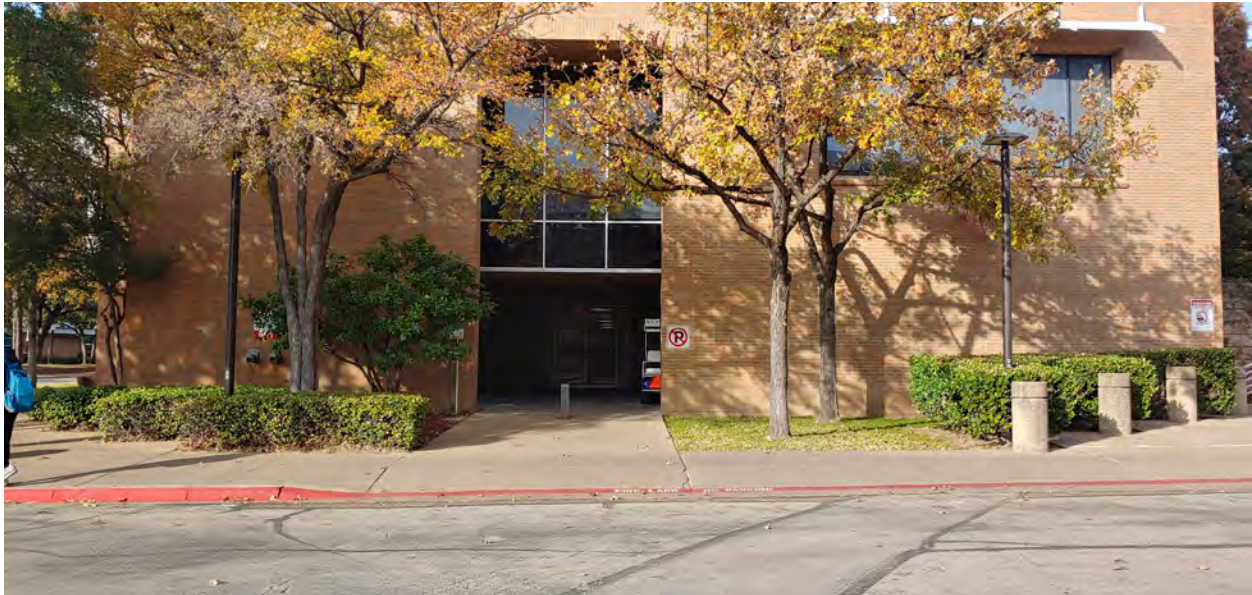
Figure 28 Greek Row Stop 3 facing north
