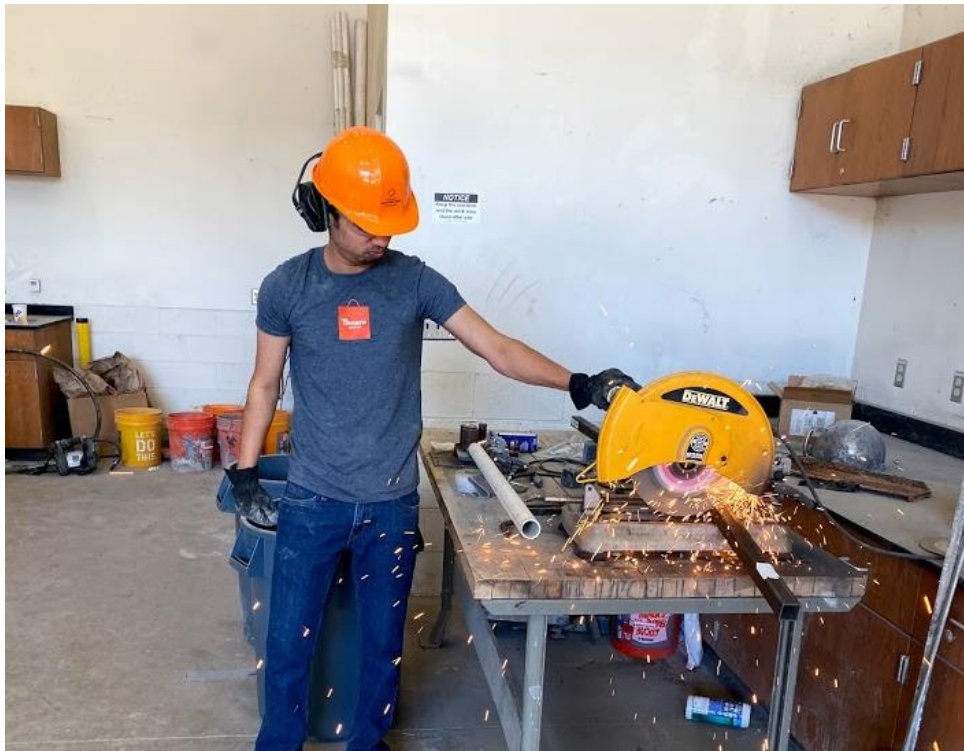
Figure 8 Cutting of HSS Steel Joists
