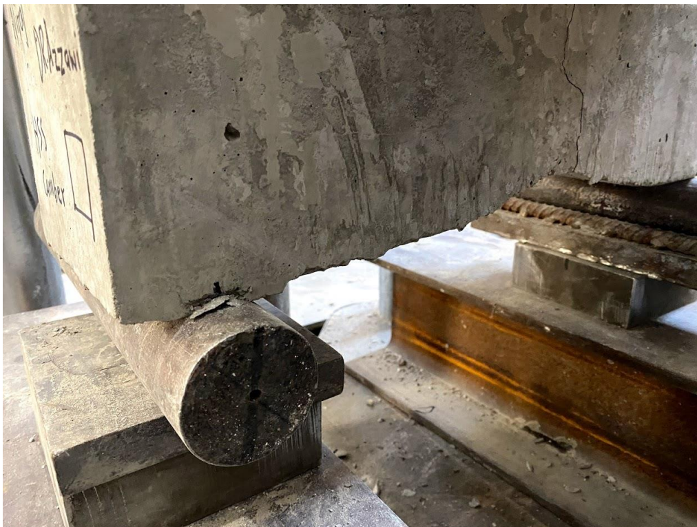
Figure 26 Beam failure and cracks formation for Preflex Beam at Peak Load 0.5%
