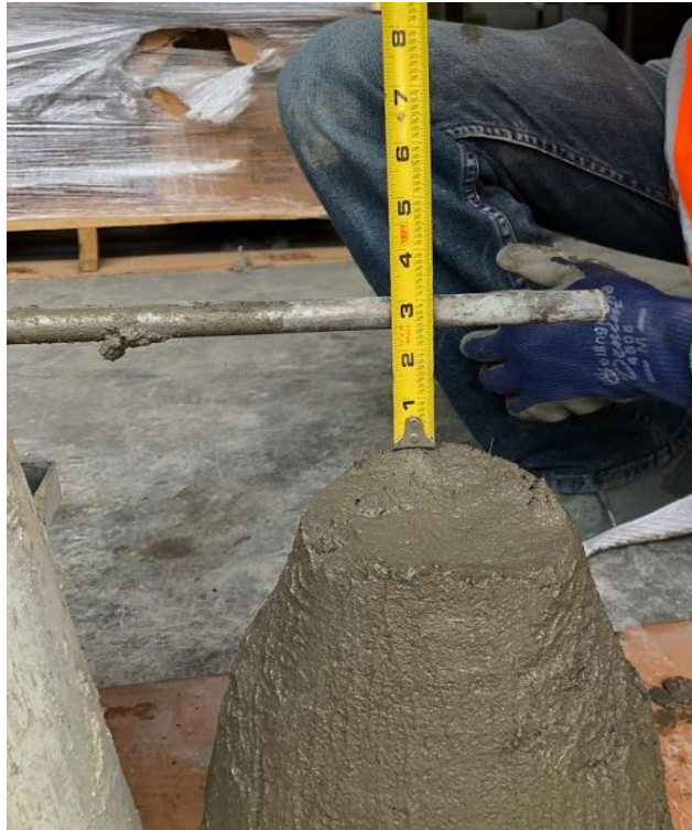
Figure 7 Slump Test of Concrete
