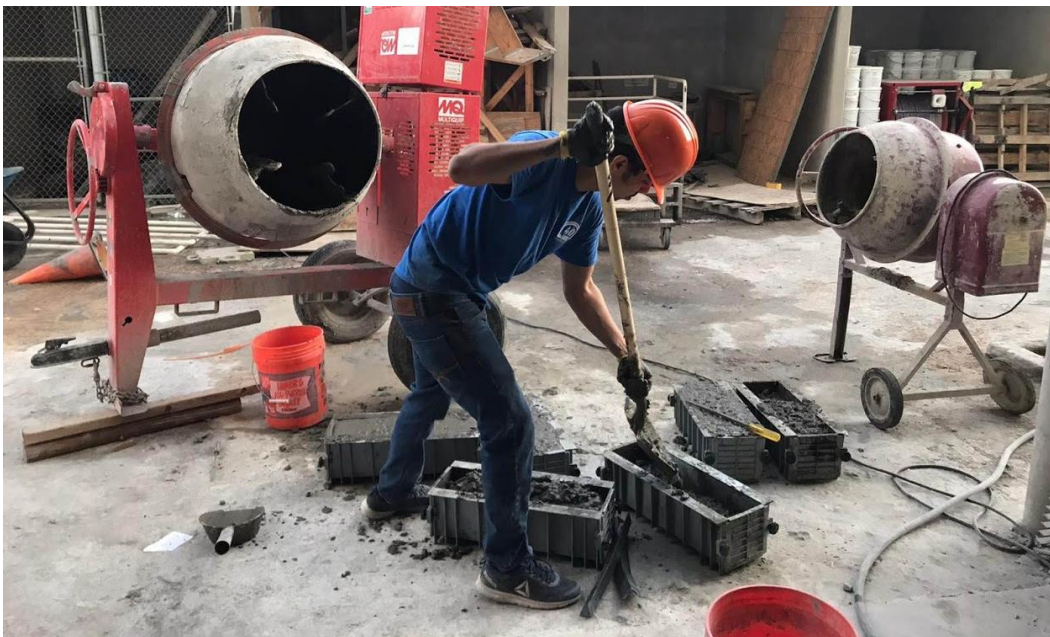
Figure 10 Casting of Beam Specimen
