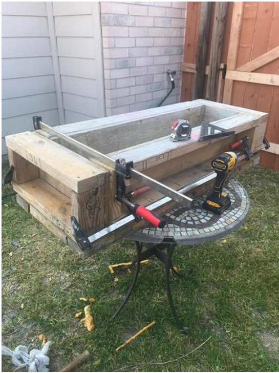
Figure 3.6 Beam Formwork Assembly
