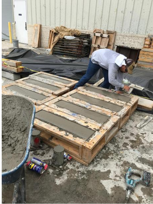
Figure 3.10 Finish of Concrete Beams
