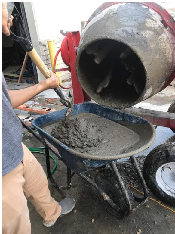
Figure 3.9 Concrete After Mixing
