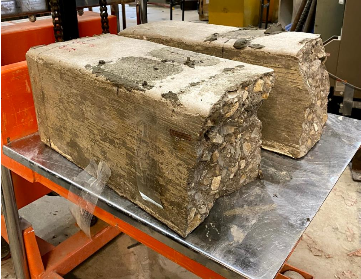
Figure 4.21 Typical Beam Failure with No Heat Exposure
