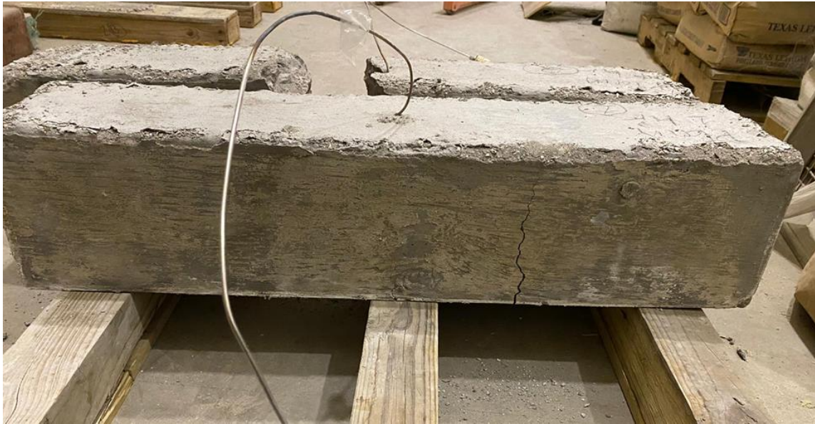
Figure 4.25 Failed Beams Before Testing
