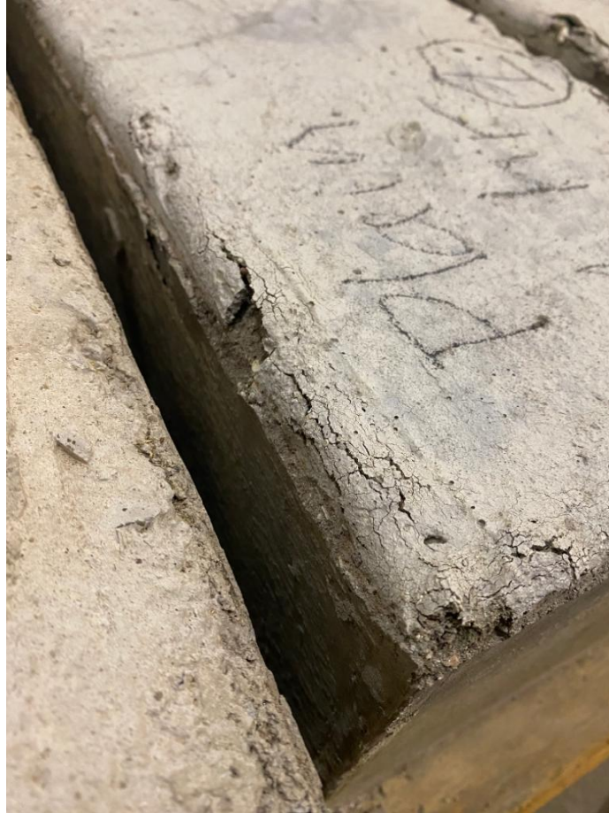
Figure 4.18 Damage of Sample with Regular Concrete After Heat Treatment
