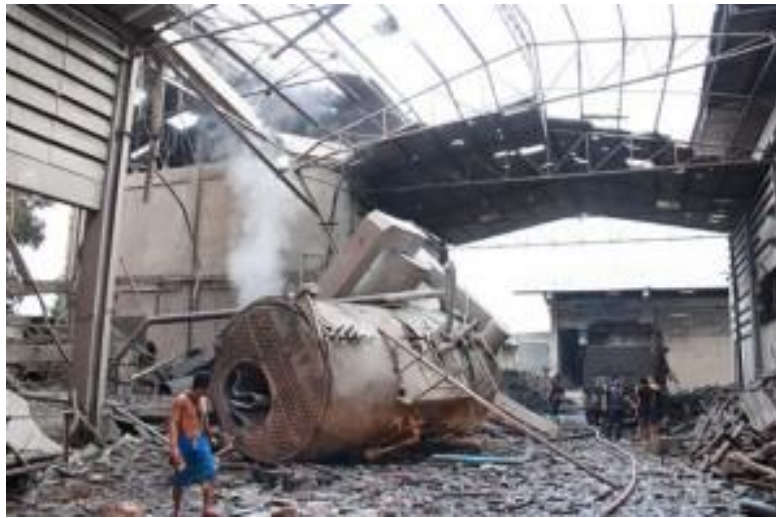
Figure 3 Boiler Explosion at a Dyeing factory in Muang district, Thailand
