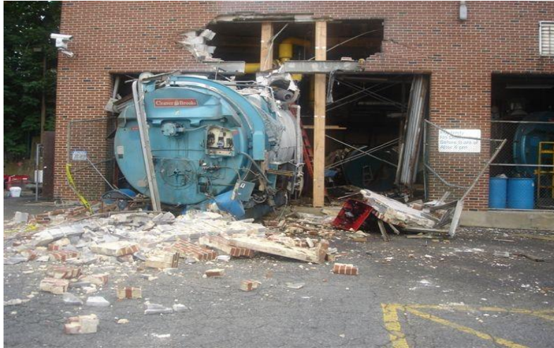
Figure 2 Boiler Explosion at St Mary's Hospital in New Jersey- United States
