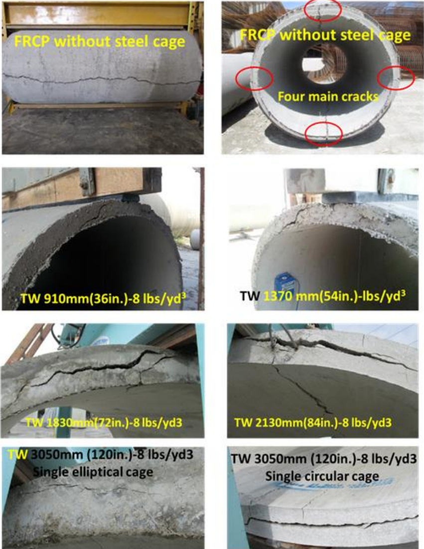
Figure 3.7 Comparison of circumferential cracks in FRCP (w/o a cage) and TW pipes (w/ a cage)
