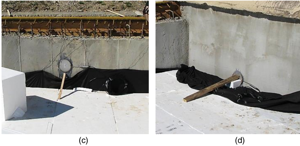
Figure 4.6 Four pressure cells installed at the bridge approach slab
