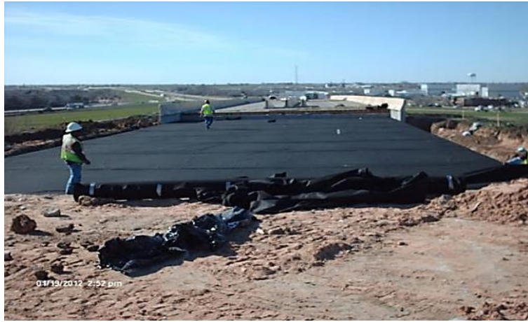
Figure 4.3 Installation of geofabric blocks in January 2012 (Ruttanaporamakul 2015)
