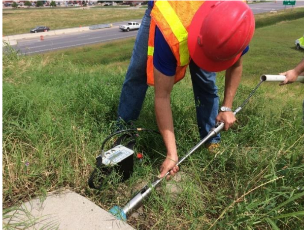
Figure 5.1 Horizontal inclinometer survey
