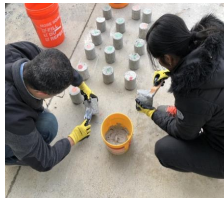
(e) Patching of voids
