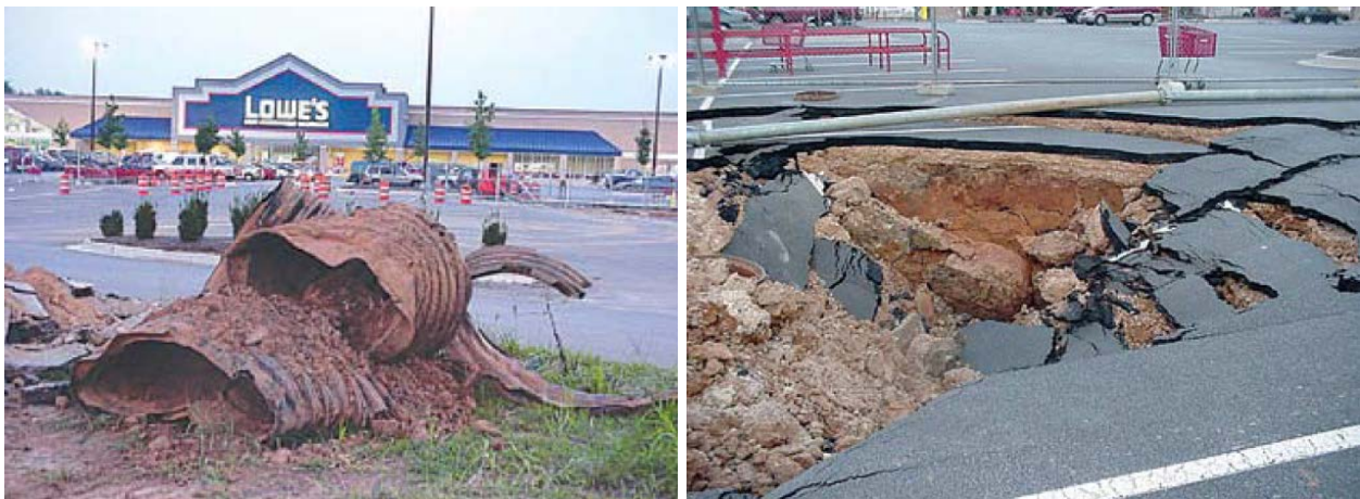
Figure 1-5. Failure of a 4-year old HDPE culvert (ACPA 2008).
