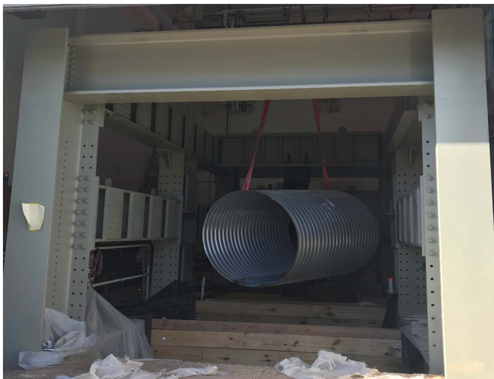
Figure G-8. Pipe installation.
