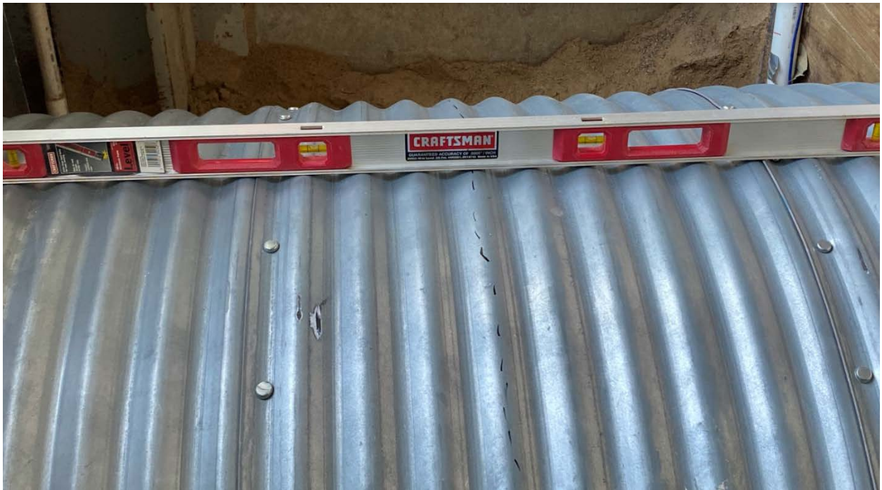
Figure G-7. Foundation and pipe's top leveling check.
