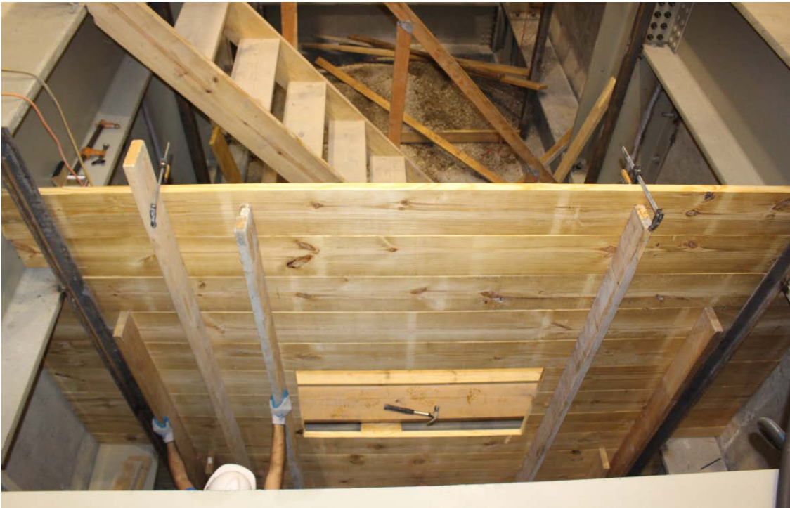
Figure G-3. Partition wall construction and soil box preparation.
