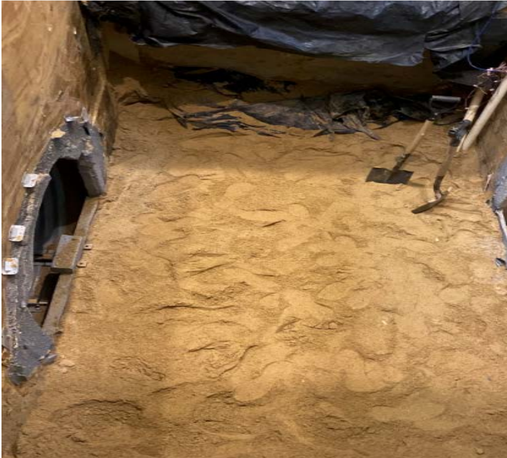
Figure G-5. Foundation Preparation using SP soil
