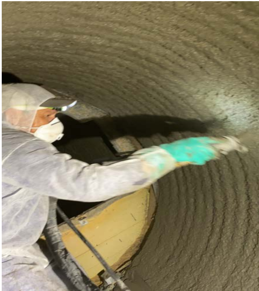
Figure G-24. Spray applied lining installation.
