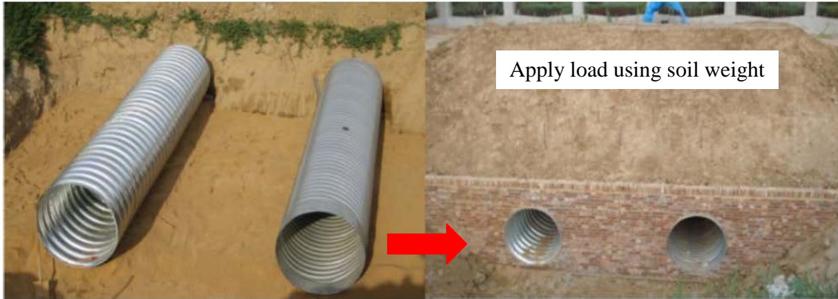
Figure 2-2. Field pipe testing using soil dead load (Liu et al. 2016)
