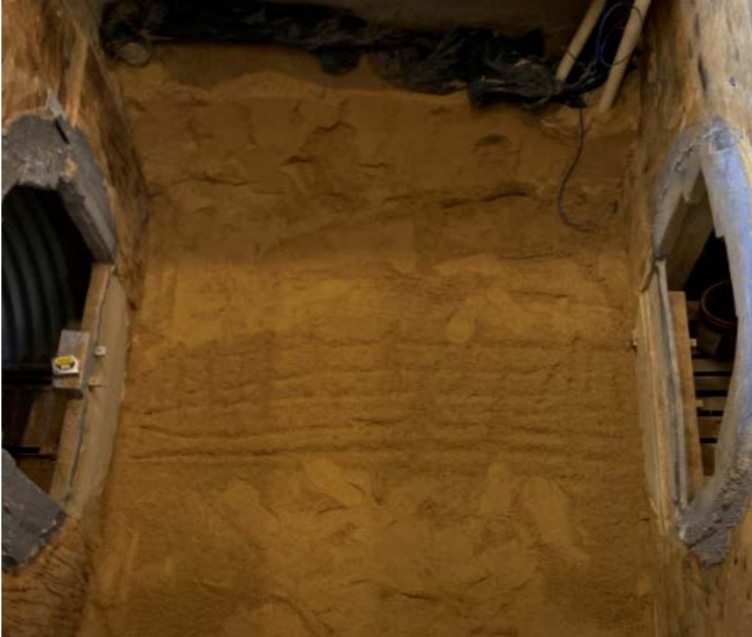
Figure G-6. Foundation compaction, leveling, and scratching.
