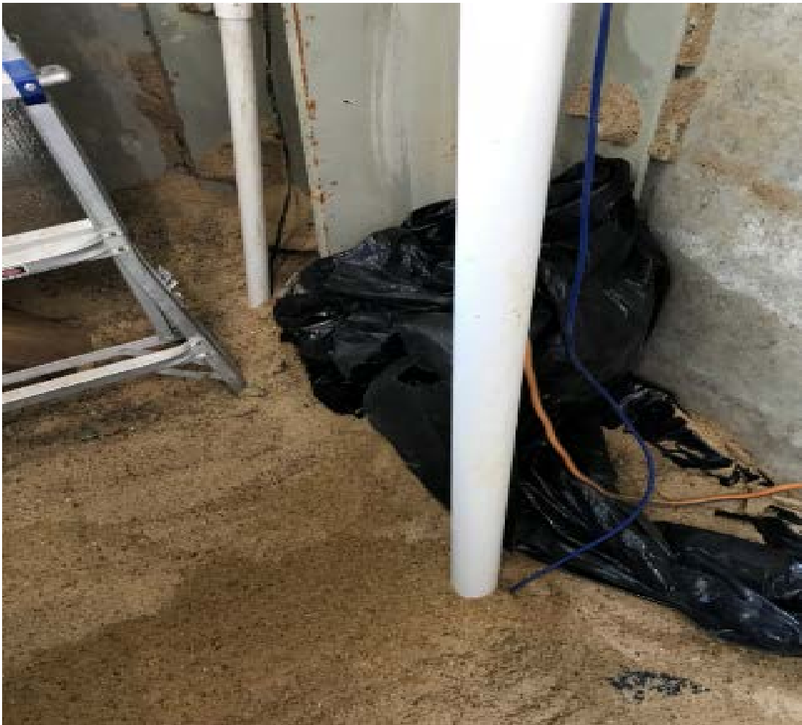
Figure G-14.PVC duct to protect the strain gauges wires.
