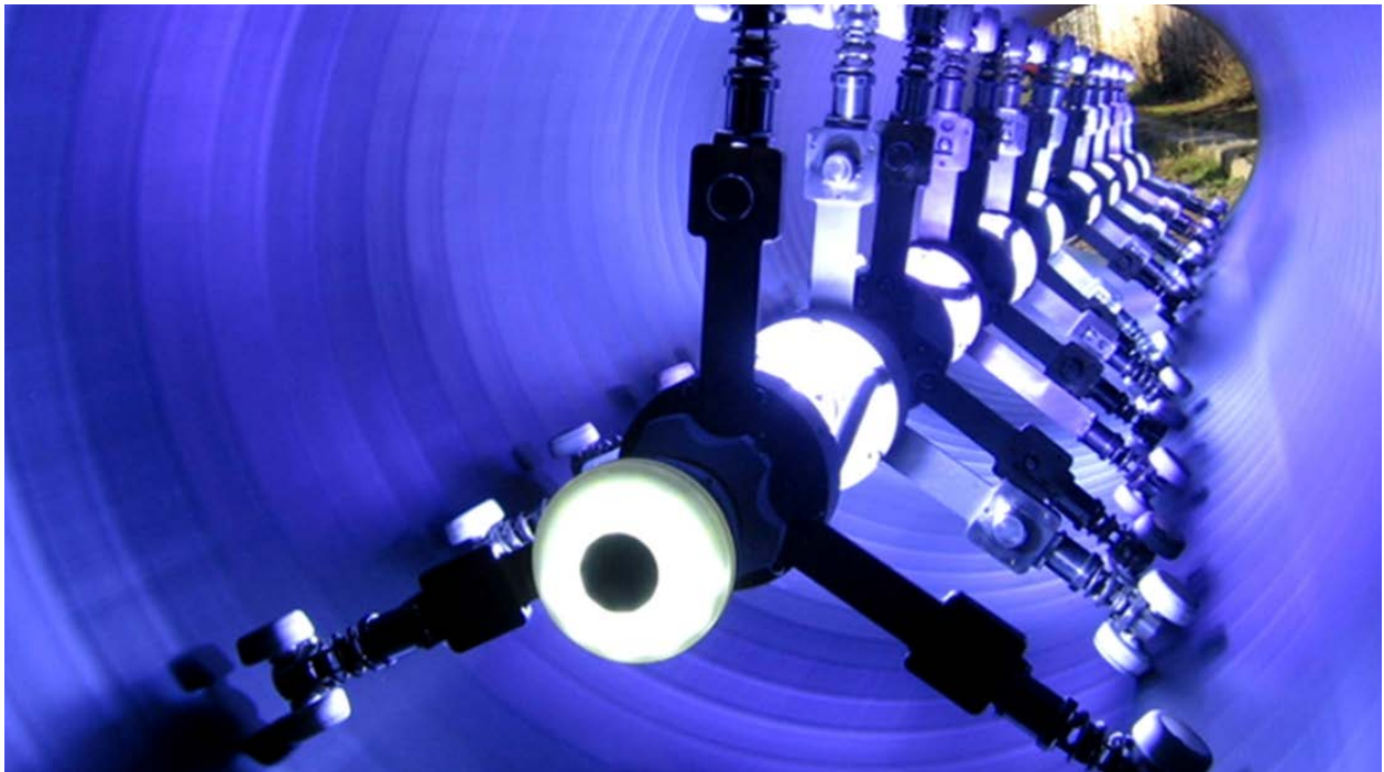
Figure 1-23. CIPP curing using UV light (photo credit: ohm-advisors.com).
