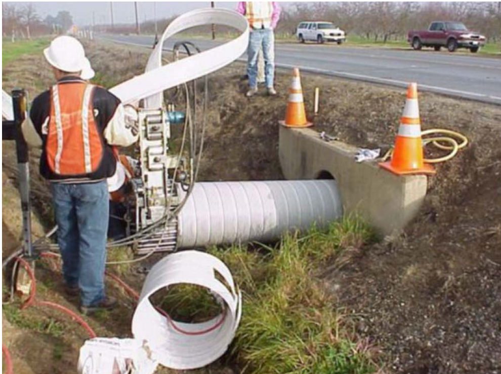
Figure 1-24. Spirally wound liner installation (Wagener and E. Leagjeid 2014).
