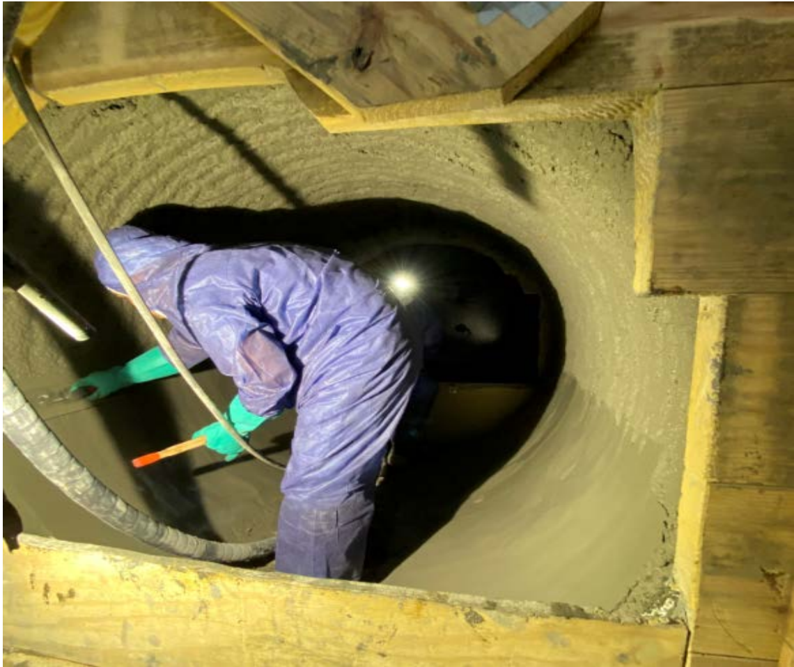
Figure G-23. SAPL Spraying and surface finishing.
