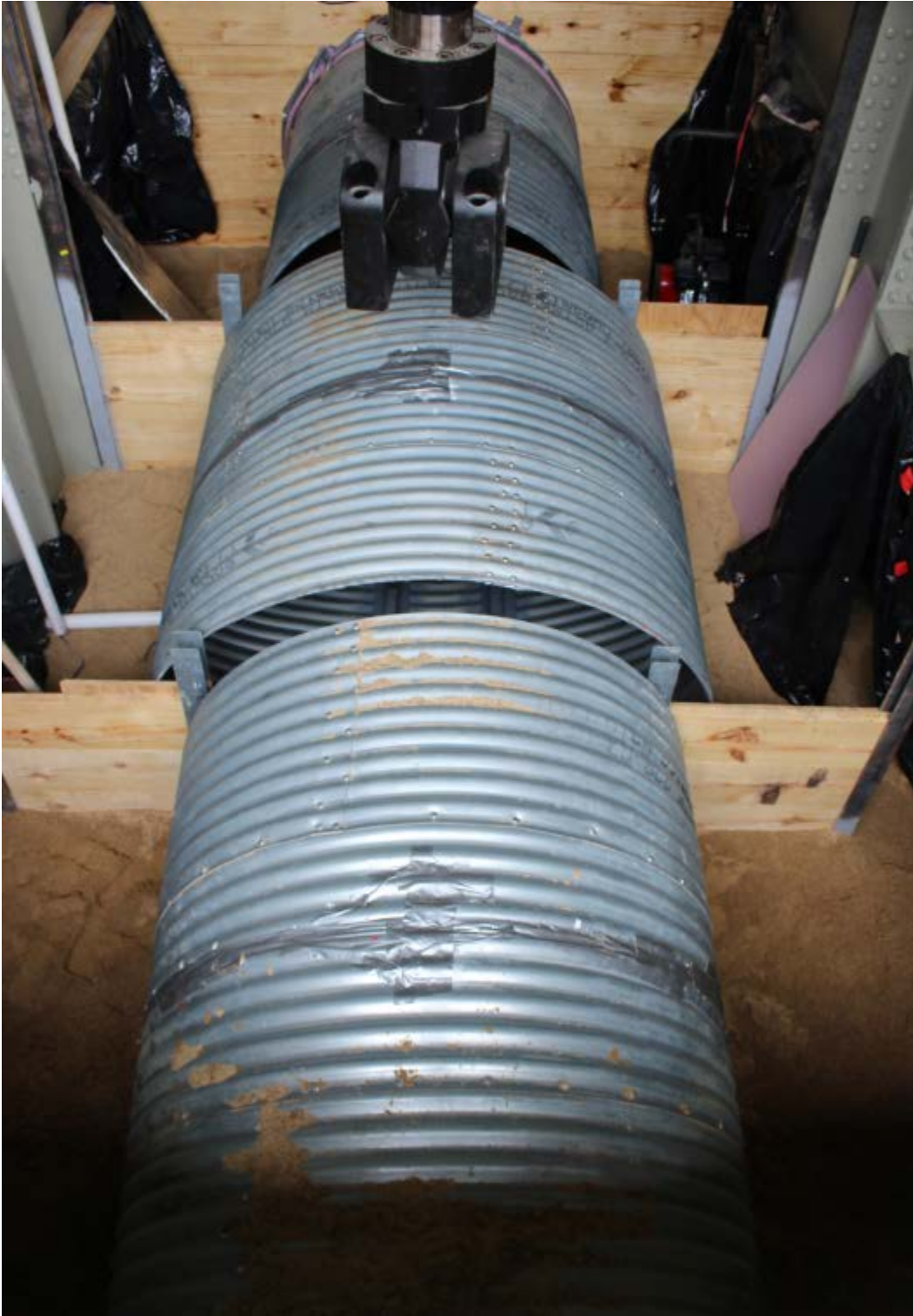
Figure G-9. CMP installation.
