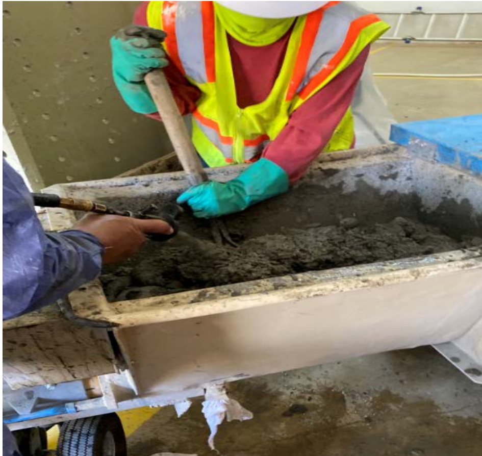
Figure G-22. Cementitious SAPL mixing and pumping.
