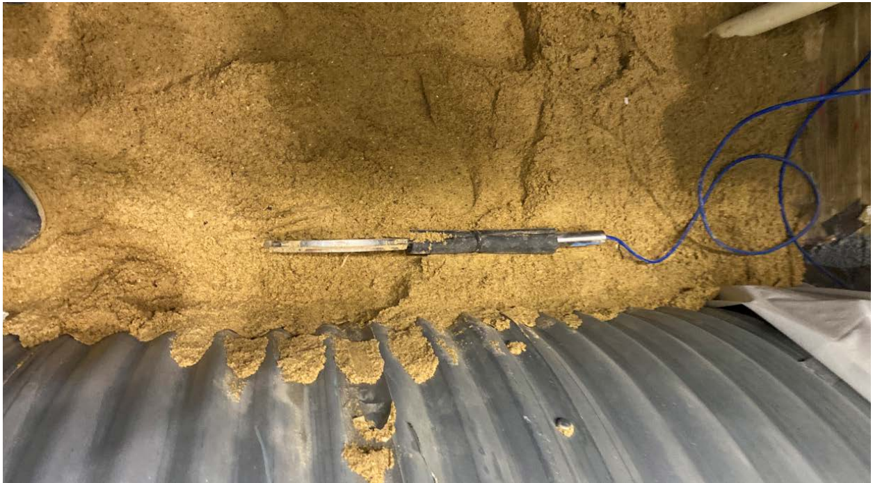
Figure G-18. Surface leveling and earth pressure cell installation.
