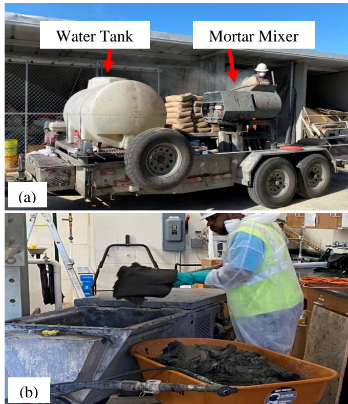
Figure 3-38. Cementitious SAPL installation equipment including: (a) portable mortar mixer, water tank, and (b) rotor-stator pump.
