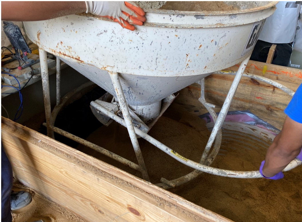
Figure G-17. Soil placement using casting bucket.
