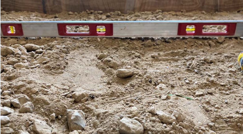
Figure G-19. Aggregate top surface leveling.
