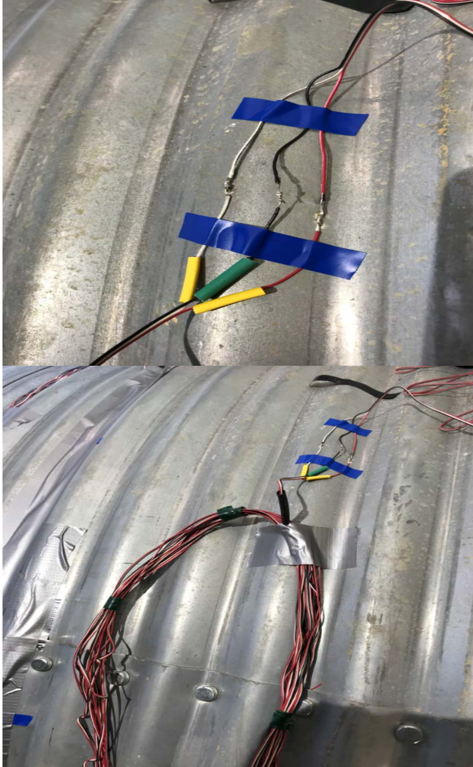
Figure G-12. Outside strain gauge installation
