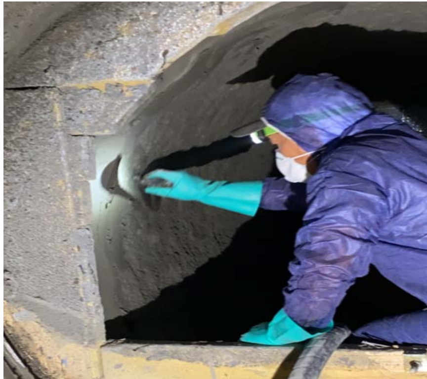
Figure G-25. Spraying and troweling.
