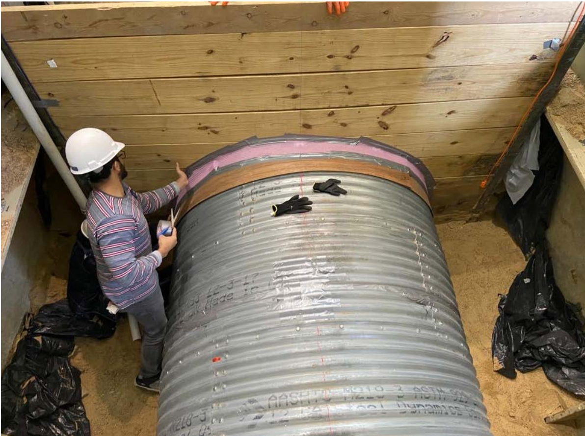
Figure G-10. Pipe-wall gap sealing.
