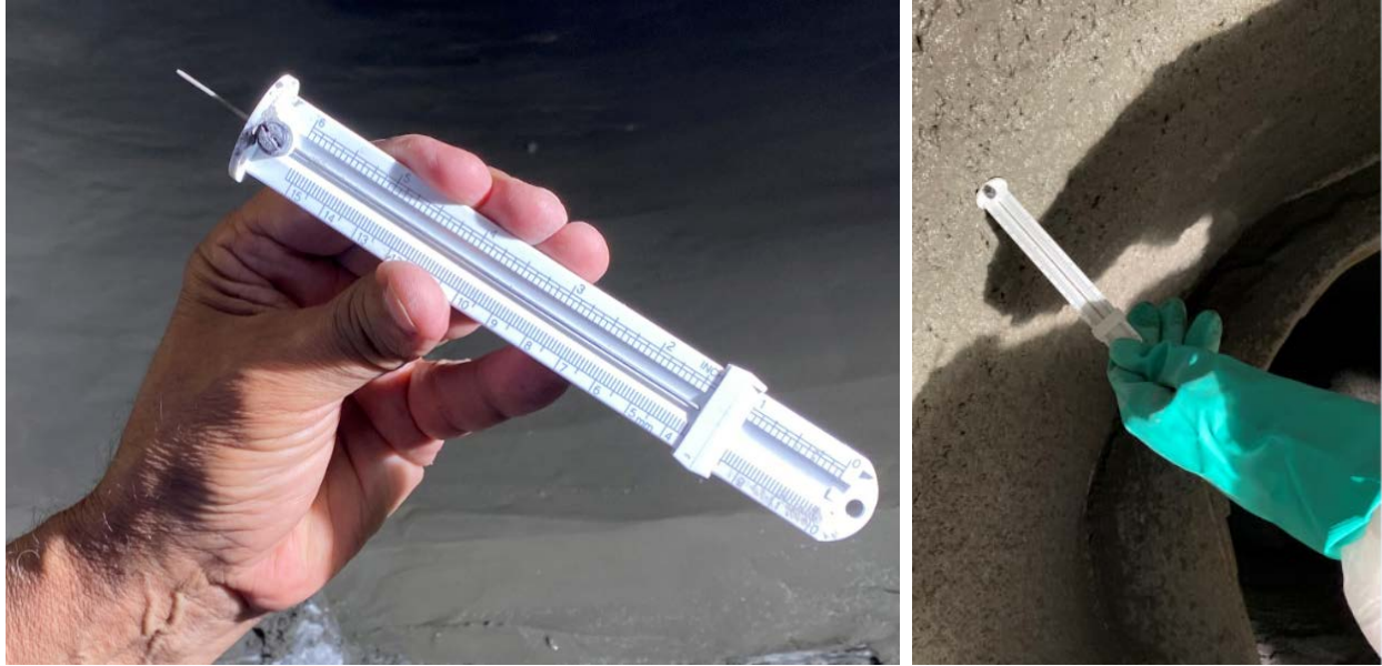
Figure 3-42. Thickness measurement using a depth gauge at the time of SAPL installation.
