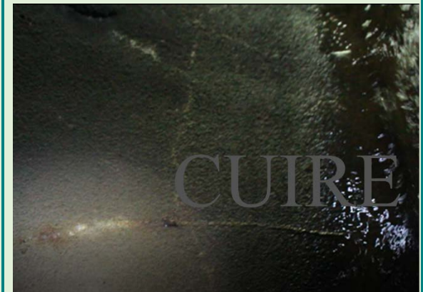
Multiple Cracks
