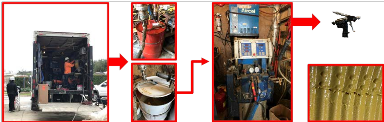
Figure 4-17 Hand spray SAPL installation.
