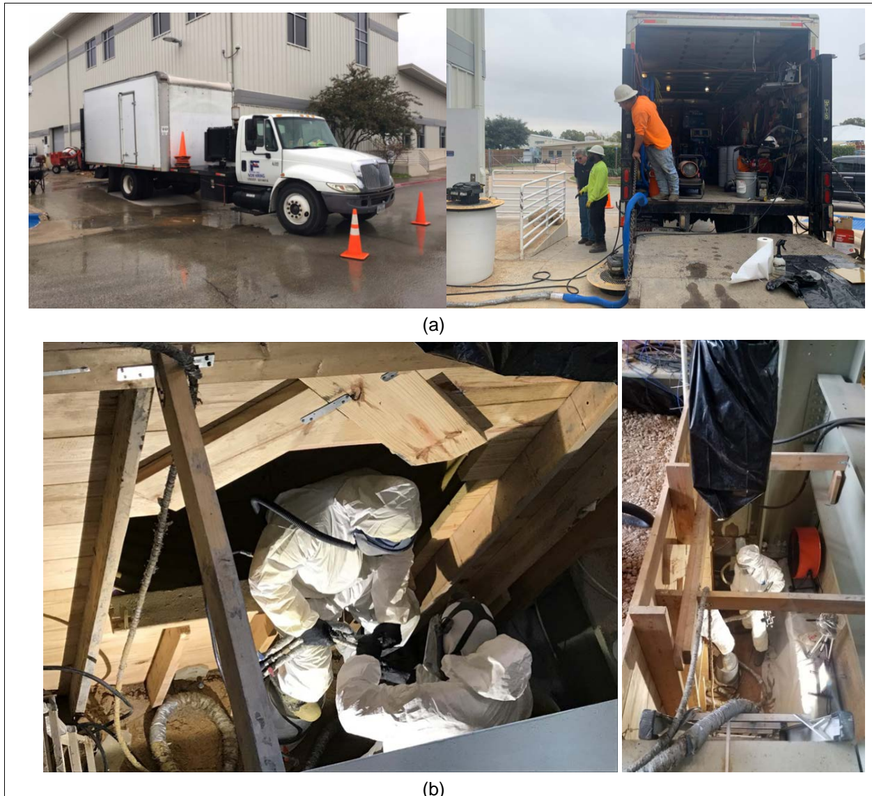
Figure 4-18 SAPL installation on circular CMP, CUIRE laboratory, UTA, 10/29/2019: (a) outside of the laboratory, and (b) inside of the soil box.
