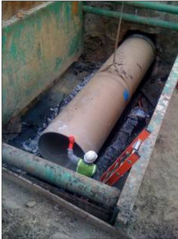
Figure 1-20 Segmental sliplining method (Source: Hobas Pipe USA).
