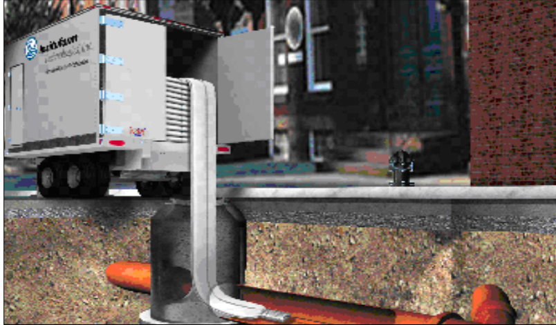
Figure 1-21 CIPP method installation process (Source: Insituform Technologies).
