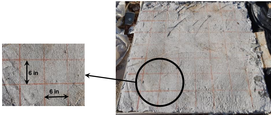
Figure 4-3 Grid lines on the slab
