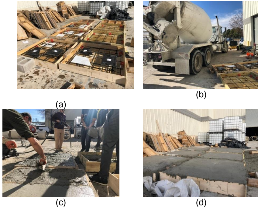
Figure 3-4. The slump of the concrete mix was 8 in (200 mm).
