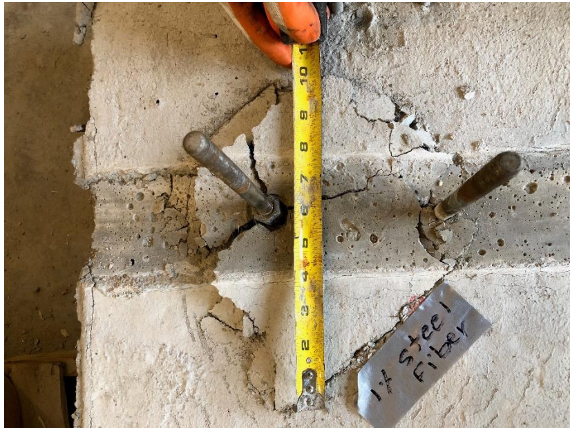
Figure 3.26 Concrete Breakout Failure (1.0% SFRC)
