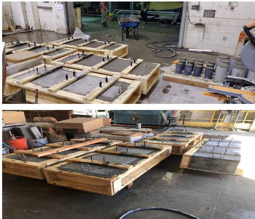
Figure 3.8 SFRC During the Pouring Day and After
