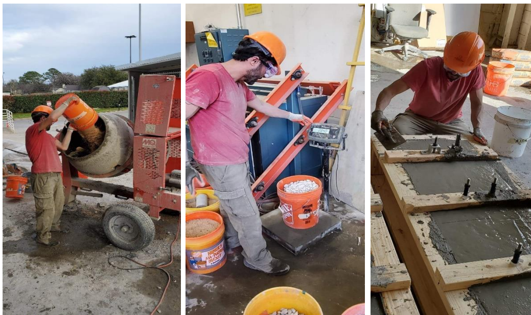
Figure 3.5 On-Site Concrete Mix
