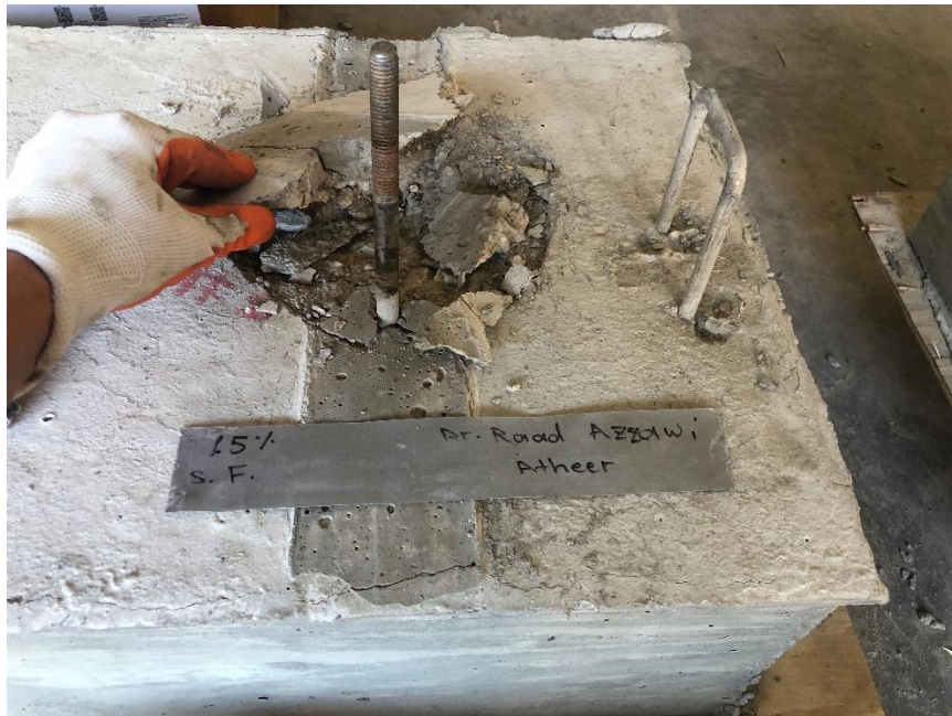
Figure 3.27 Concrete Breakout Failure (1.5% SFRC)
