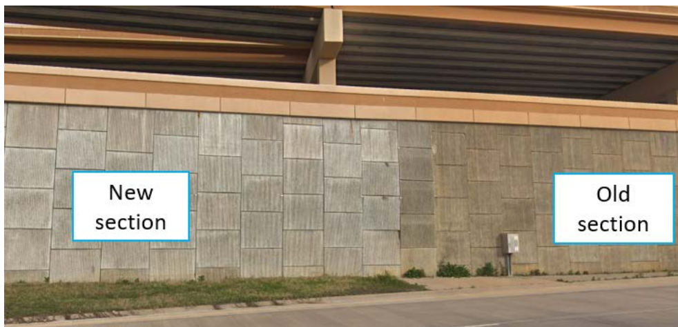
Figure 3-2 Old and new sections of Wall 264R
