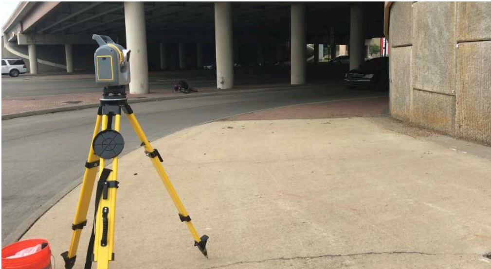
Figure 4-8 SX10 robotic laser scanner setup above a control point
