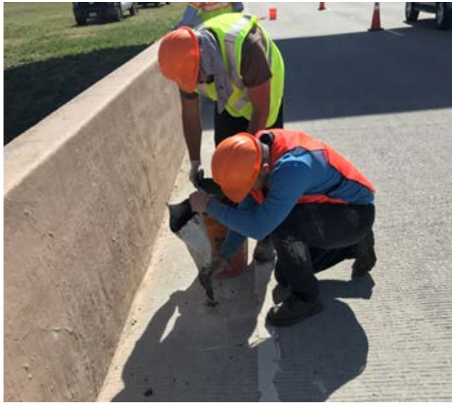
(e) Patching the holes with rapid concrete mortar
