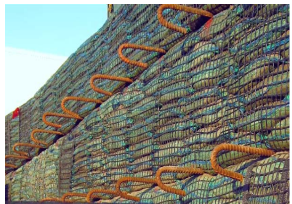
(f) Cast-in-place (CIP)
