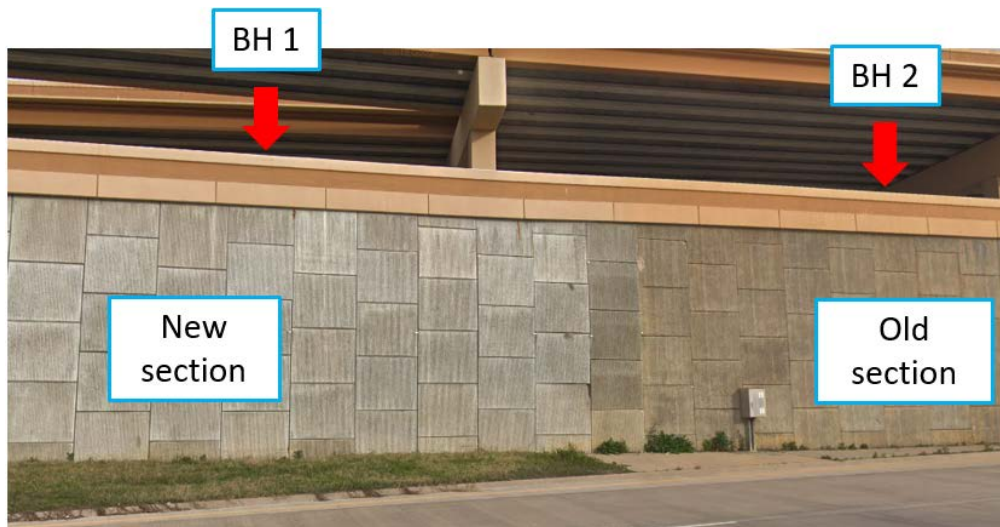
Figure 4-51 Old and new sections of Wall 264R
