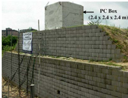
Figure 2-22 Surcharge load application through the poured concrete (PC) box (Yoo and Kim 2008)
