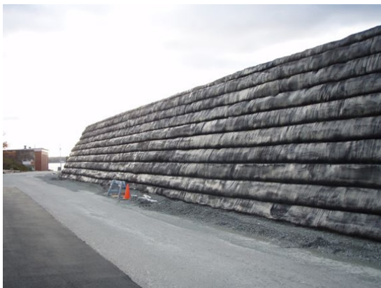
(e) Geosynthetic reinforcements
