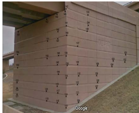
Figure 4-10 Target locations at (a) Wall 264R, (b) Wall 179L, and (c) Walls CC1-3
