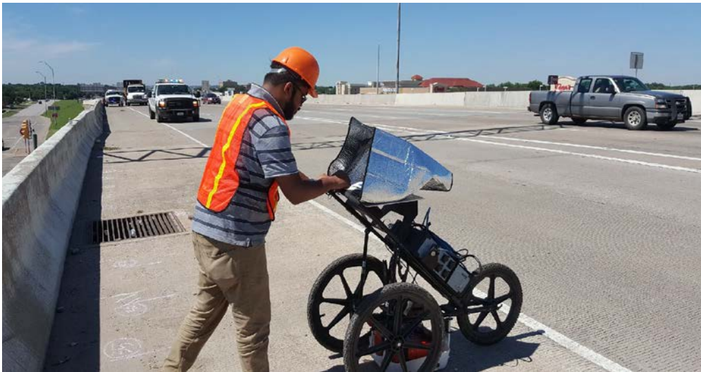
Figure 4-17 GPR scanning with 400 MHz antenna
