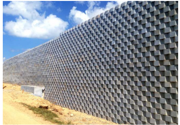
(b) Modular block wall (MBW)
