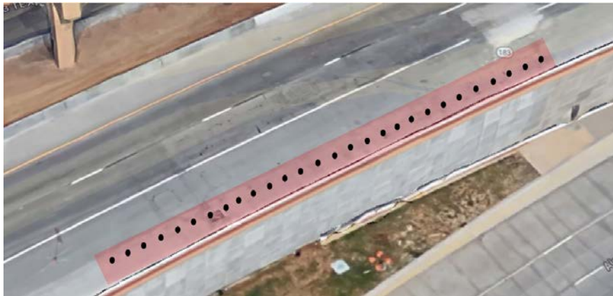
(a) RI scan area at Wall 264R
