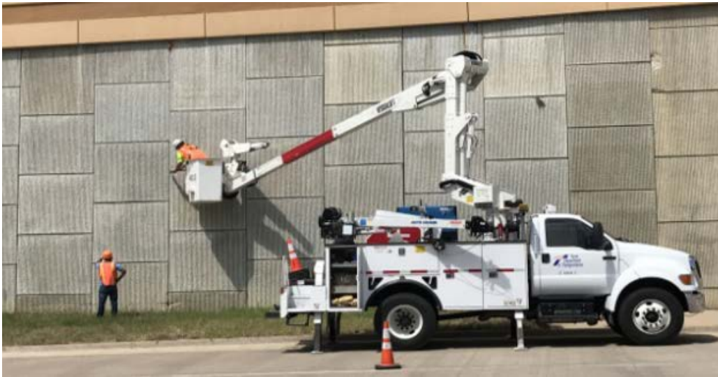
Figure 4-9 Installing targets using a bucket truck
