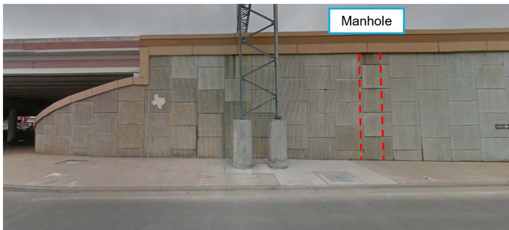
Figure 3-10 Manhole location at Wall 179L
