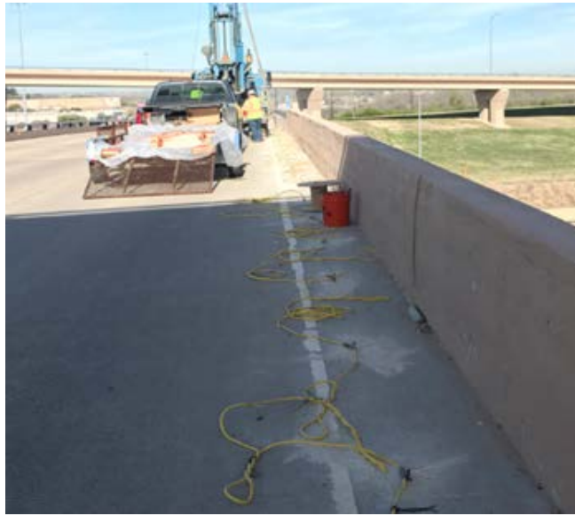
(c) Connecting the electrodes to RI cable
