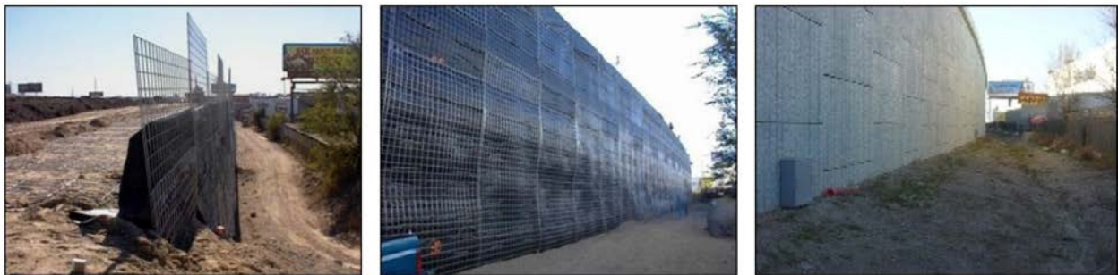
Figure 2-11 MSE wall reconstruction phase (Budge et al. 2006)
