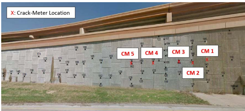
Figure 4-13 Crack meter locations at Wall 264R
