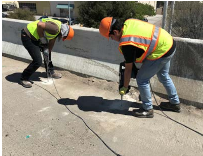
(a) Drilling 28 holes
