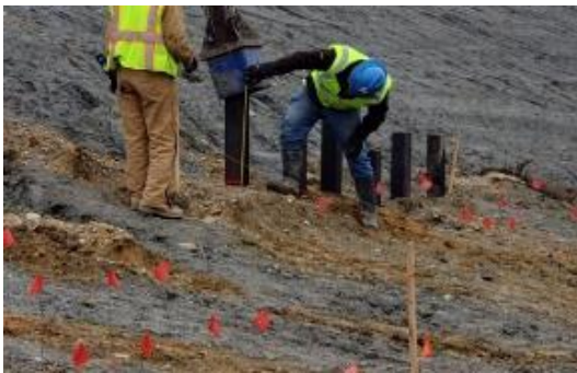
Driving the pin upto 8 ft. length
