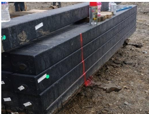
Marking of pins at 8 ft. from the bottom end / 2 ft. from the top end
