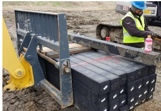
Marking of pins at 8 ft. from the bottom end / 2 ft. from the top end
