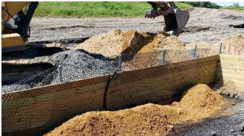
Placement of sand layer
