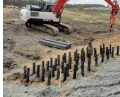
Driving the pin upto 8 ft. length
