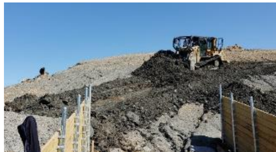
Backfilling from behind the section
