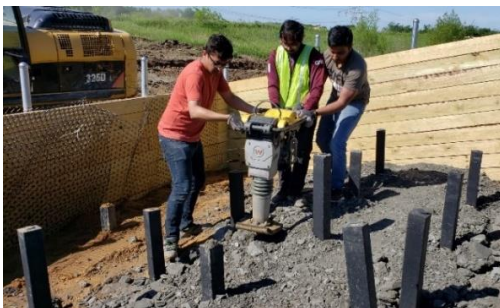
Compaction using Jumping Jack compactor
