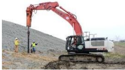
Placing the hammer system over the pin
