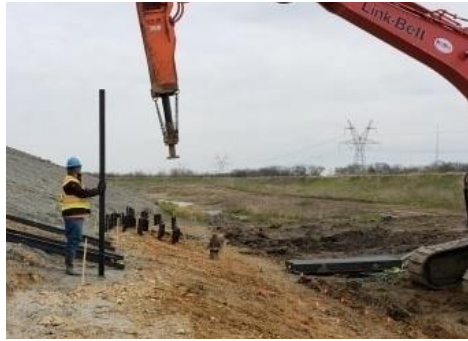
Positioning the pin at marked location
