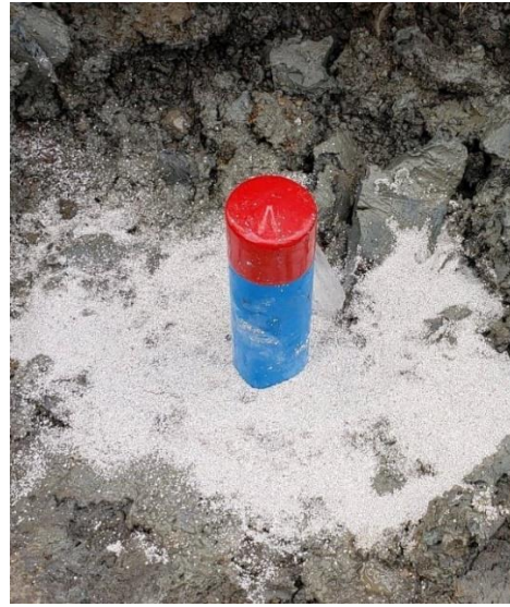
Figure 3-22 Installation Sequence of Vertical Inclinometer Casings
