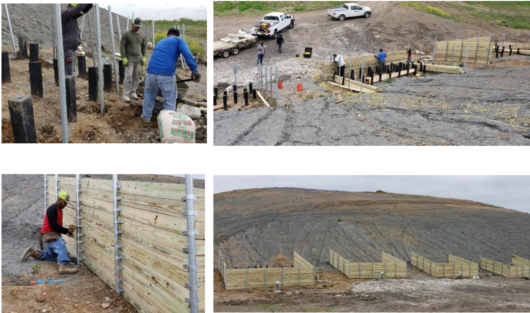
Figure 3-24 Construction of Test Sections
