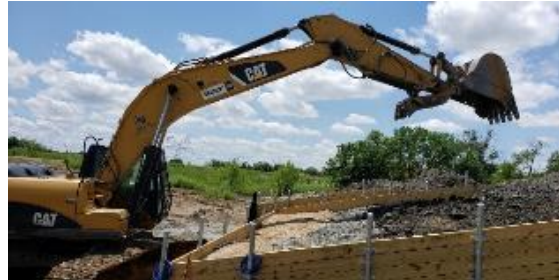
Placement of clay layer
