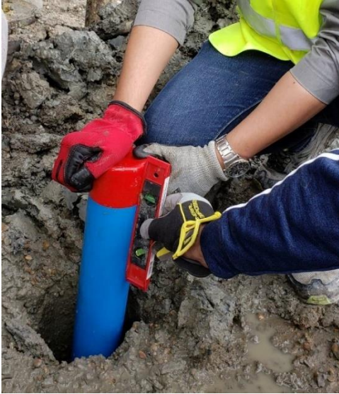
Figure 3-22 Installation Sequence of Vertical Inclinometer Casings
