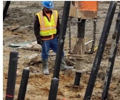
Driving the pin upto 8 ft. length
