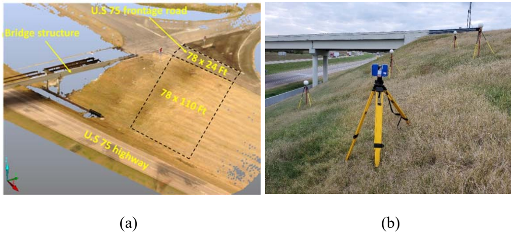
Figure 6.17 (a) LIDAR surveying area and (b) LIDAR surveying on the treated slope section
