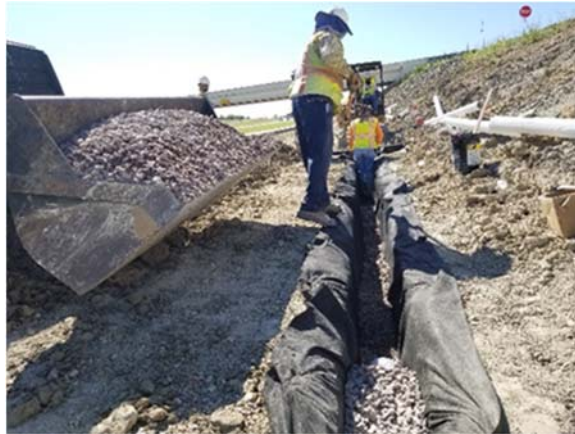
Figure 6.9 Installation of longitudinal underdrains
