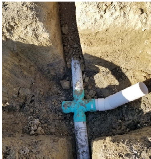
Figure 6.10 Connection of longitudinal and lateral drainpipes
