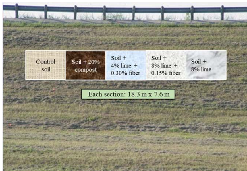
Figure 3.15 Layout of the treated test sections for Grapevine and Joe Pool dams
