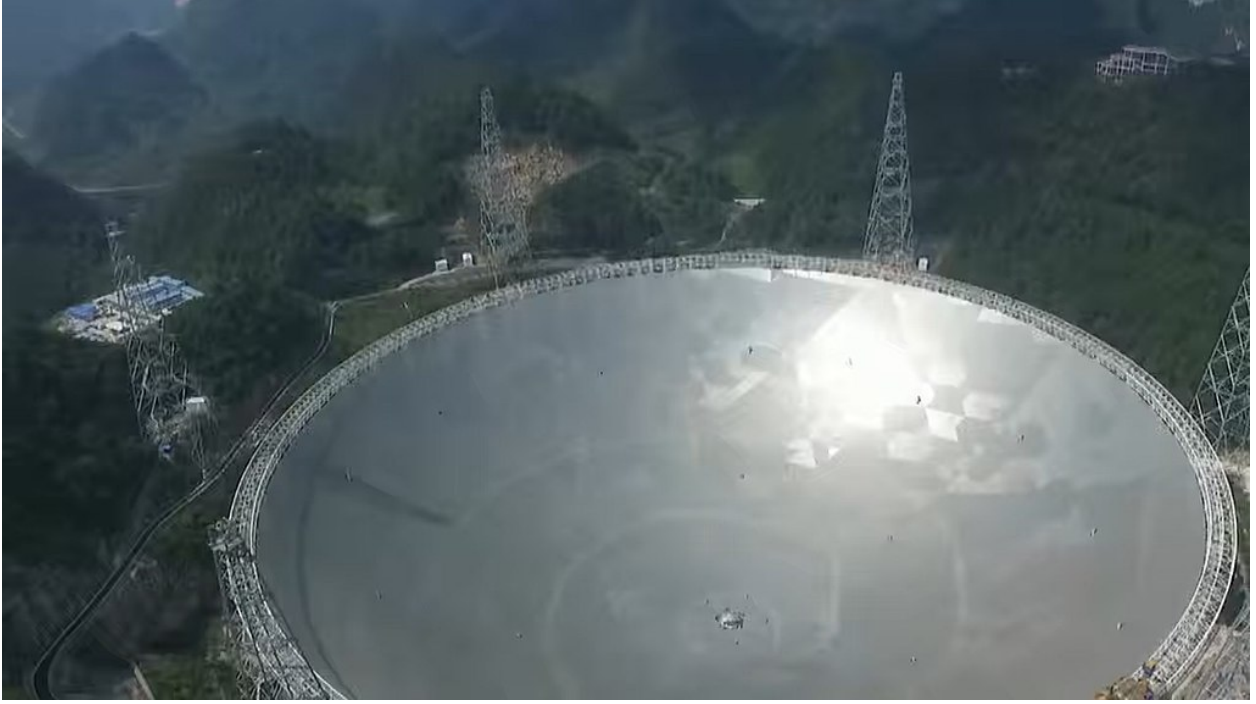
Figure 1.4: At the time of this writing the largest filled-aperture single dish radio telescope in the world is the Five-hundred-meter Aperture Spherical radio Telescope (FAST) in China. Credit: AbsoluteCosmos [2020]
