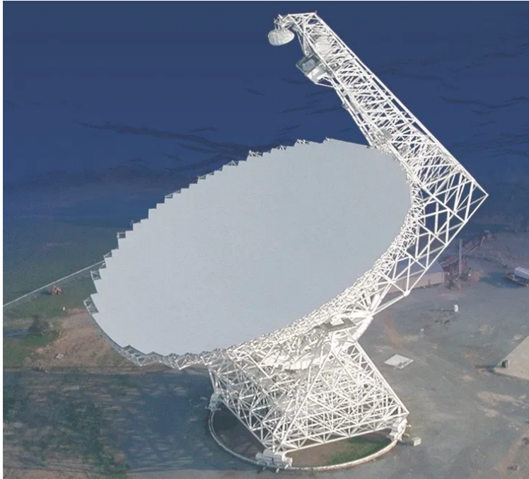
Figure 3.11: The Robert C. Byrd Green Bank Telescope (GBT). With a 100 m diameter collecting area, the GBT is the world’s largest fully steerable radio telescope. Credit: Green Bank Observatory
