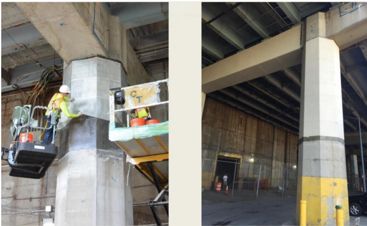
Fig 2.5: Application of pre-saturated CFRP on RFK bridge (Triborough bridge), NYC (White, 2018)
