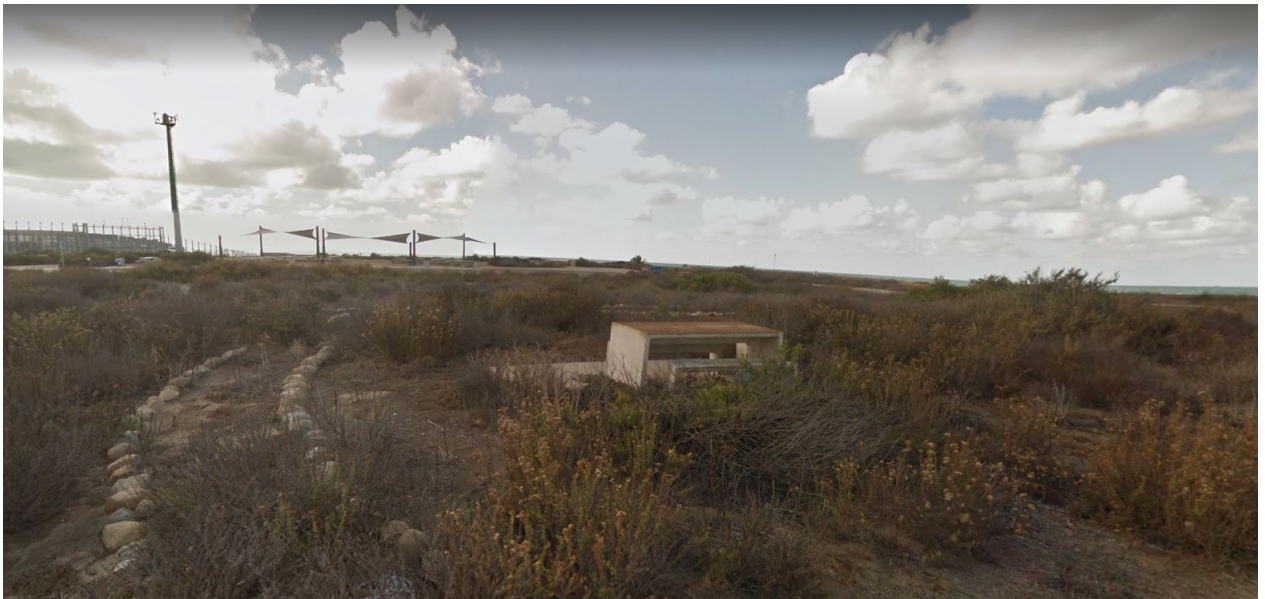
Figure 4.11. Weathered Concrete Benches
