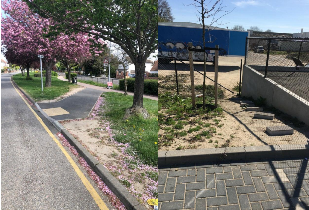
Figure 9 - Differing Quality of Paving Add Desire Paths into Formal Path Network
