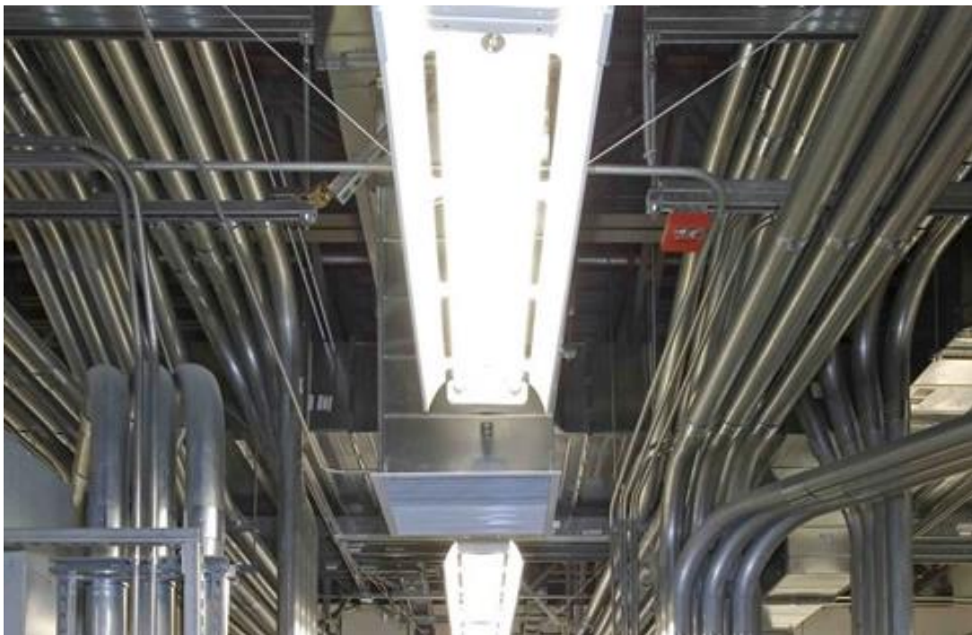
Figure 4- 8. Power conduits [14]
