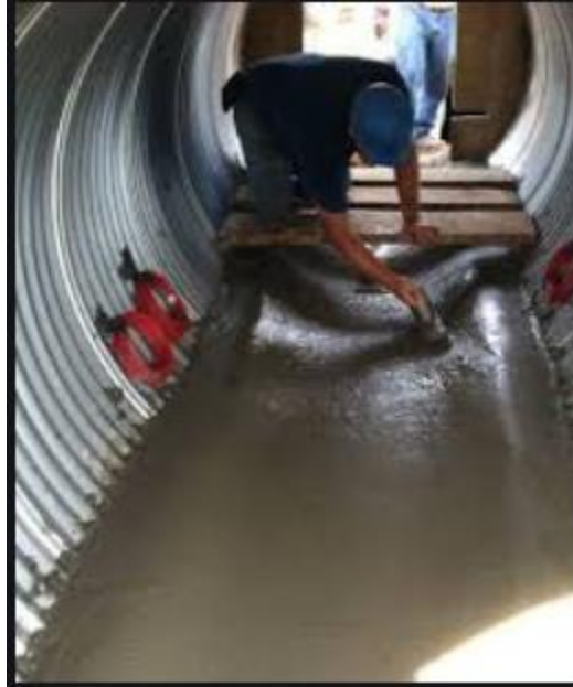
Figure 2-14 Invert Paving (Masada, 2017)
