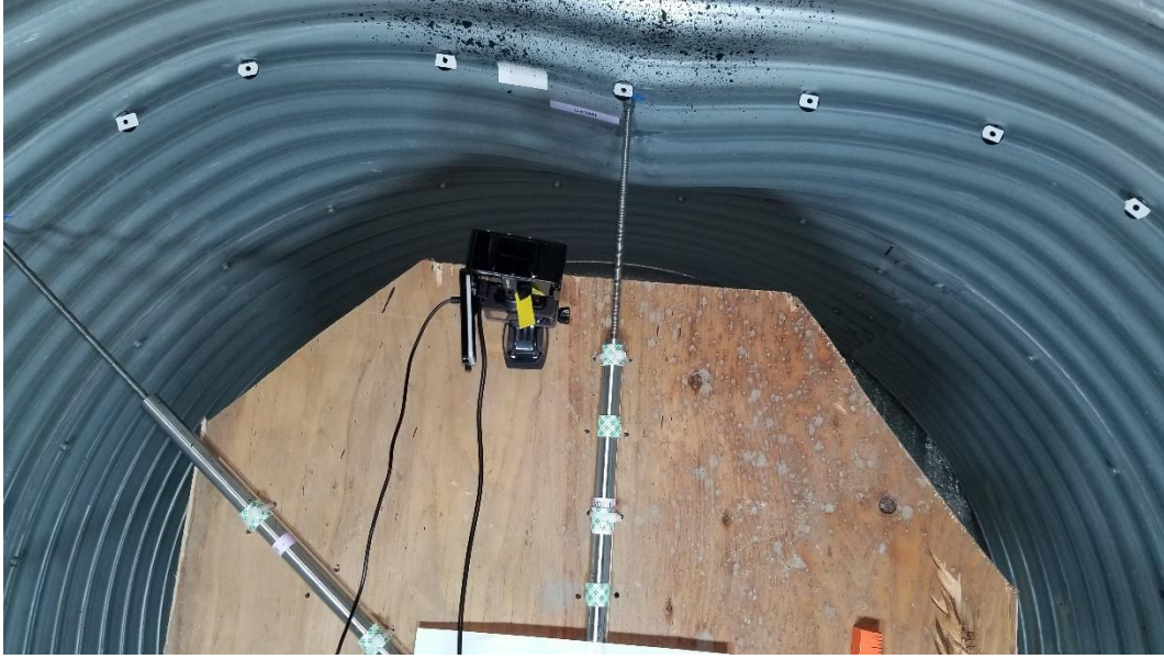
Figure 3-42 Deformation of the CMP after loading (Source: CUIRE LAB)
