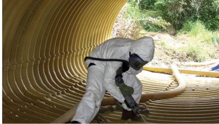
Figure 1-4 Lining the culvert (Mandli, 2017)
