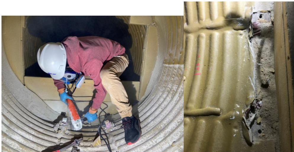
Figure 3-39 End Strip removed (Source: CUIRE LAB)
