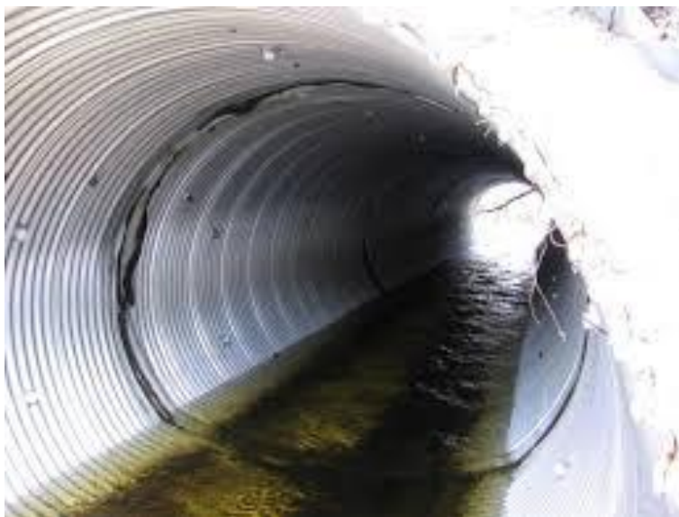
Figure 1-01 Metal culverts in operation (Hartley, 2014)
