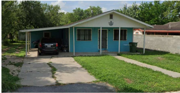
Figure 18. Wooden house in Cameron Park
