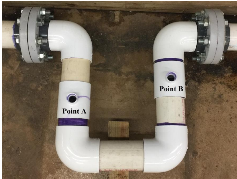
Figure 3-6. Injection points after addition of bends to the pipeline
