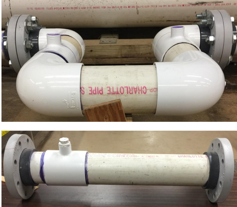
Figure 3-2. Removable sections of the 4.0-inch pipeline
