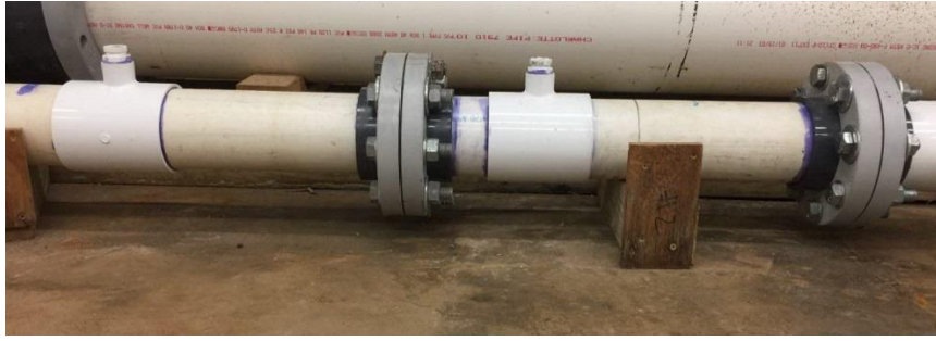
Figure 3-11. Straight section of the pipeline with two injection points
