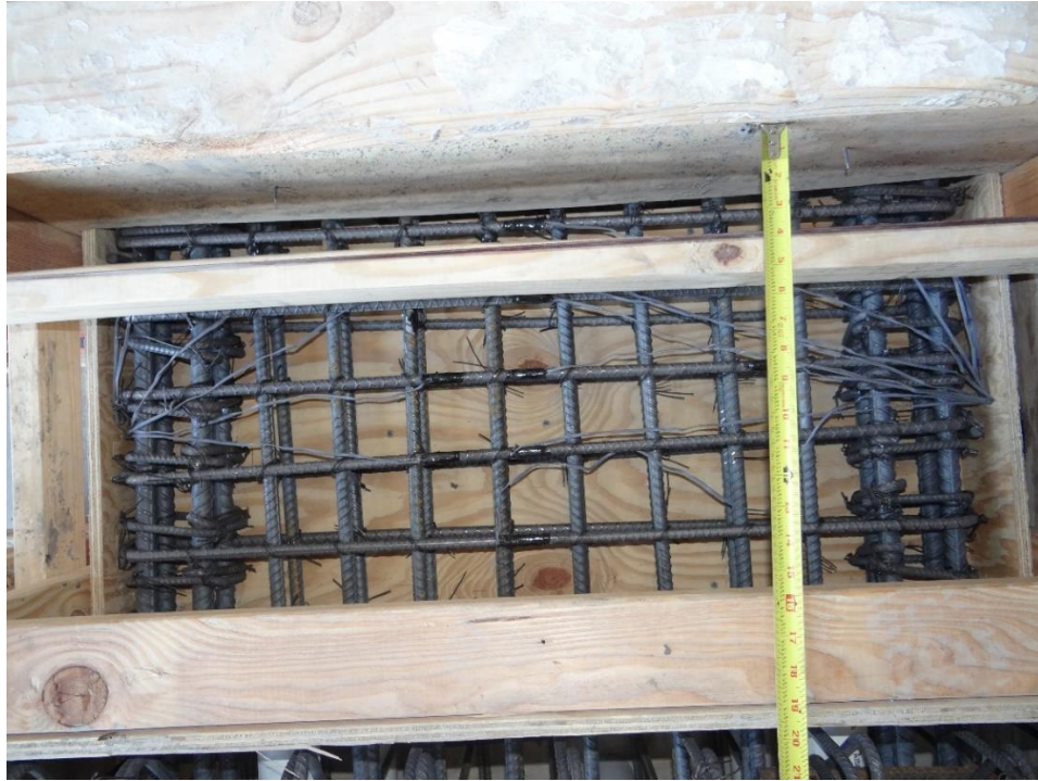
Figure 4-57 Wall height is 20 inches.
