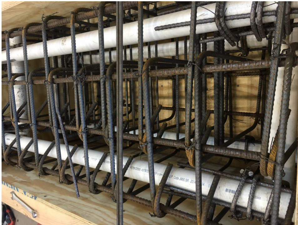
Figure 4-16 The steel reinforcement of loading block
