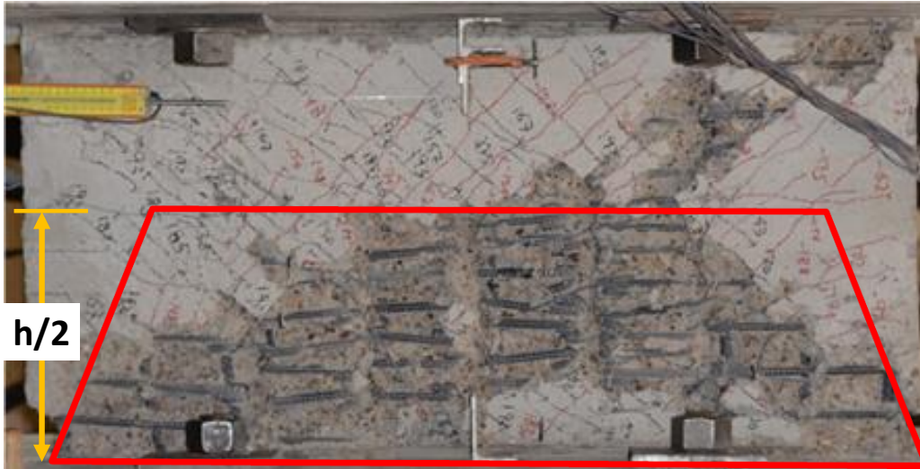
Figure 3-8 Failure mode of specimen SW-HP-0.5-1 at drift ratio 2.5%
