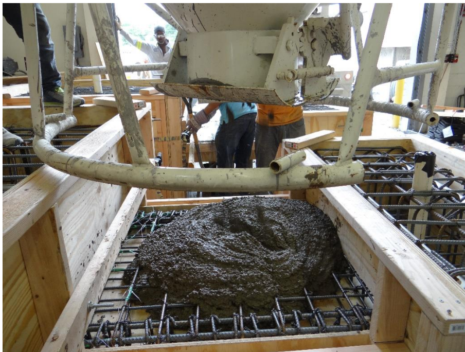
Figure 4-20 Concrete casting of the wall
