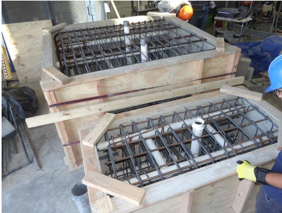
Figure 4-67 Formwork of the completed specimen
