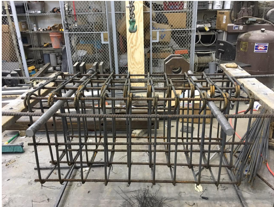
Figure 4-10 The fabricated cage of loading block.
