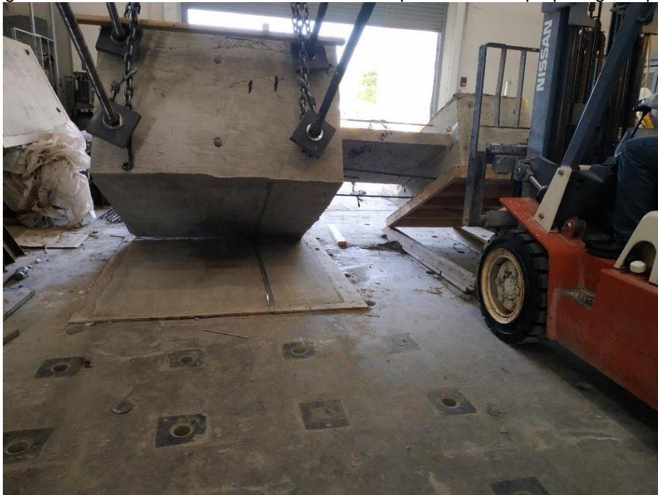
Figure 4-28 Gradually flipping the specimen. The supporting block lifted by crane and the loading block by the forklift, both blocks are connected by \frac{3}{4} -inch diameter rods
