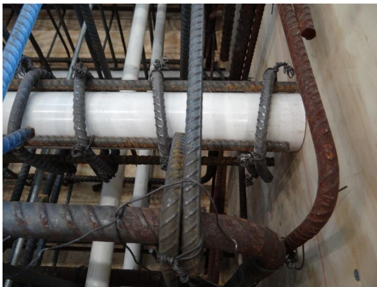
Figure 4-18 Confining hoops around the plastic pipes
