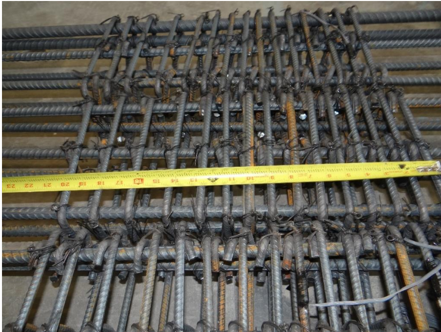
Figure 4-65 Wall height is 20 inches.
