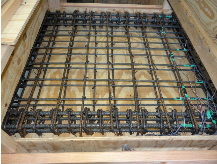
Figure 4-15 The steel reinforcement of wall
