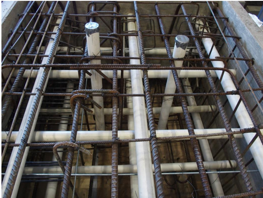
Figure 4-77 Supporting block reinforcement cages and plastic pipes
