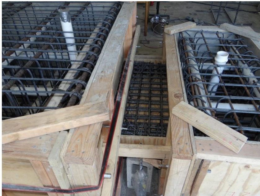
Figure 4-76 Completed formwork and reinforcement fabrication
