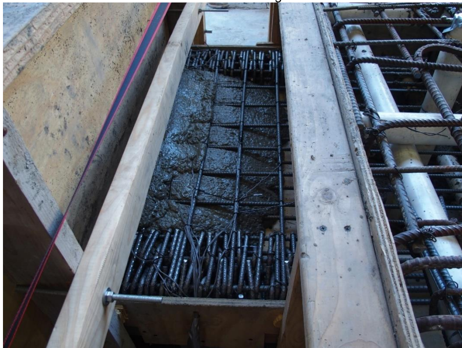
Figure 4-80 Concrete casting
