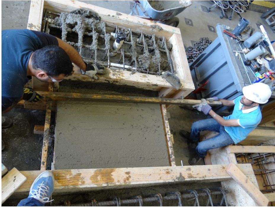
Figure 4-21 Smoothing the wall face after concrete casting
