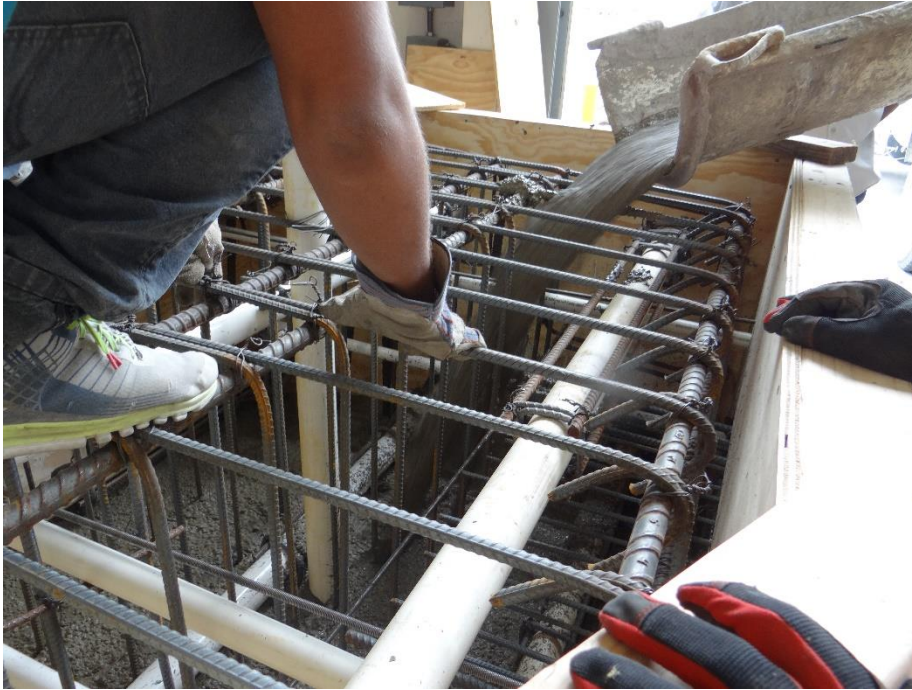
Figure 4-19 Concrete casting of supporting block
