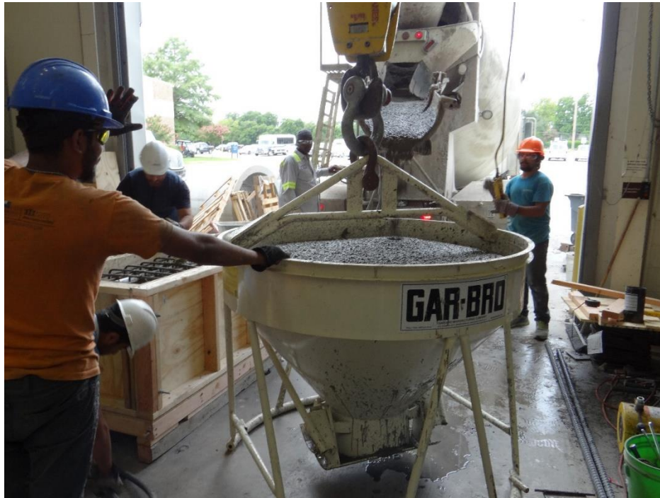
Figure 4-41 Concrete conical bucket to cast concrete
