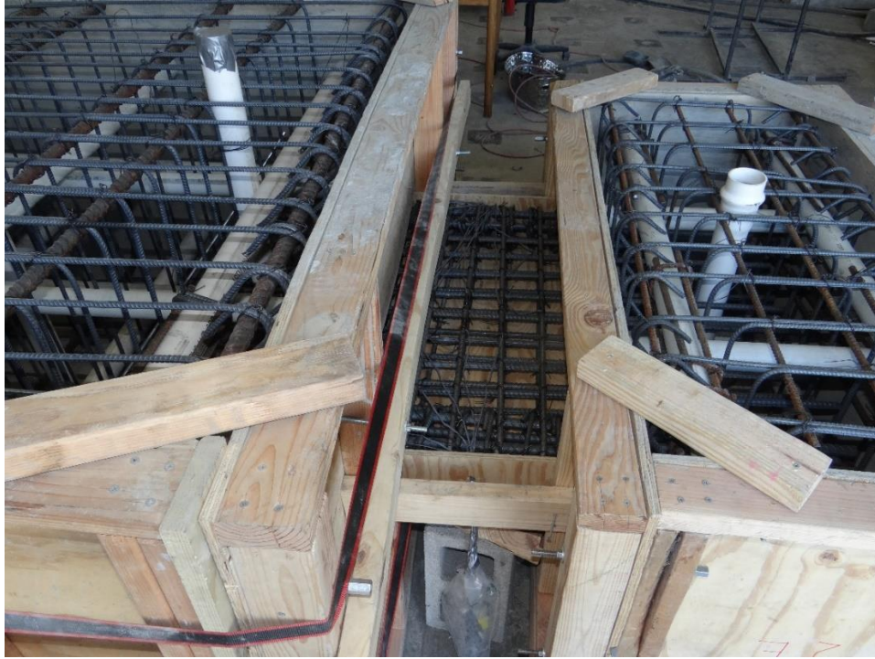
Figure 4-55 Overall steel reinforcement of specimen
