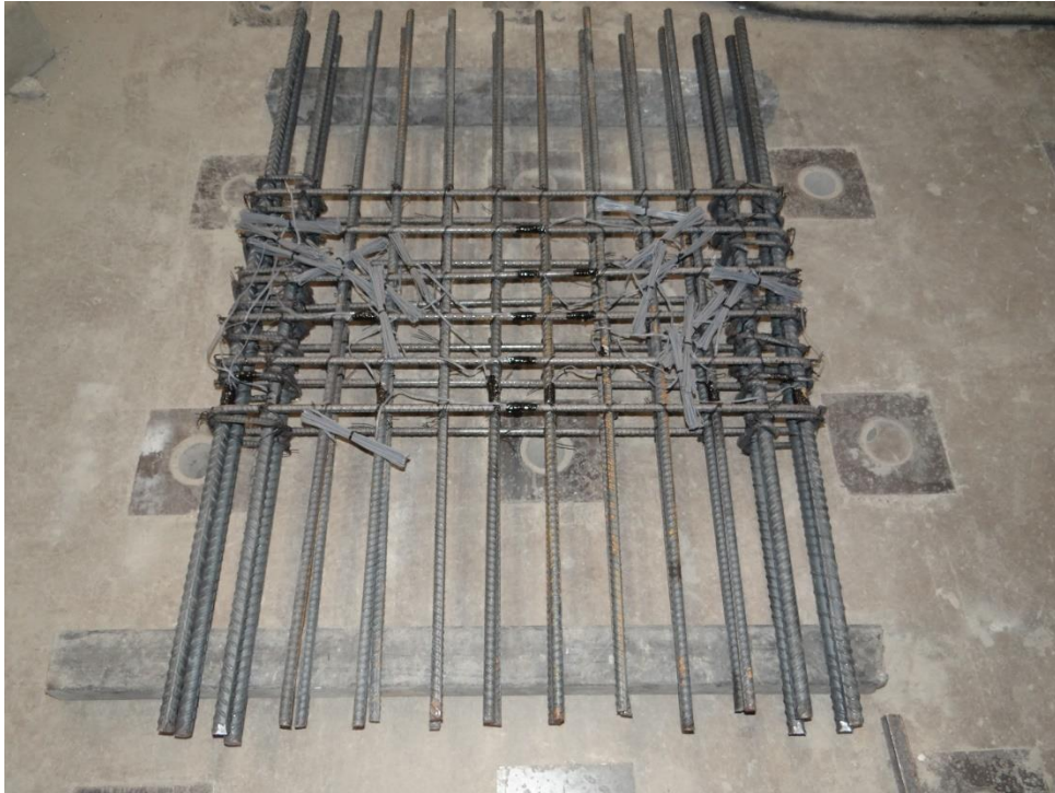
Figure 4-51 Fully prepared cage reinforcement including the attached strain gauges.
