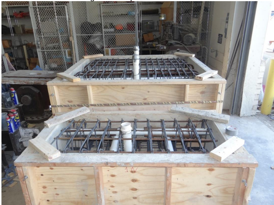
Figure 4-54 Formworks of Supporting and loading blocks
