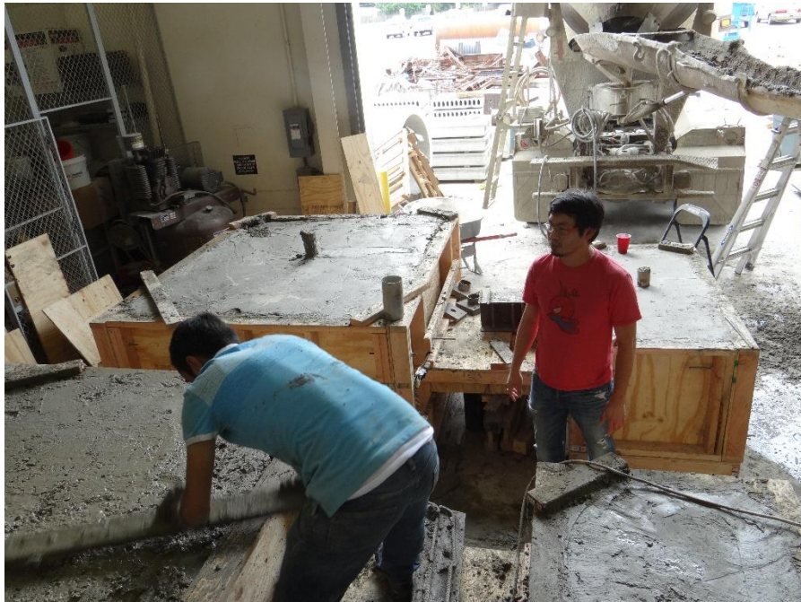
Figure 4-22 Finishing the blocks surfaces.
