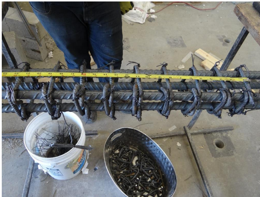
Figure 4-48 preparing the boundary steel cages
