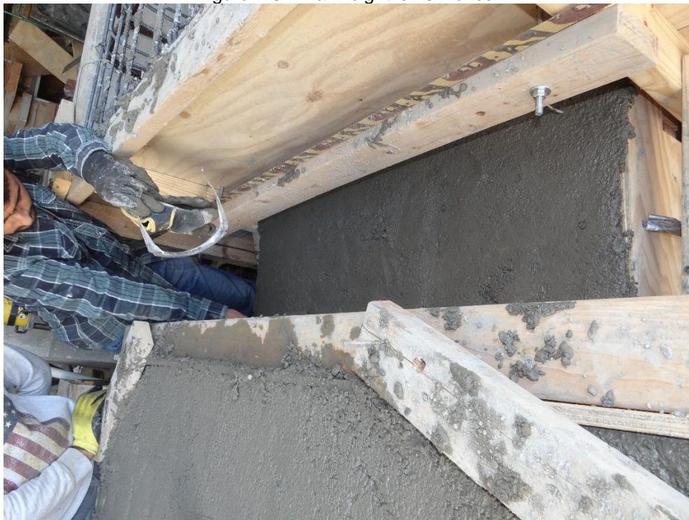
Figure 4-58 Concrete finishing
