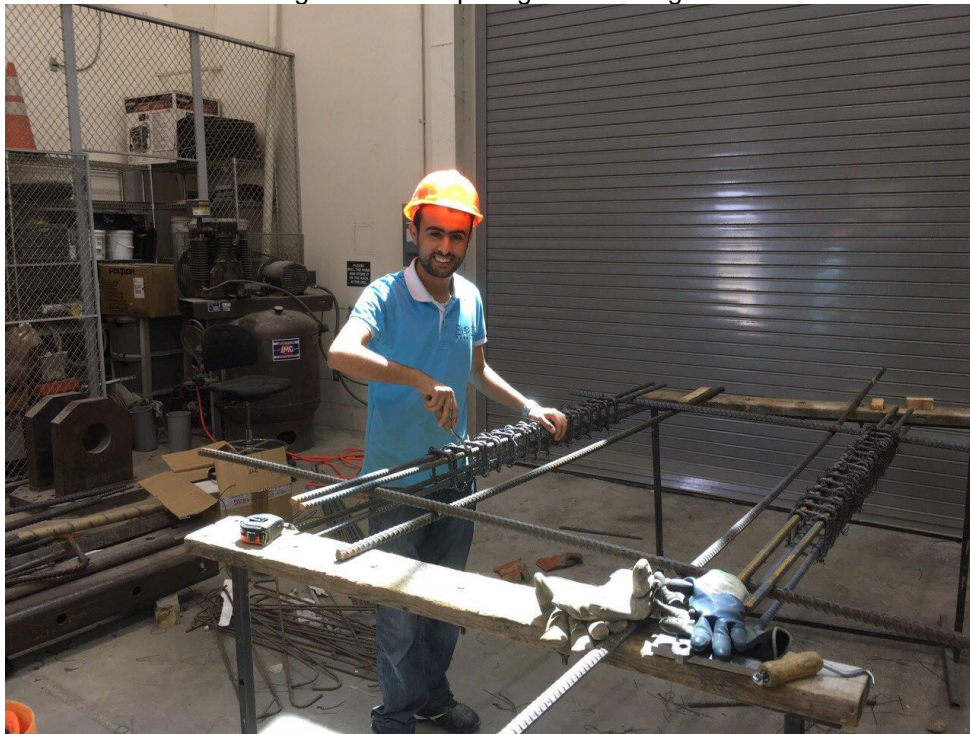
Figure 4-37 Preparing the boundary cages
