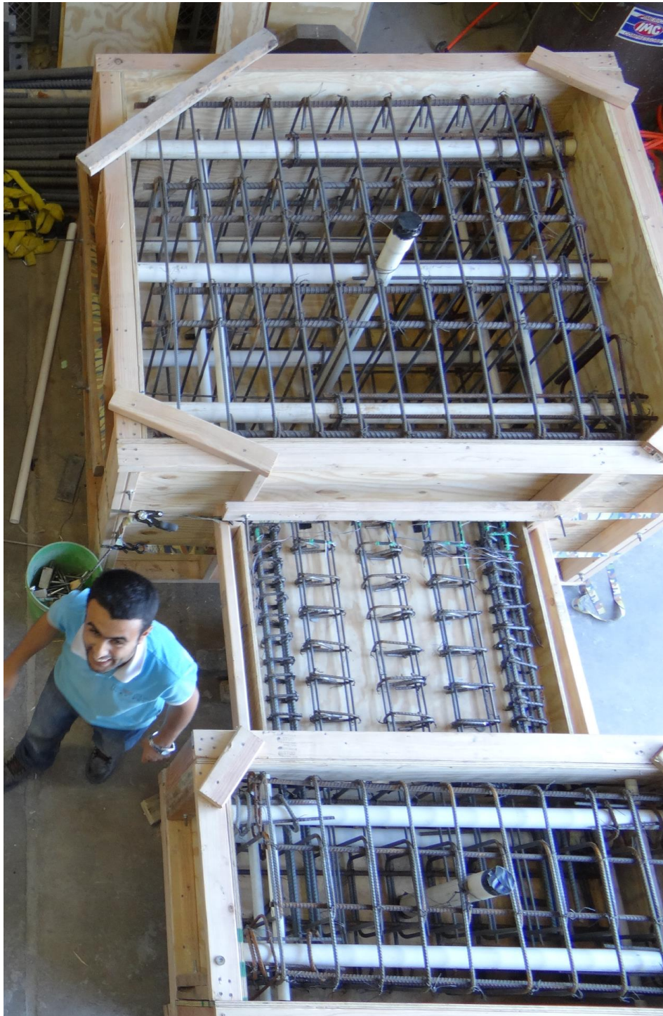
Figure 4-38 Completed construction work, just before casting the concrete
