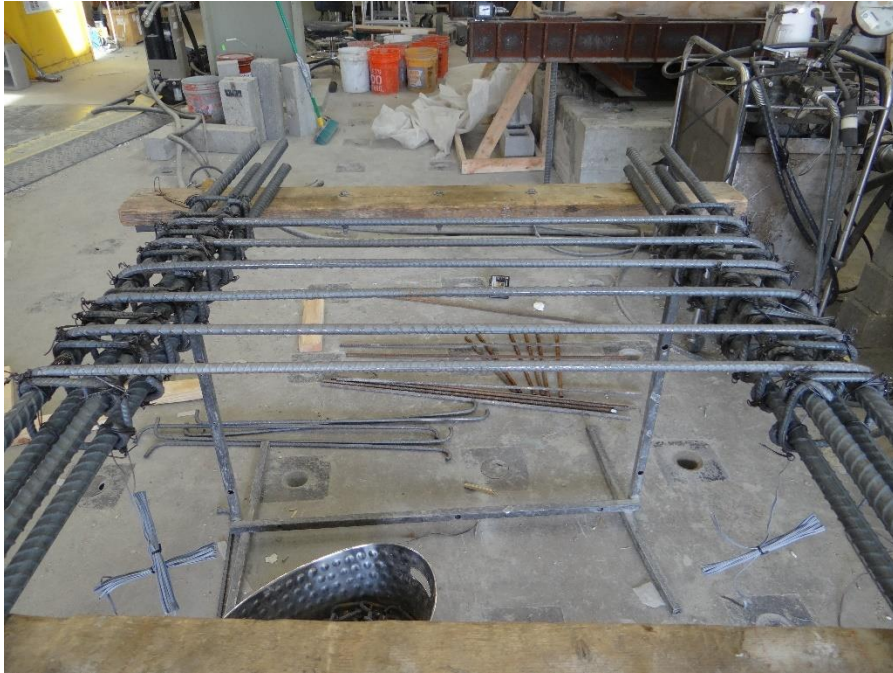
Figure 4-49 Connecting the horizontal steel bars to the boundaries
