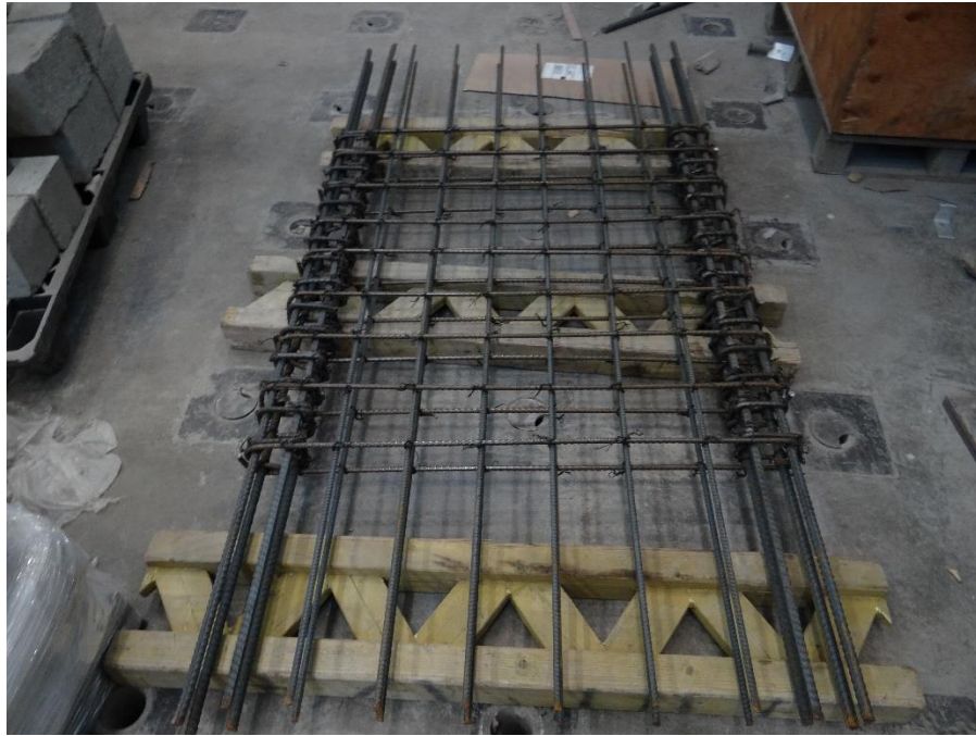
Figure 4-12 The fabricated wall reinforcement
