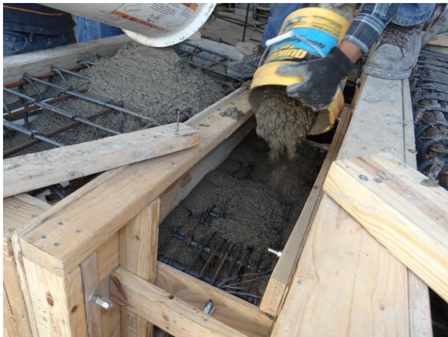
Figure 4-70 Concrete casting.
