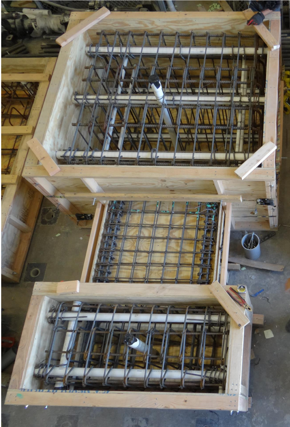
Figure 4-14 Complete specimen components before concrete casting.
