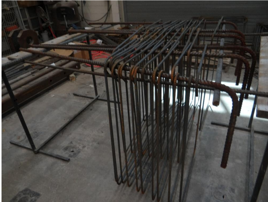
Figure 4-8 Preparing the steel cage of supporting block
