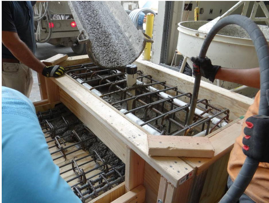
Figure 4-39 Concrete casting of the loading block up to mid height.
