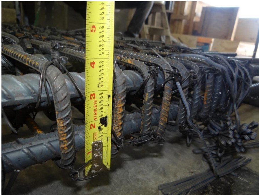
Figure 4-66 Wall thickness is 4 inches.
