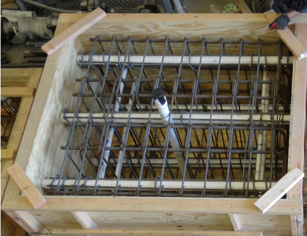
Figure 4-17 The steel reinforcement of supporting block
