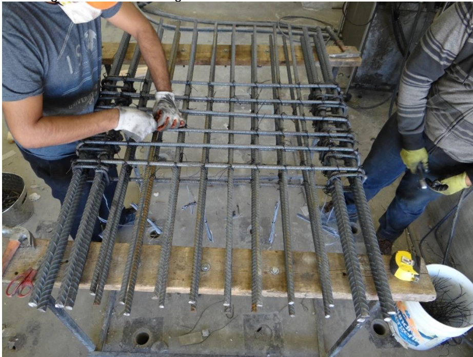
Figure 4-50 Fabricating the wall cage
