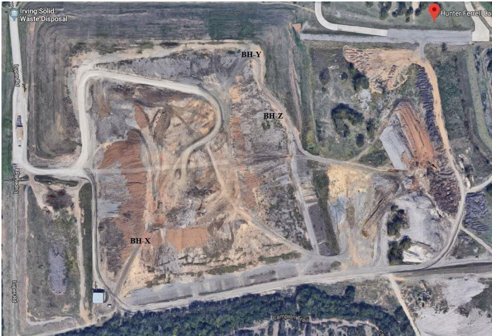
Figure 3-4 Positions of the boreholes in City of Irving landfill
