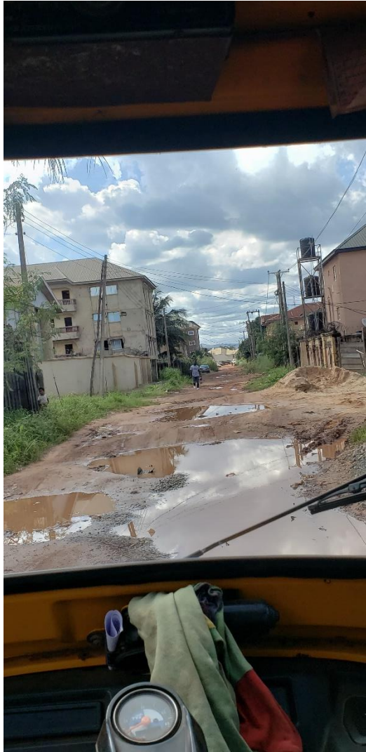
Figure 12. Lack of drainage and unpaved roads in Iji-Nike Community
