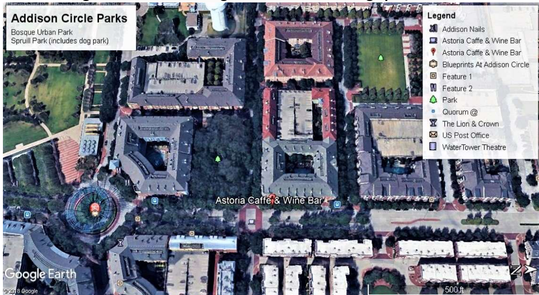
Aerial image of New Urban Addison Circle, showing Bosque Park central to the photo.
