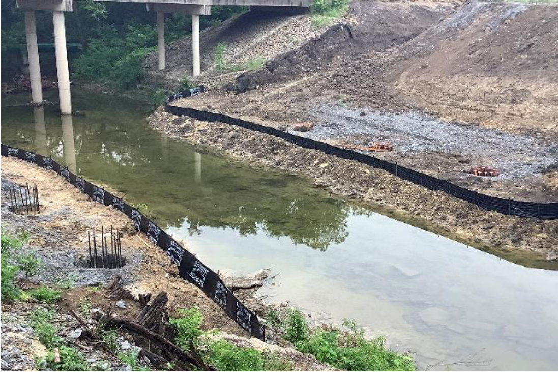
Figure 4 Silt fence installed in Wilson Creek
