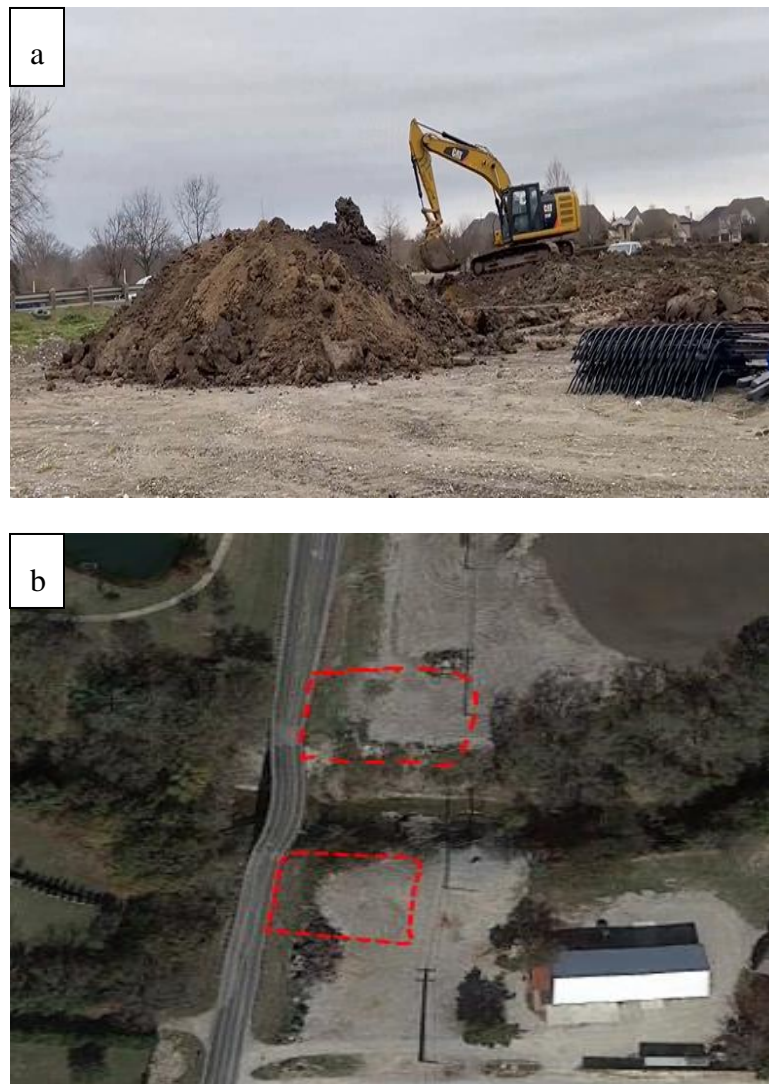
Figure 22 Grading work (a)Boundary for grading work, (b) Site grading works
