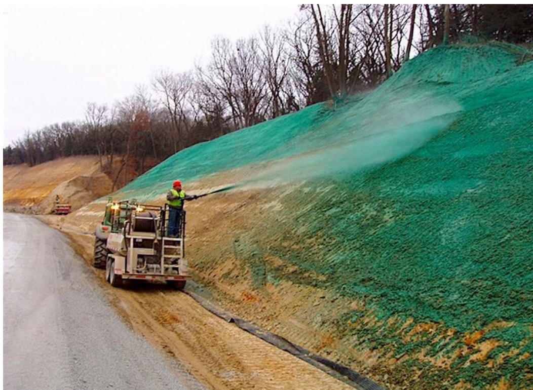
Figure 13 Hydroseeding (CALTRANS 2017)
