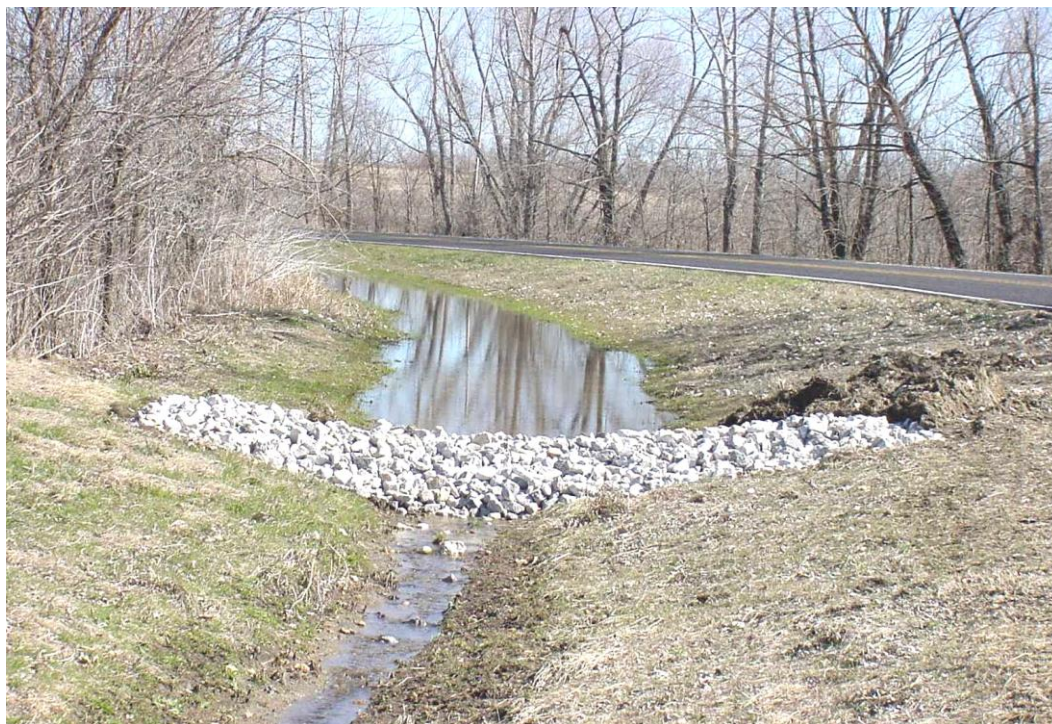
Figure 11 Rock filter dam (TxDOT 1993)
