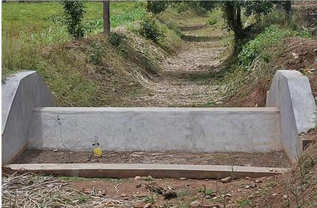
Figure 12 Check dam (Da-Chuan et al., 2008)
