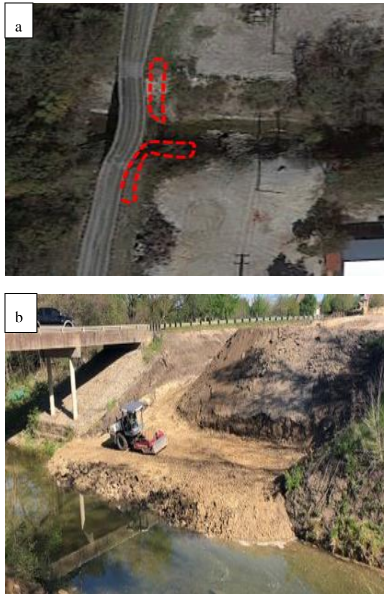
Figure 23 Formation of access road (a) boundary, (b) site works
