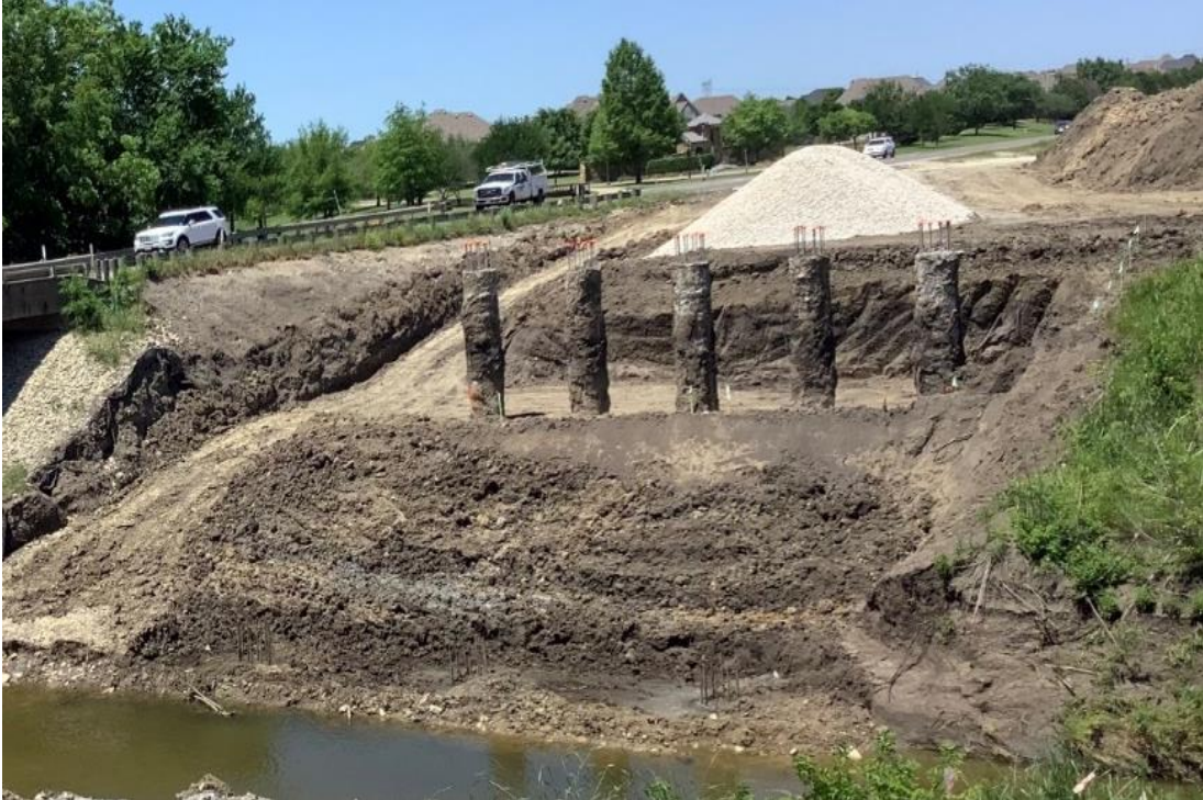
Figure 3 Bridge construction at Wilson Creek
