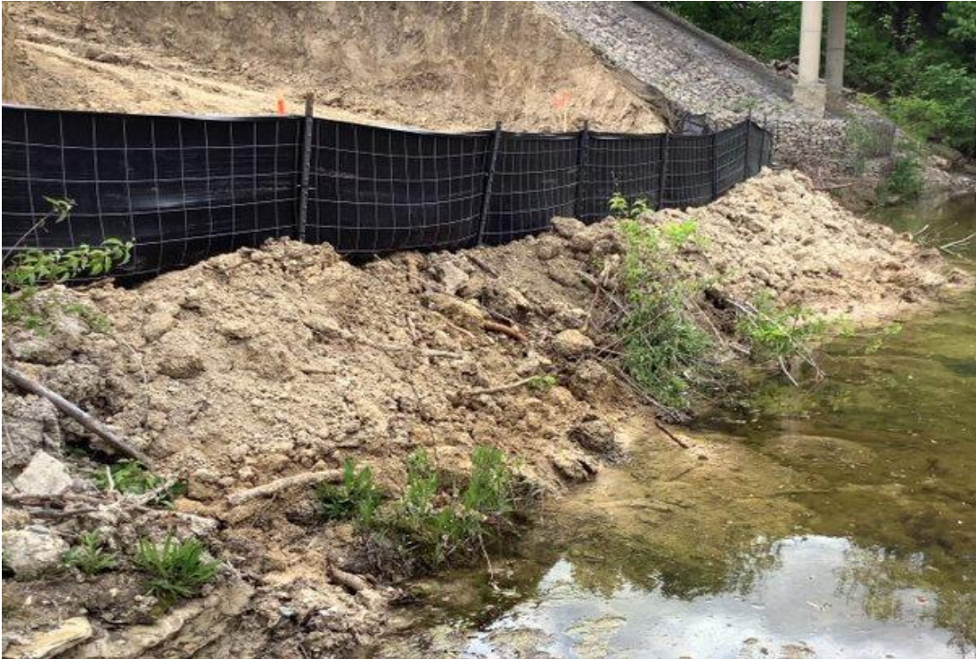
Figure 6 Silt fence installed at edge of construction works
